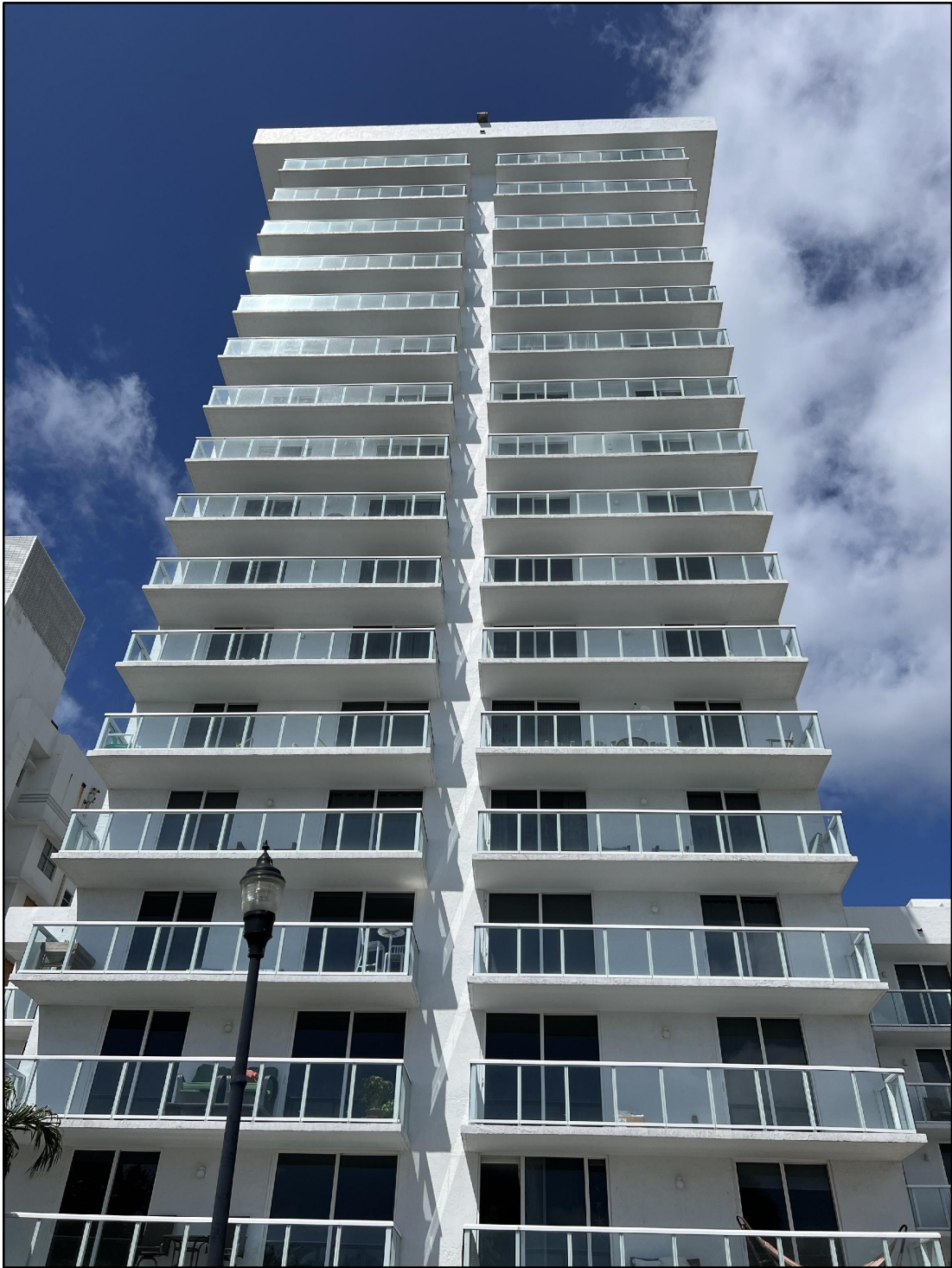
2457 COLLINS AVE. REAR OF BUILDING EAST FACADE 03/28/2023
