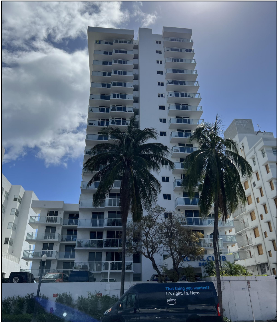
2457 COLLINS AVE. FRONT OF BUILDING WEST FACADE 03/28/2023
