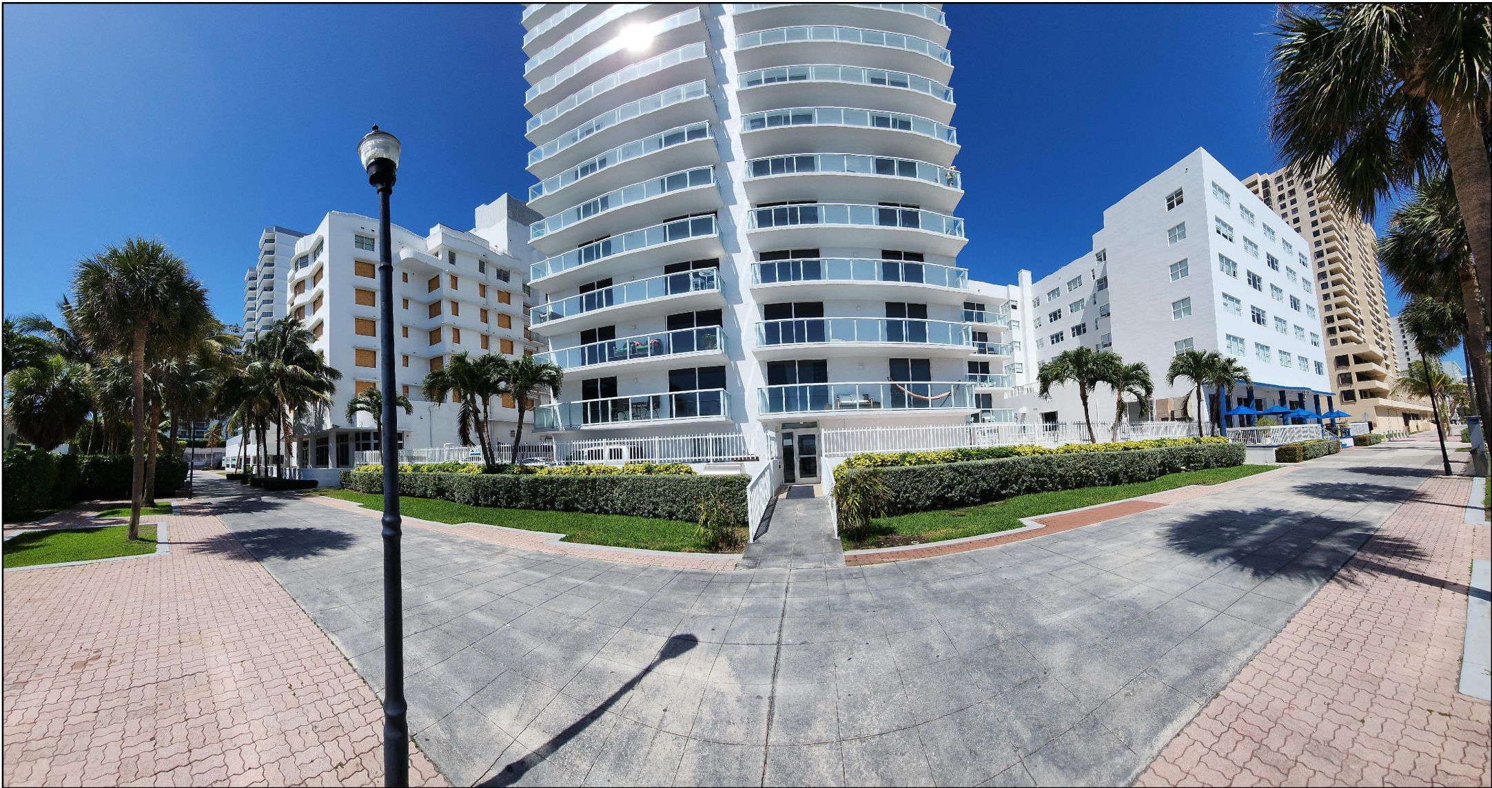
2457 COLLINS AVE. REAR OF BUILDING EAST FACADE 03/28/2023
