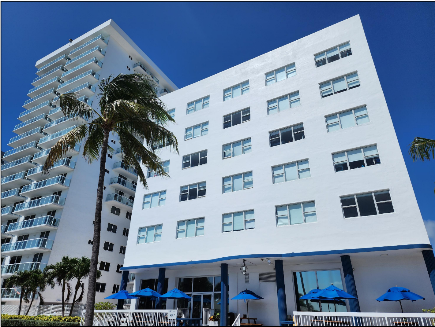
2457 COLLINS AVE. REAR OF BUILDING EAST FACADE 03/28/2023
