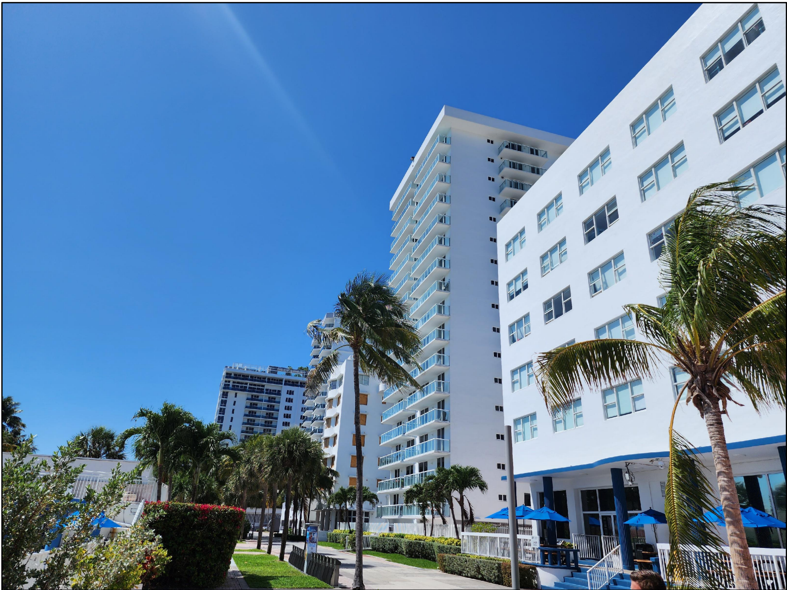
2457 COLLINS AVE. REAR OF BUILDING EAST FACADE 03/28/2023
