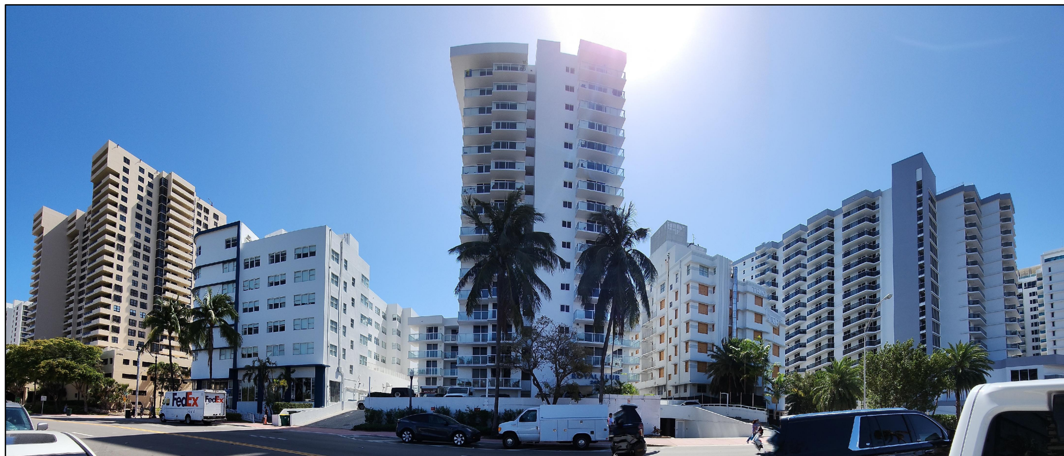
2457 COLLINS AVE. FRONT OF BUILDING WEST FACADE 03/28/2023
