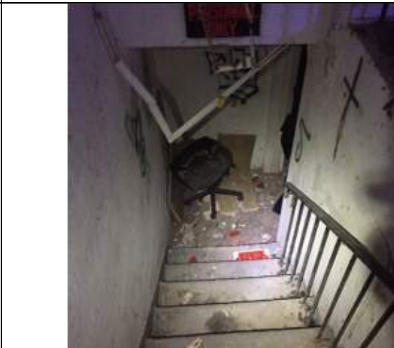
Level 1 – Central Stair down to basement
