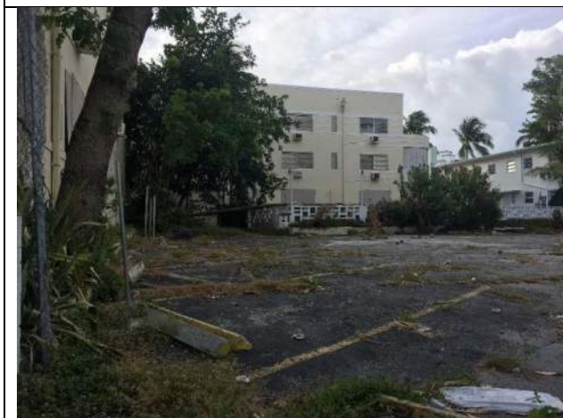
South & West Elevations And Washington Ave. parking lot
