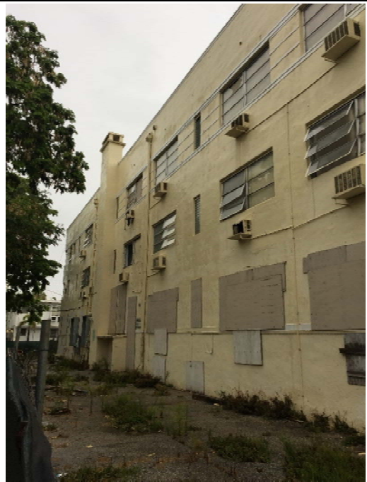
North Elevation from west
