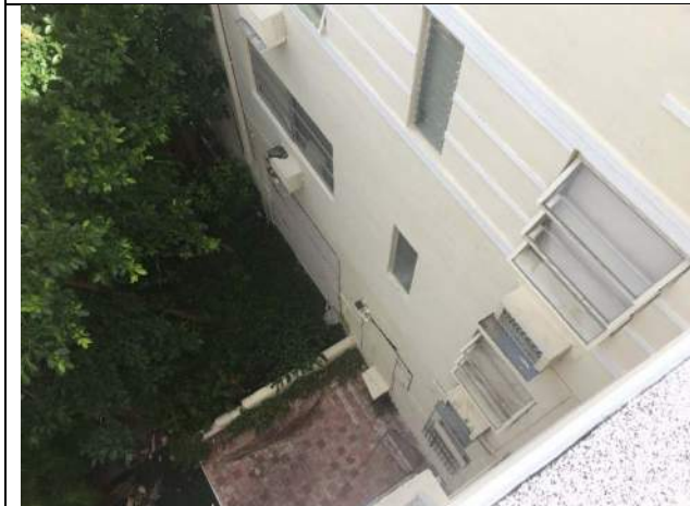
View from roof to west entrance and south facade
