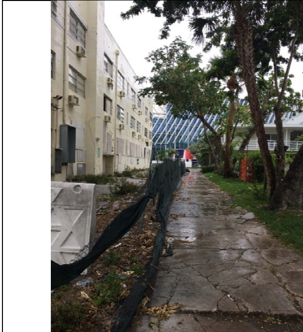
North Elevation and side yard, from east
