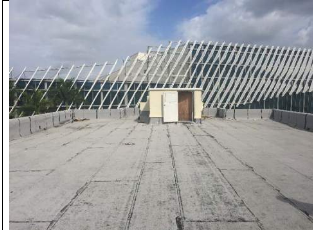
North wing roof – view west
