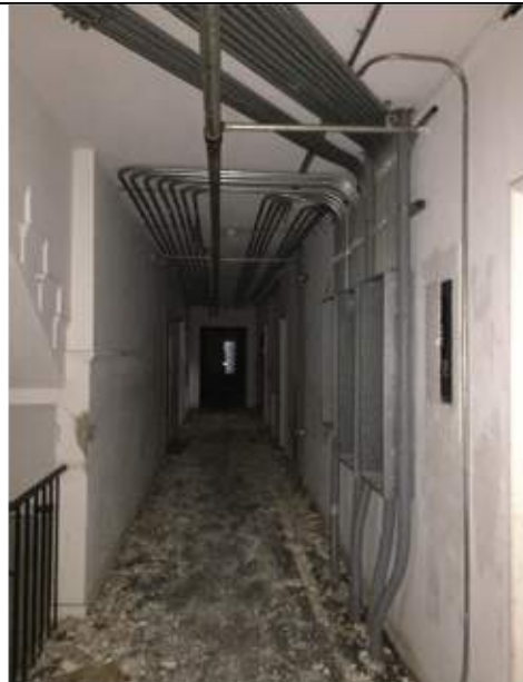
Corridor – exposed electrical conduit
