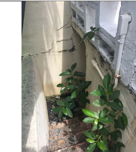
Stair down to Pool Equipment Room
