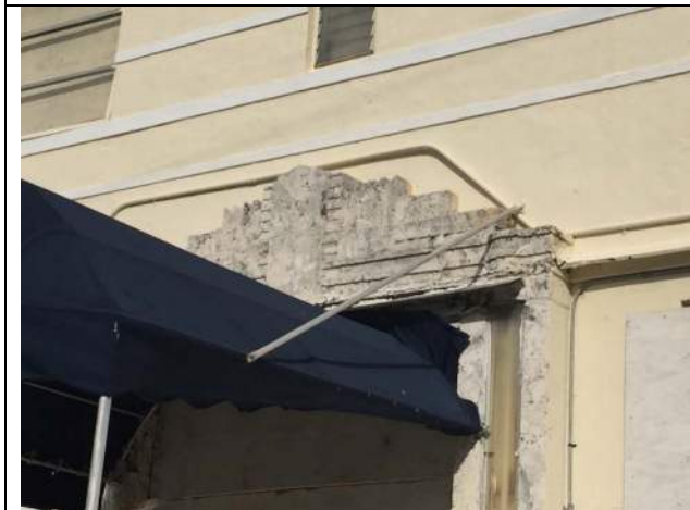
Main Entrance Stone & Light Fixture Detail
