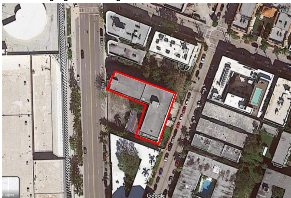
Figure 1. Aerial view of building
