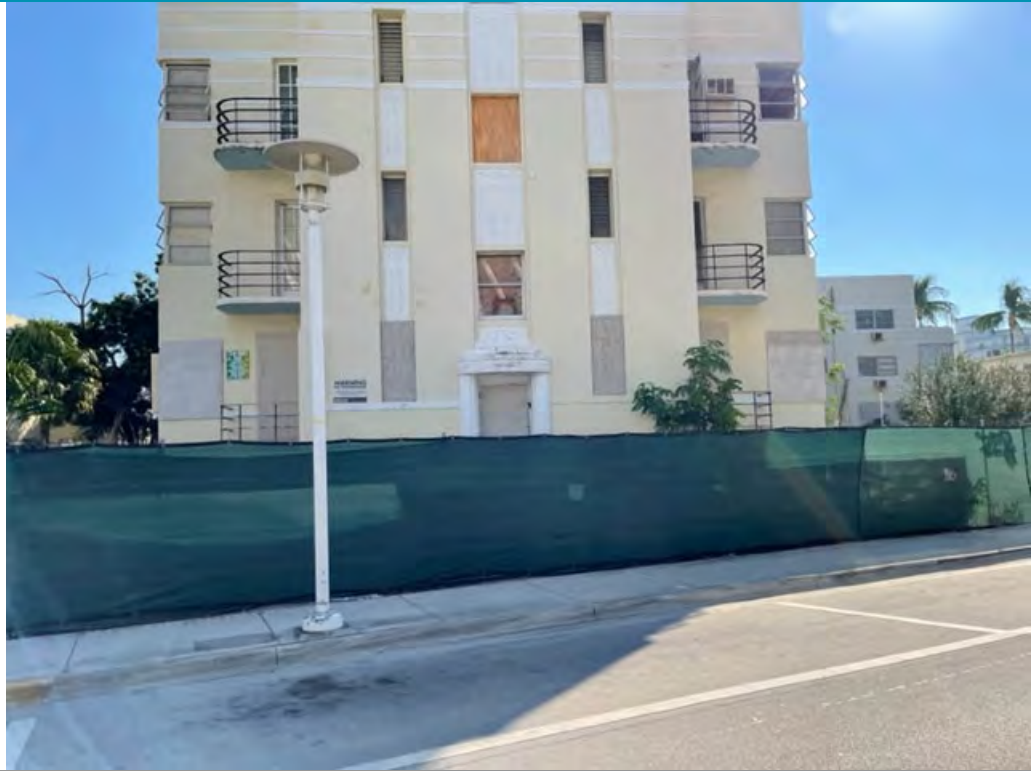
VIEW OF SUBJECT SITE
