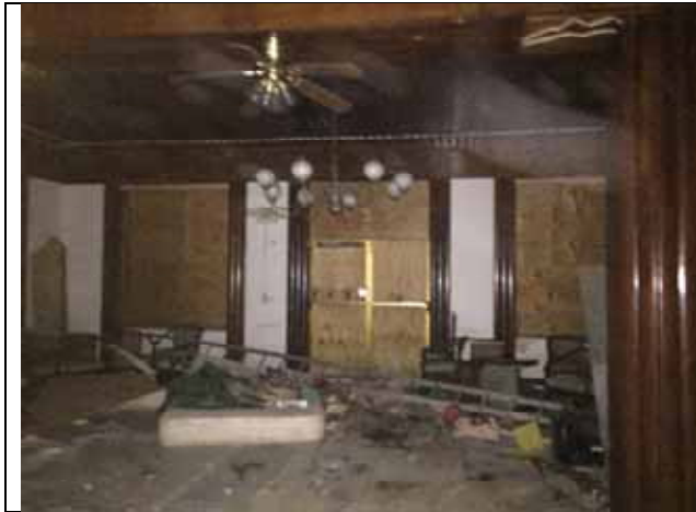
Lobby – view to east
