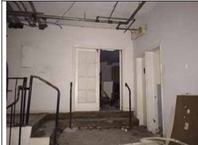
Lobby – steps up to north wing, RR on right
