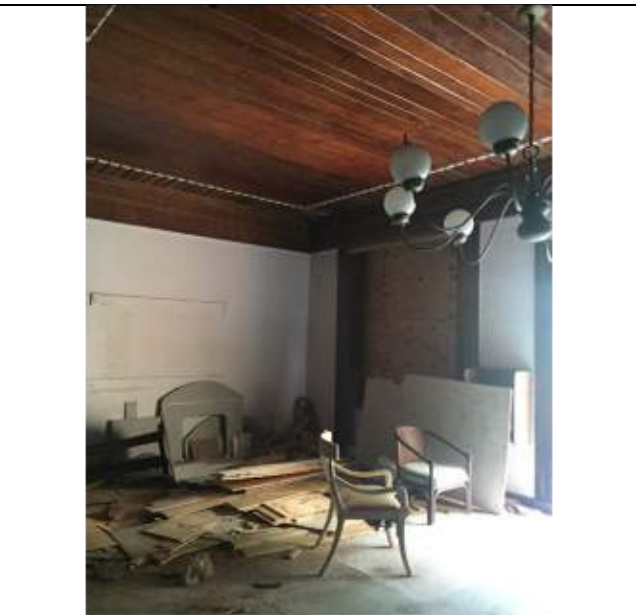
Lobby – view to SW
