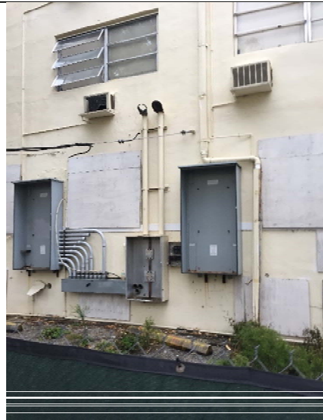
North Elevation Former electrical service location
