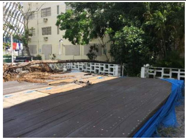
Pool – view from southeast
