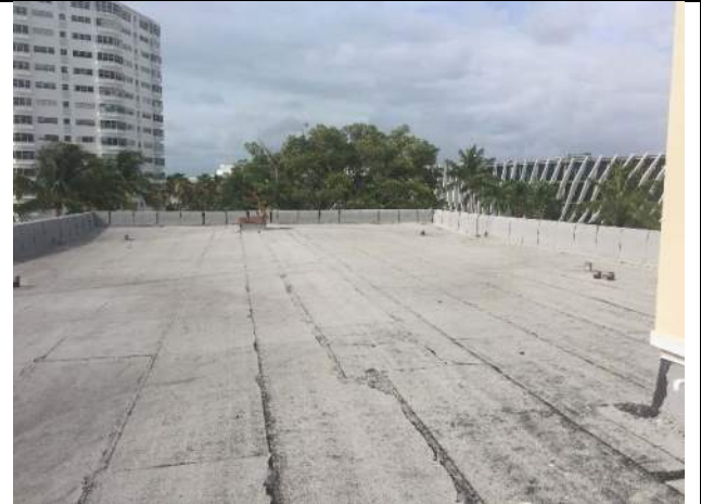
South wing roof – view south
