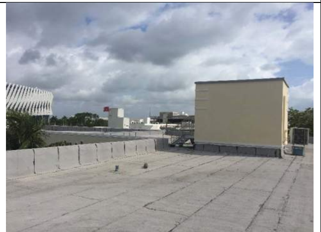
South wing roof – view north. Elevator Machine Room.
