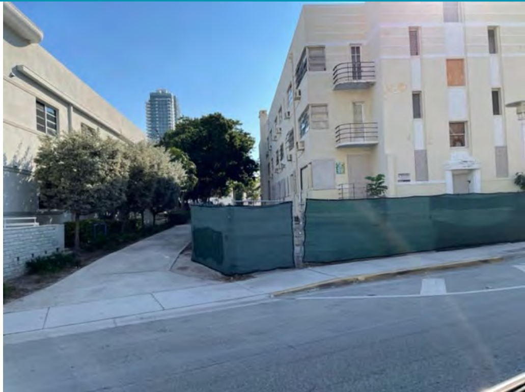
VIEW OF SUBJECT SITE
