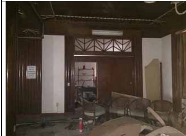
Lobby – View to north lounge
