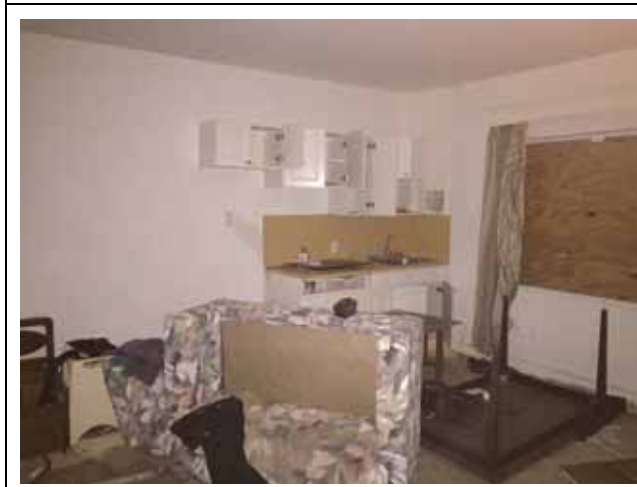
Level 1 north wing – communal room
