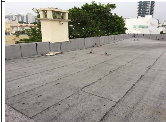
North wing roof – view east. Former Kitchen Exhaust.
