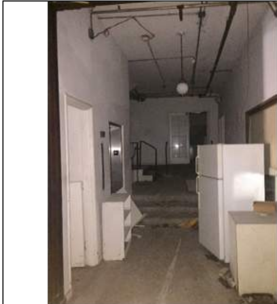
Lobby – passage to elevator & north wing
