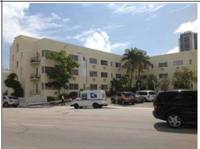
Washington Avenue – Southwest Elevation
