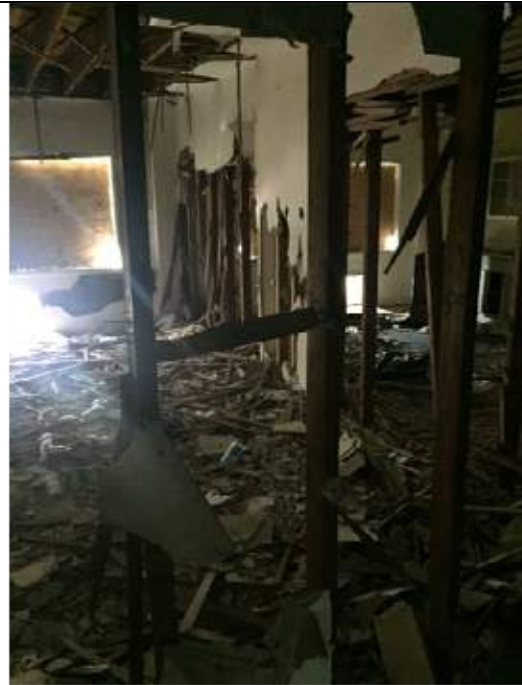
Apartment – corridor furring & finish removed
