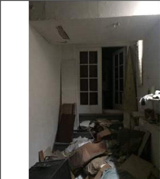
Lobby lounge – steps up to communal room
