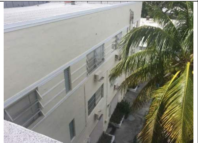
View from roof to pool deck and west facade .
