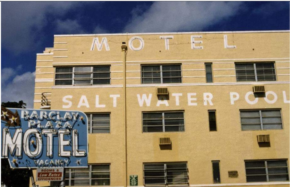
View from south on Washington Avenue
