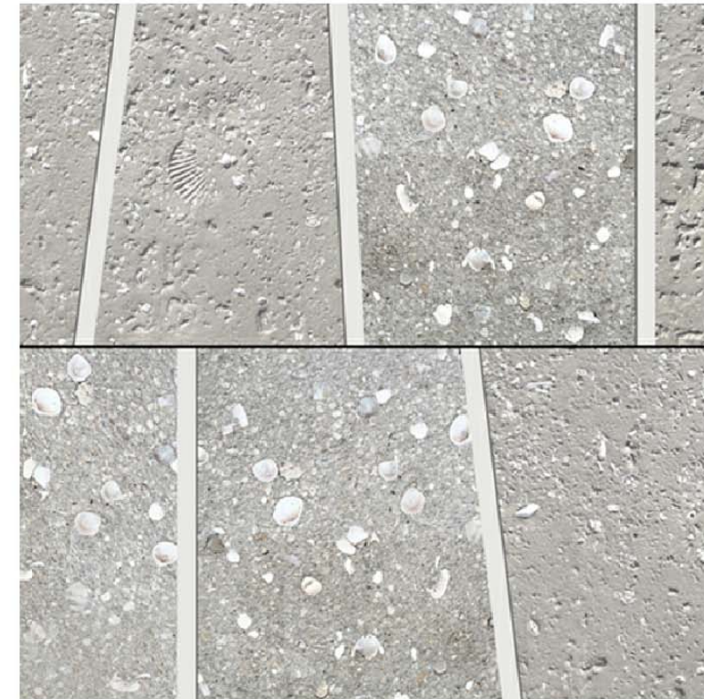
PRECAST PAVERS at the drop-off
