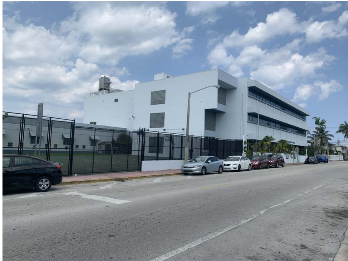
(1) VIEW FACING NORTHEAST ON 77th STREET
