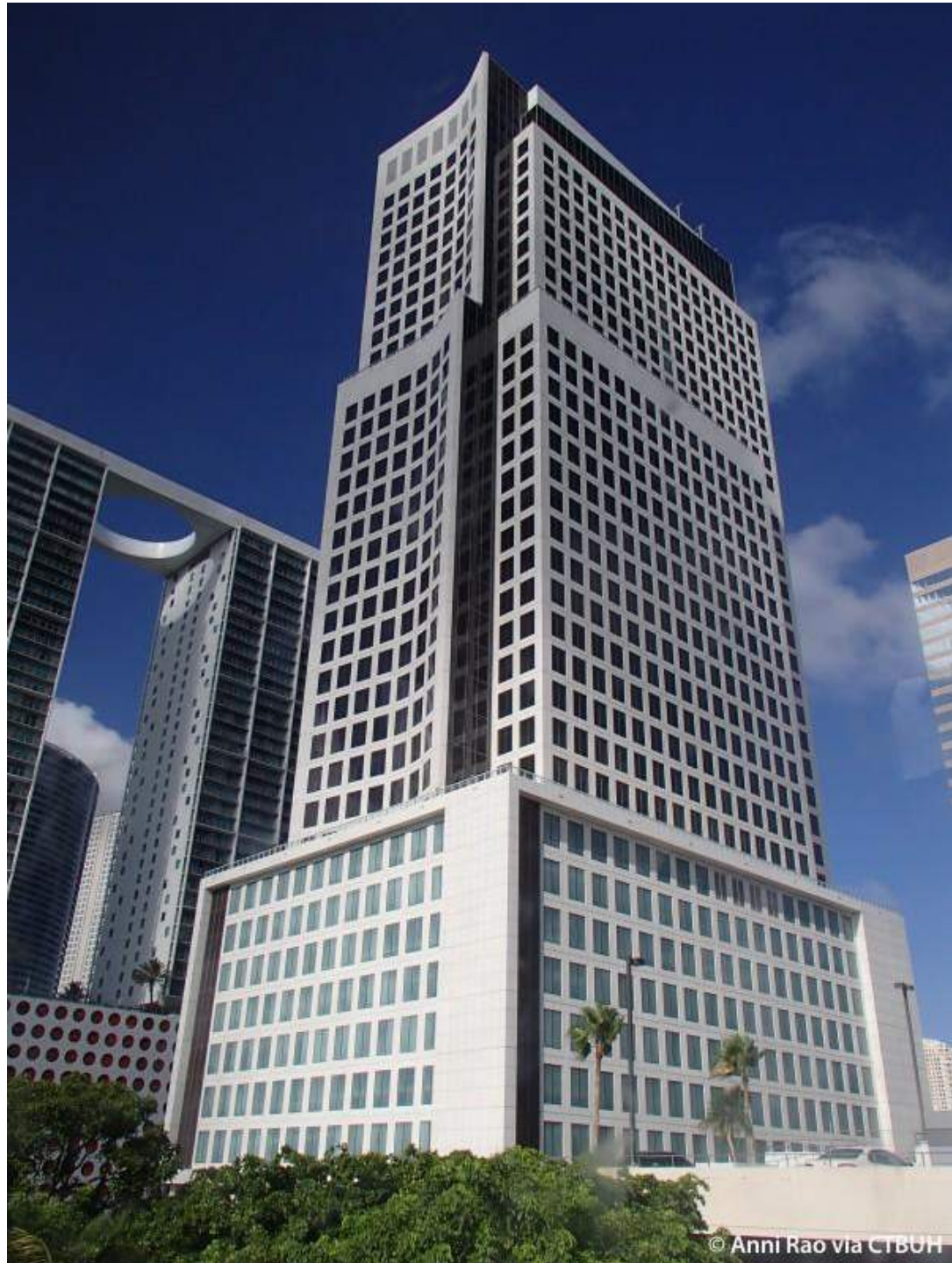
CLASS A OFFICE TOWER: 600 BRICKELL AVENUE TENANT: SITEL FLOOR TO FLOOR HEIGHT: 13'-6" FINISHED CEILING HEIGHT: 10'-0"
