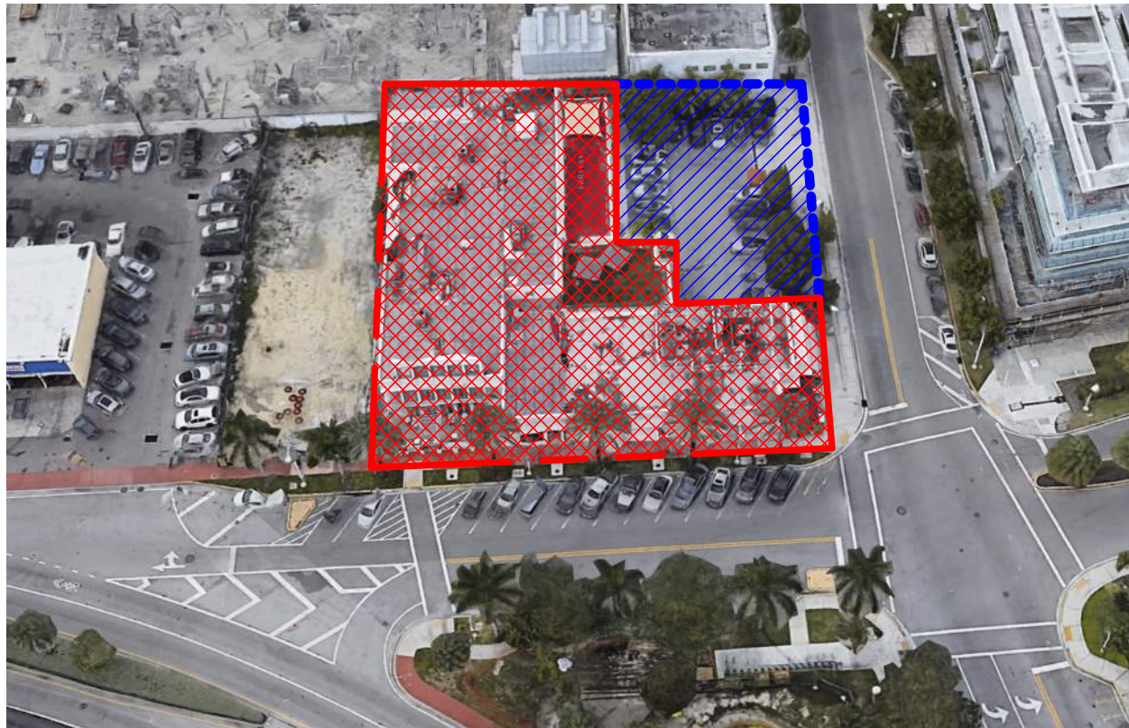
1. AERIAL OF PROPERTY FROM ALTON ROAD
