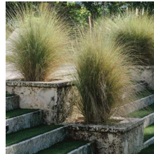
KEYSTONE CLAD RETAINING WALL/PLANTER
