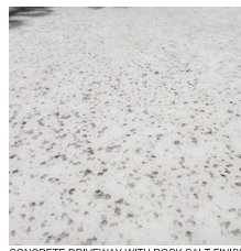
CONCRETE DRIVEWAY WITH ROCK SALT FINISH
