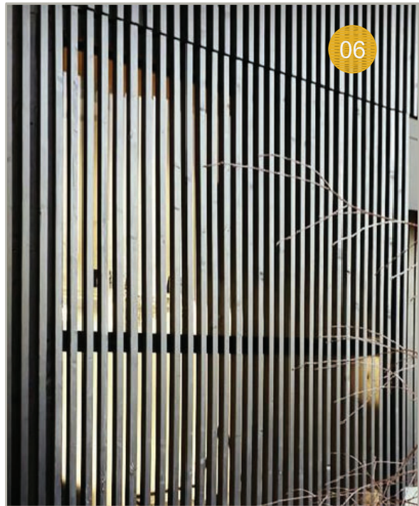
BLACK ALUMINUM BATTENS SCREEN @ FIRST FLOOR
