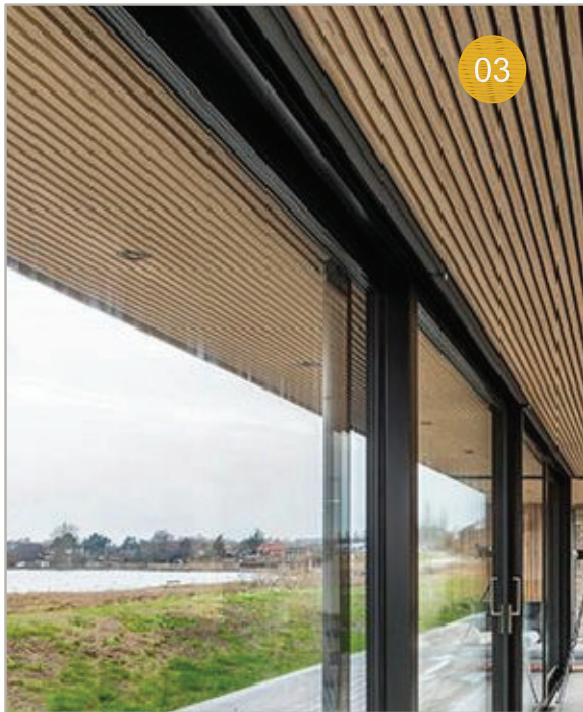
WOOD PLANK CEILING SYSTEM @ BALCONIES & OVERHANGS
