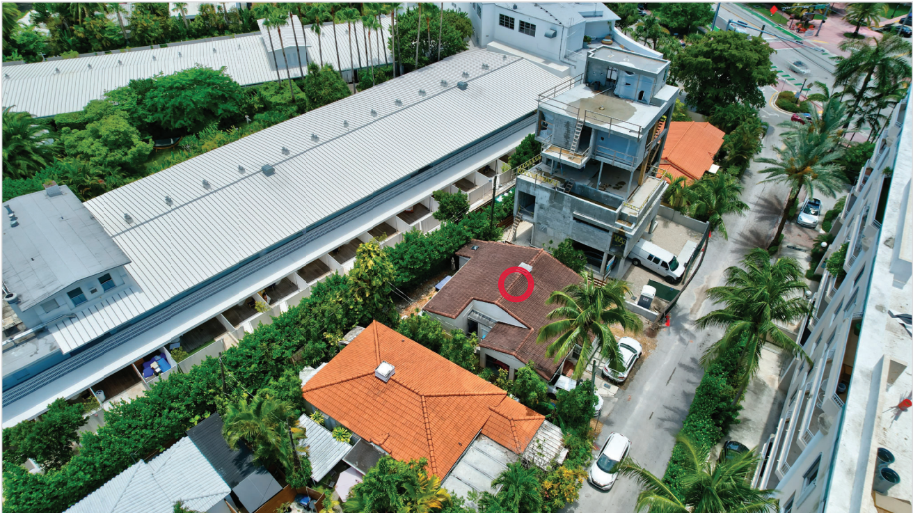
AERIAL SITE VIEW 01
