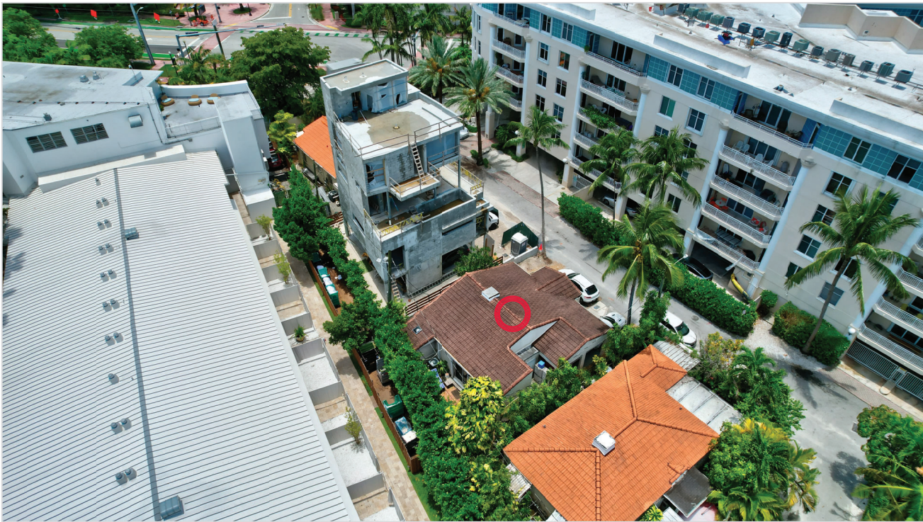
AERIAL SITE VIEW 02
