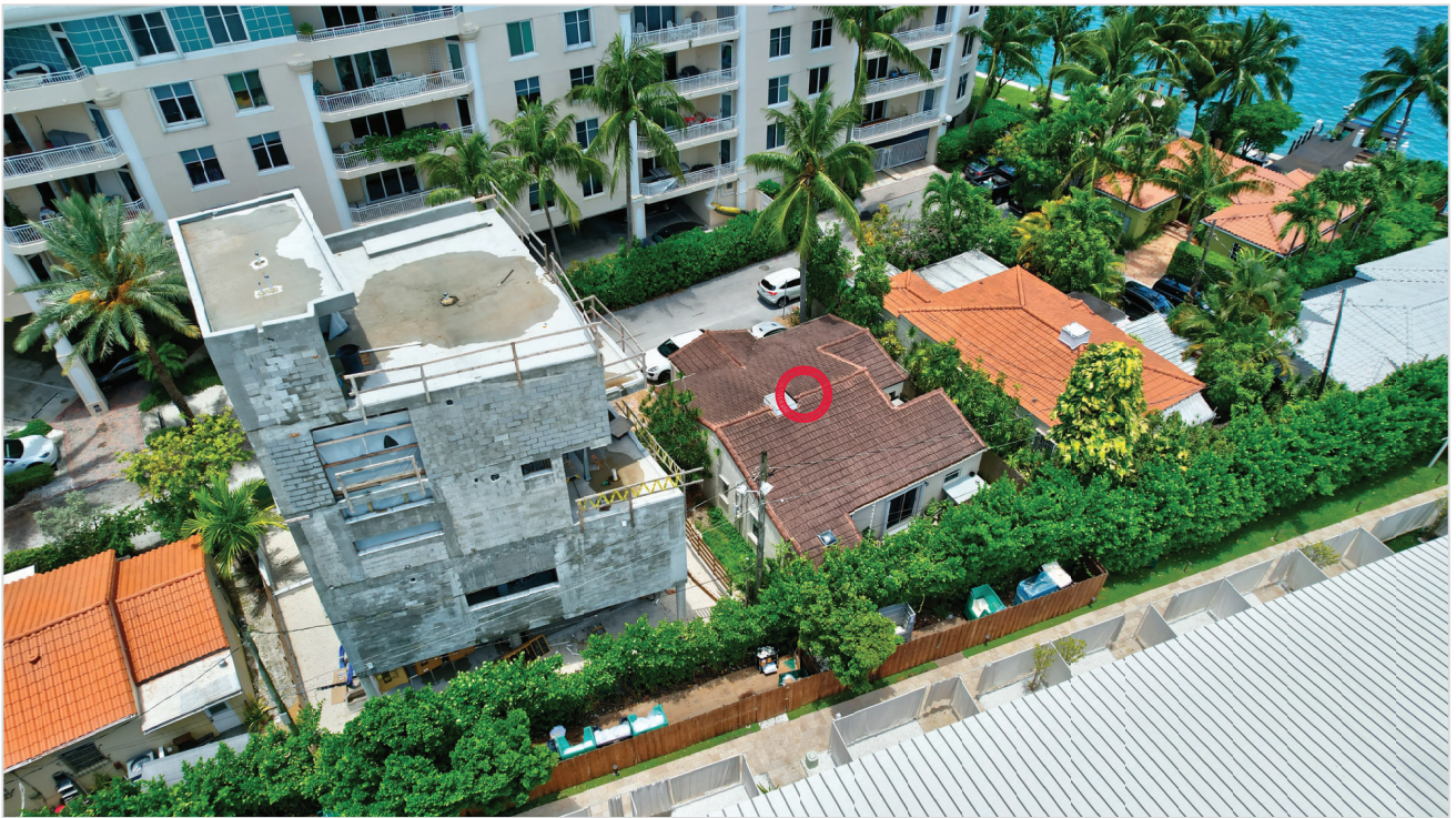
AERIAL SITE VIEW 03
