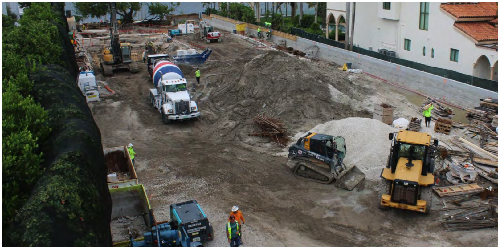
CONSTRUCTION PHOTO | FACING SOUTHEAST | OCT 2022
