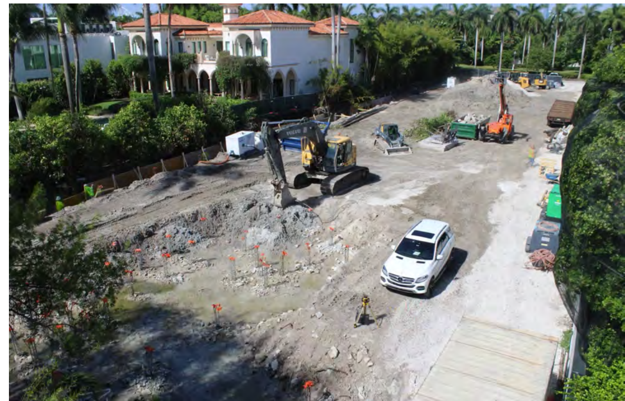
CONSTRUCTION PHOTO | FACING SOUTHWEST | AUGUST 2022
