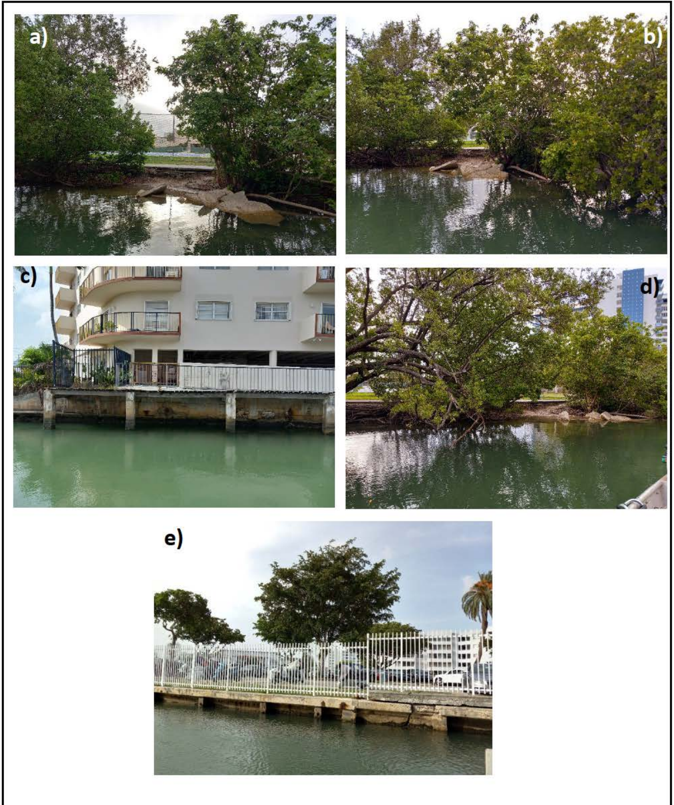
Figure D.7: Shoreline types along PVC varies from sediment shoreline with dense mangrove canopy, exposed sediments showing signs of erosion, sediment shoreline reinforced with human-made walls, and a retaining wall extending to an undetermined depth
