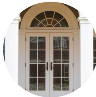
IMPACT RESISTANT DOORS & WINDOWS W/ CLEAR GLASS. DESIGN BASIS: CGI SENTINEL SERIES WINDOWS AND DOORS IN EXISTING BUILDING TO MATCH HISTORIC LAYOUT AND DIMENSIONS OF FRAMES, MUNTINS AND LITES. TYP.
