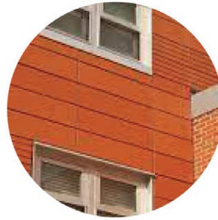
TERRACOTTA CLADDING DESIGN BASIS: NBK TERRACOTTA - TERRART ECO22 10" X 60" HORIZONTAL PANELS COLOR: 1.02-0 (GROUP 2)
