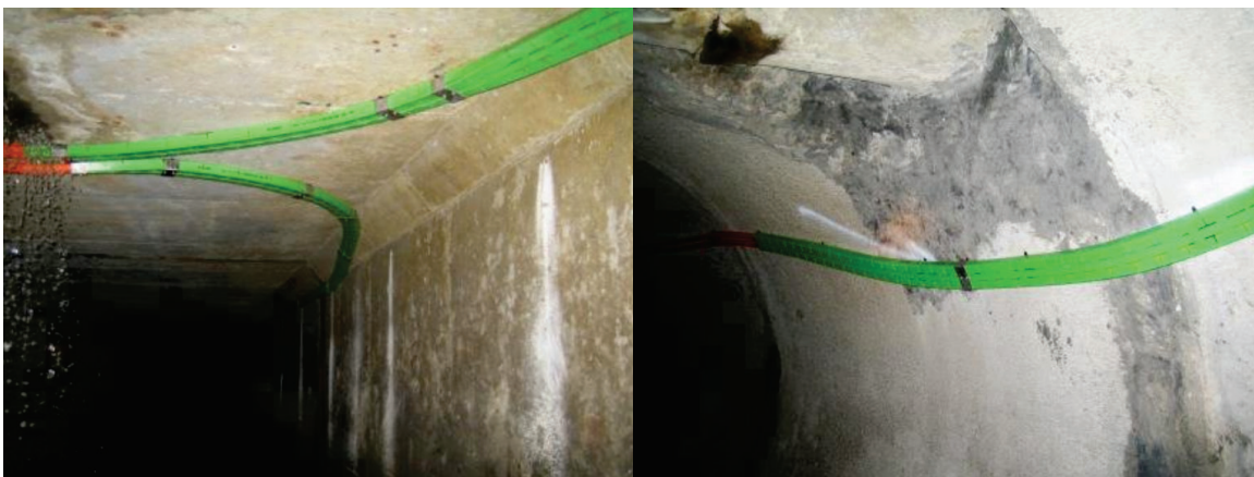
Figure 2-4: CableRunner installation in Heights Hilltop Interceptor in Cleveland, Ohio.
