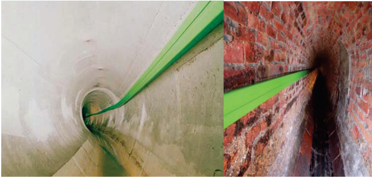
Figure 2-1: CableRunner technology installed in an accessible sewer of diameter greater than 80 cm (30 in).
