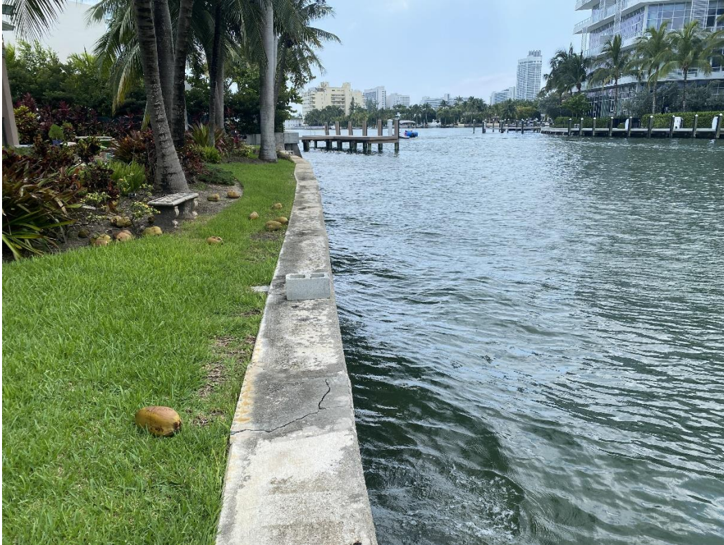
Photograph 1: View of existing seawall and yard facing east.
