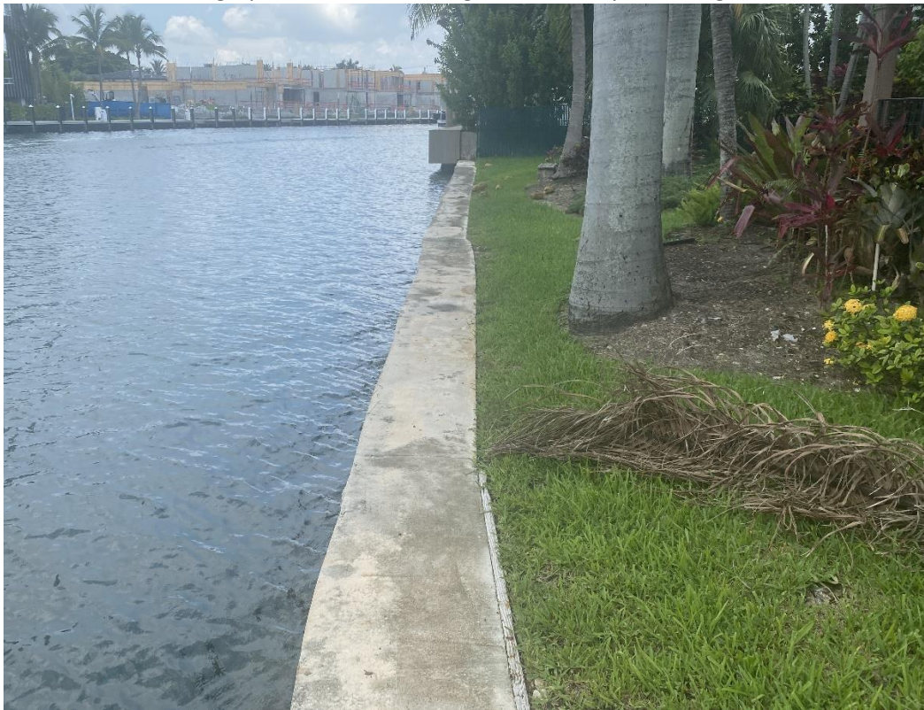
Photograph 2: View of existing seawall and yard facing west.
