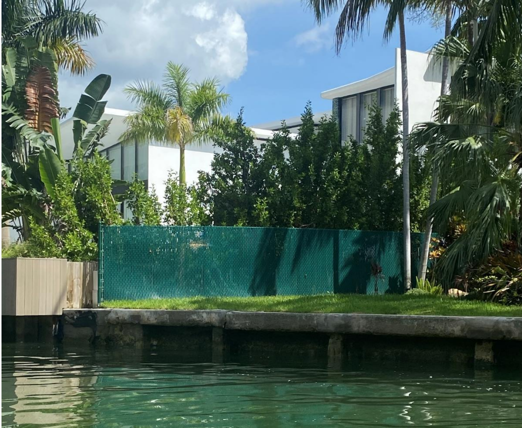
Photograph 5: View of existing seawall and neighboring seawall facing west.
