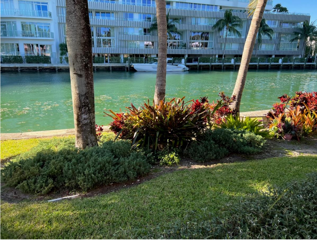
Photograph 3: View of existing seawall and yard facing the canal to the south.
