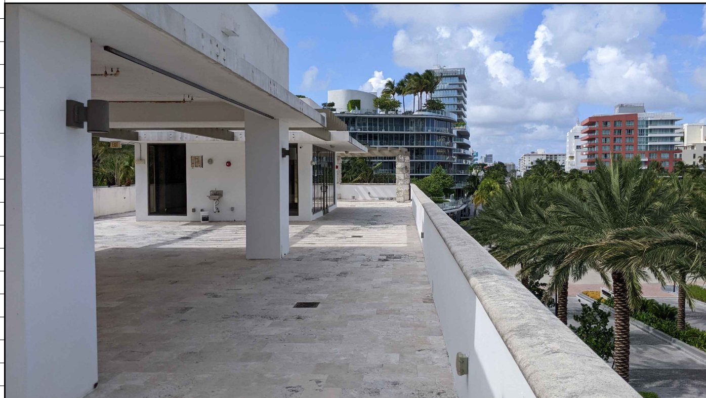
B NORTH-EAST EXTERIOR ROOF - EXISTING SCALE: NTS
