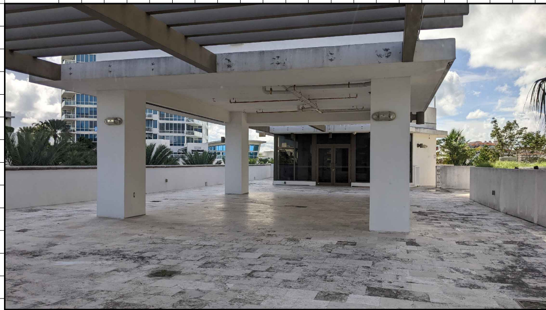
A SOUTH EXTERIOR ROOF - EXISTING SCALE: NTS
