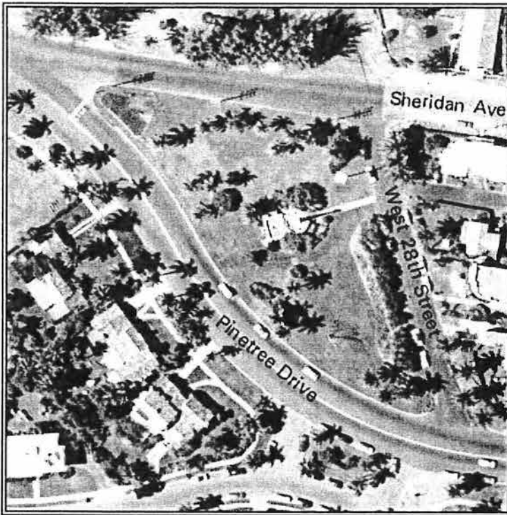
Figure 24 A small addition was built in 1948 on the south side (left) of the 28th Street Obelisk and Pumping Station to house an electrical generator, as seen in this 1954 aerial photo. The original landscape wall and steps may have been removed at the same time this addition was constructed.
