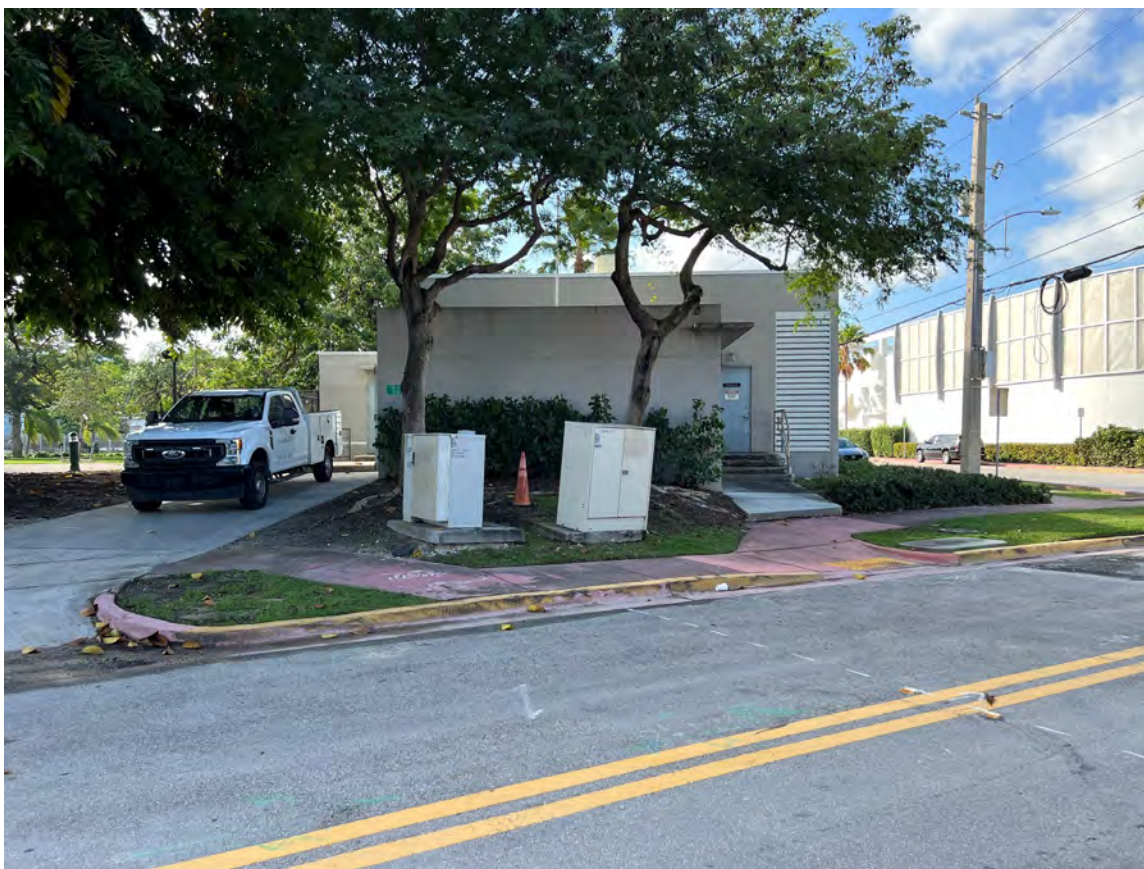
VIEW OF EXISTING BUILDING – NORTH FACADE
