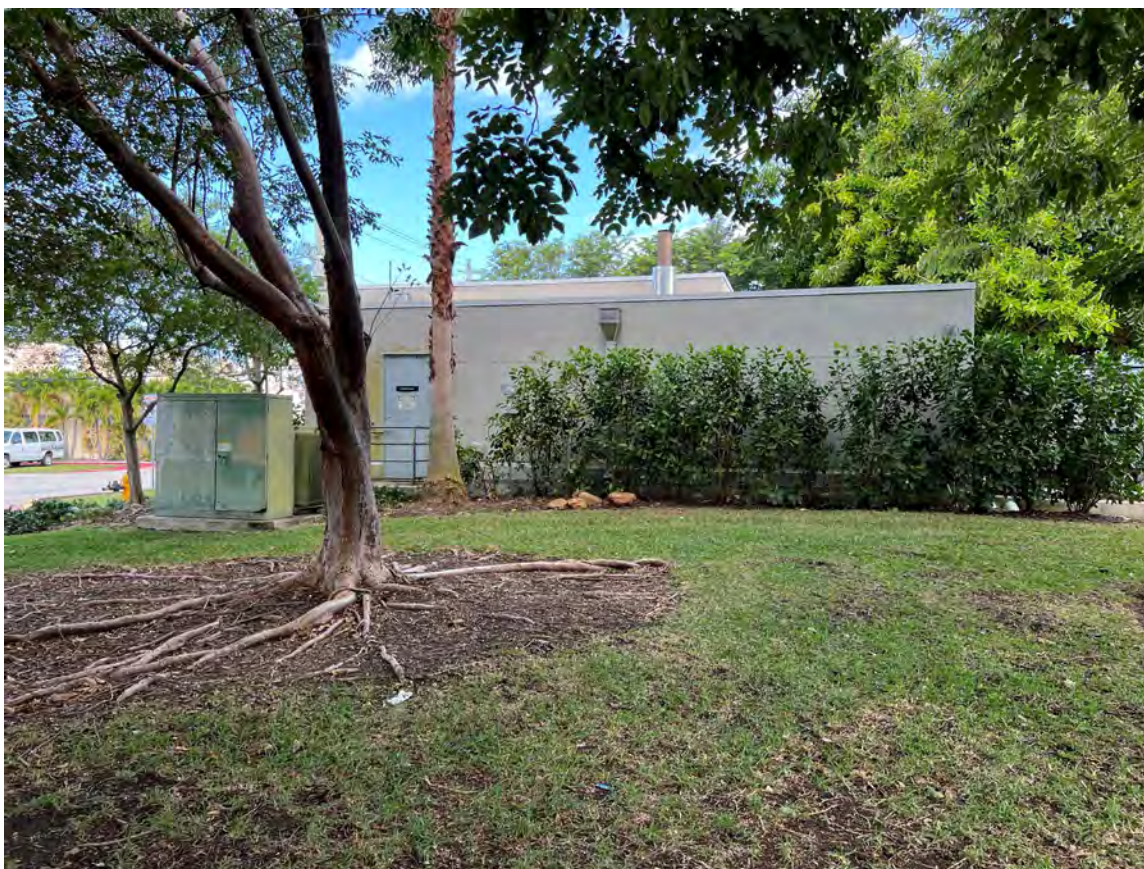
VIEW OF EXISTING BUILDING – SOUTH FACADE
