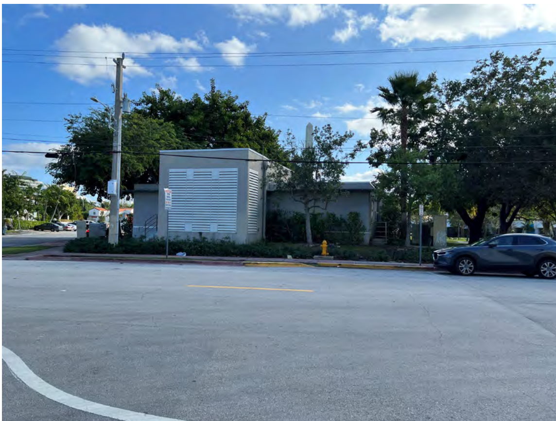
VIEW OF EXISTING BUILDING – WEST FACADE
