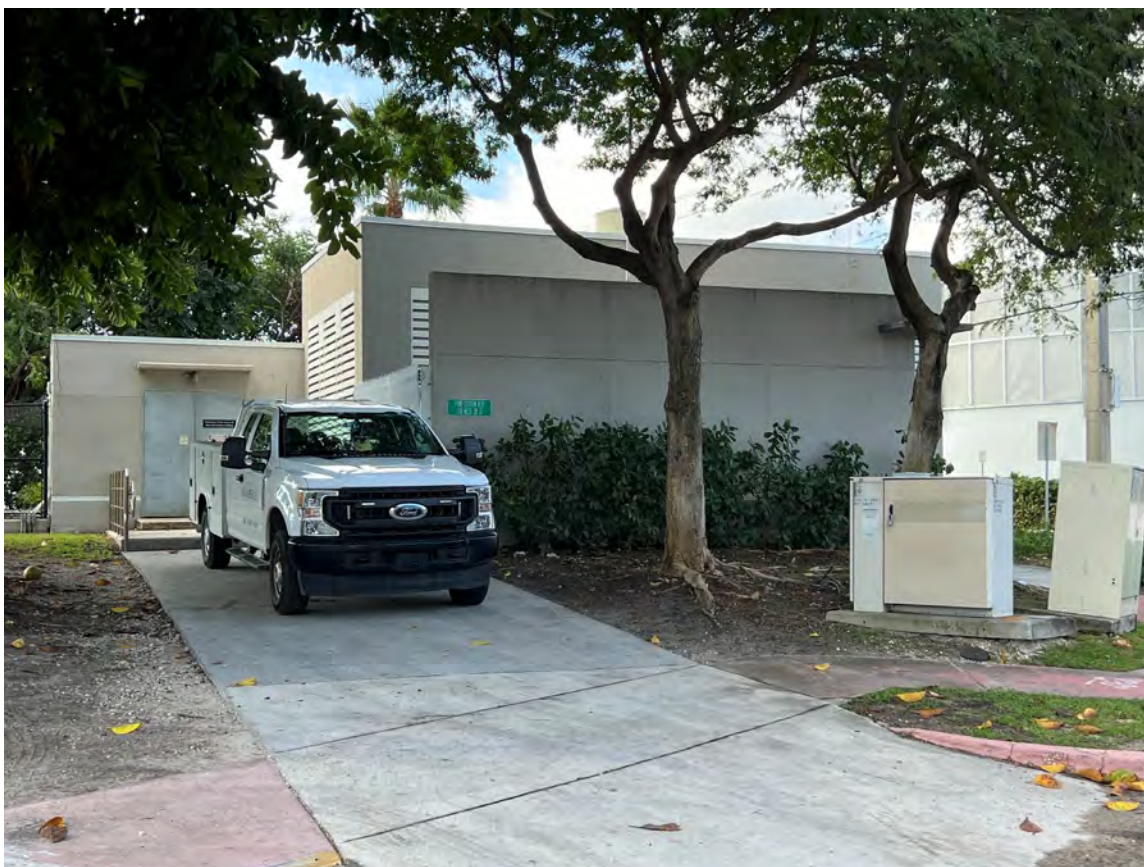
VIEW OF EXISTING BUILDING – NORTH FACADE
