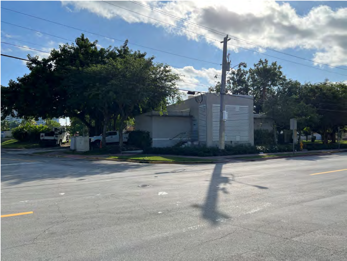
VIEW OF EXISTING BUILDING – NW CORNER
