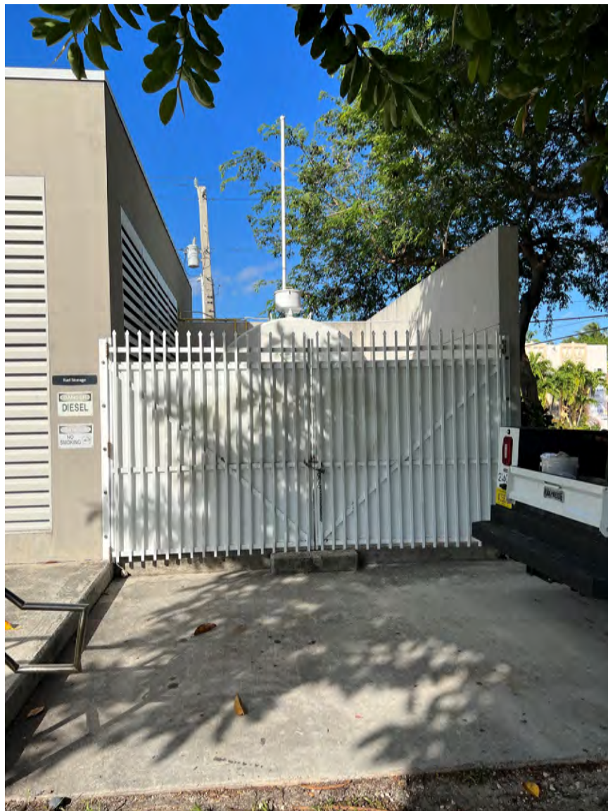
VIEW OF EXISTING BUILDING (FUEL TANK ENCLOSURE) – EAST FACADE
