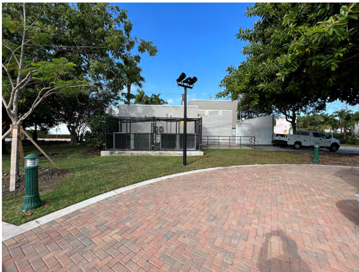
VIEW OF EXISTING BUILDING – EAST SIDE
