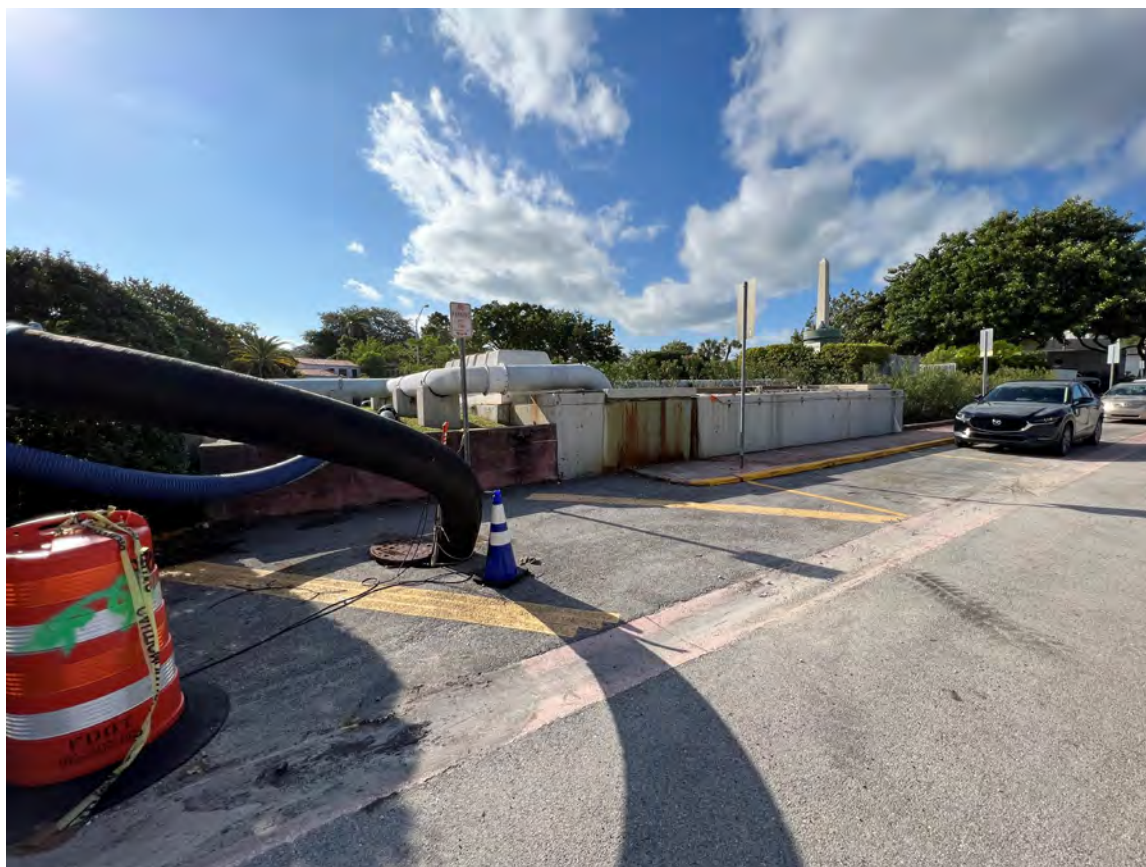
VIEW OF SITE – NORTH SIDE
