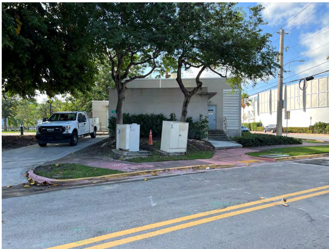
VIEW OF EXISTING BUILDING – NORTH FACADE
