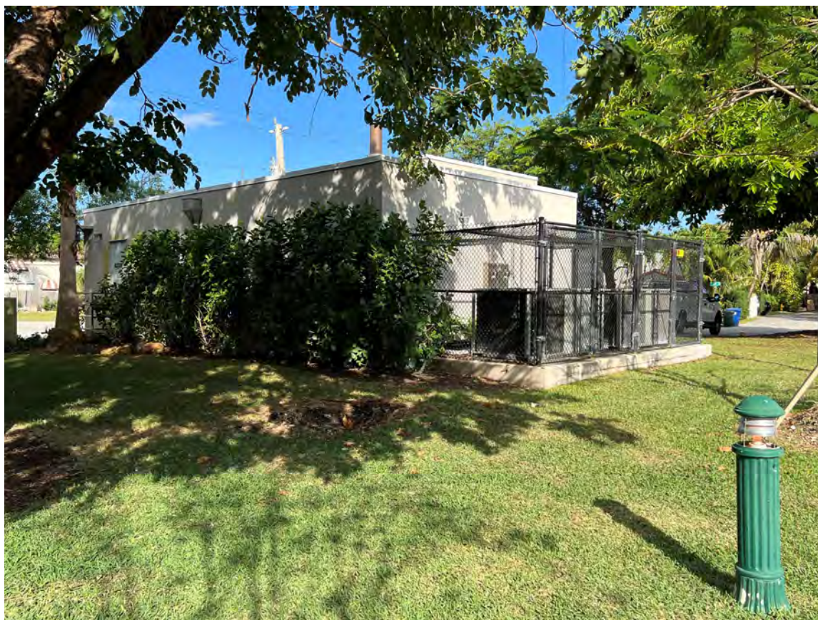
VIEW OF EXISTING BUILDING – SE CORNER
