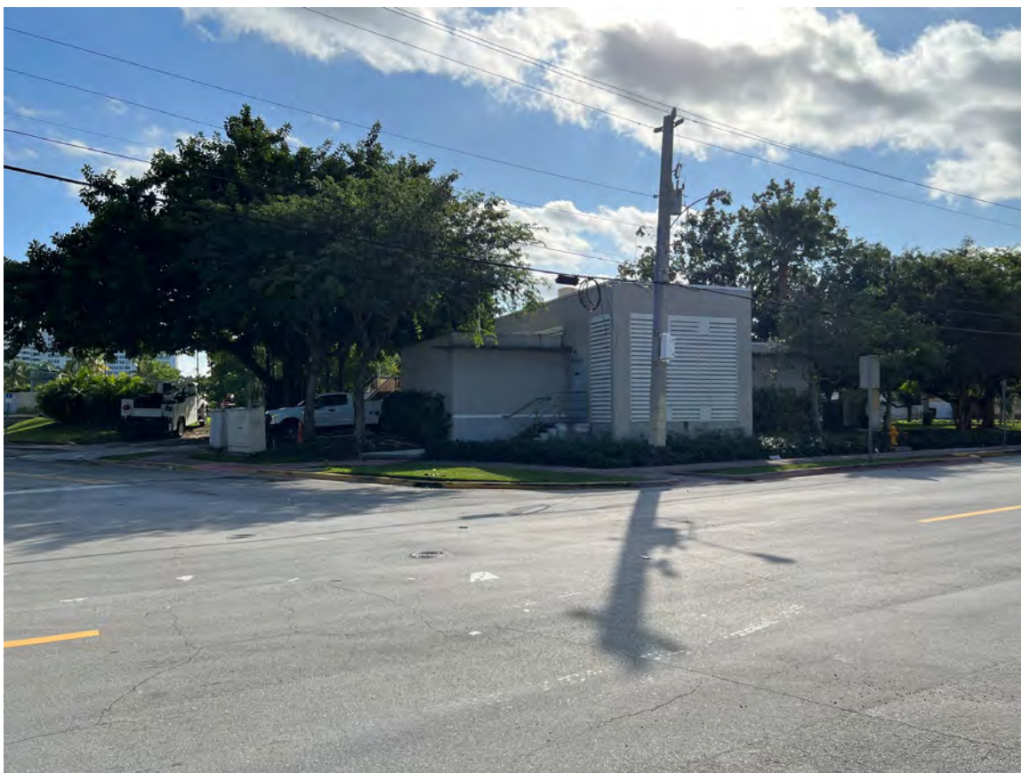
VIEW OF EXISTING BUILDING – NW CORNER
