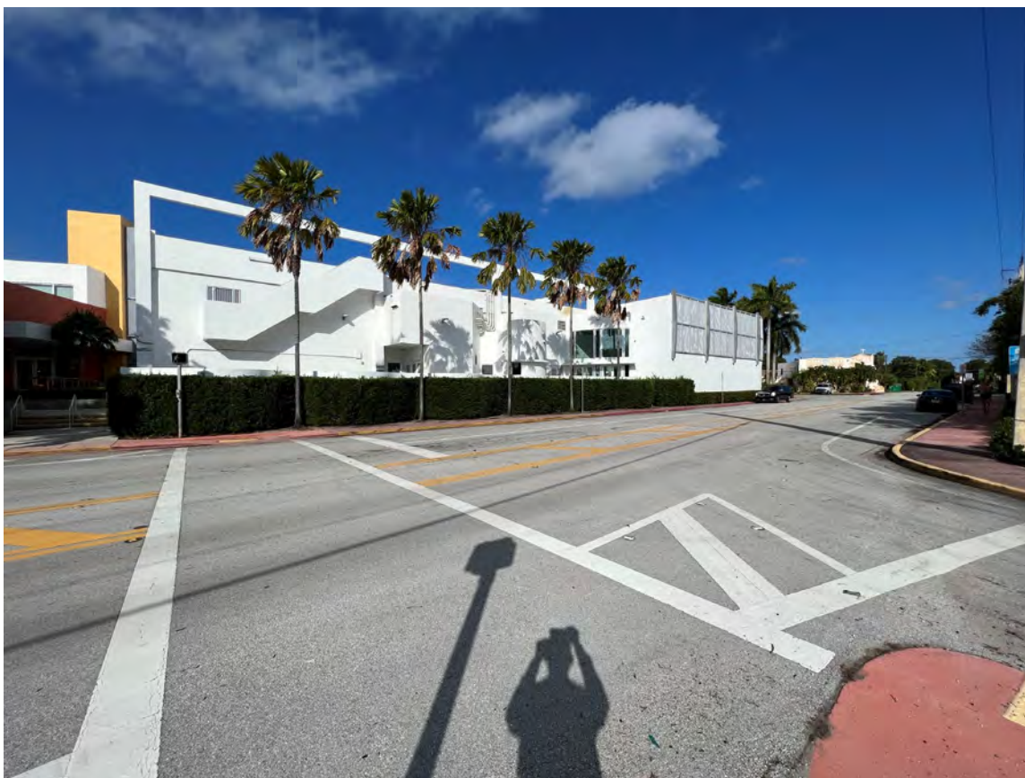
VIEW OF NEIGHBORING PROPERTY – WEST SIDE
