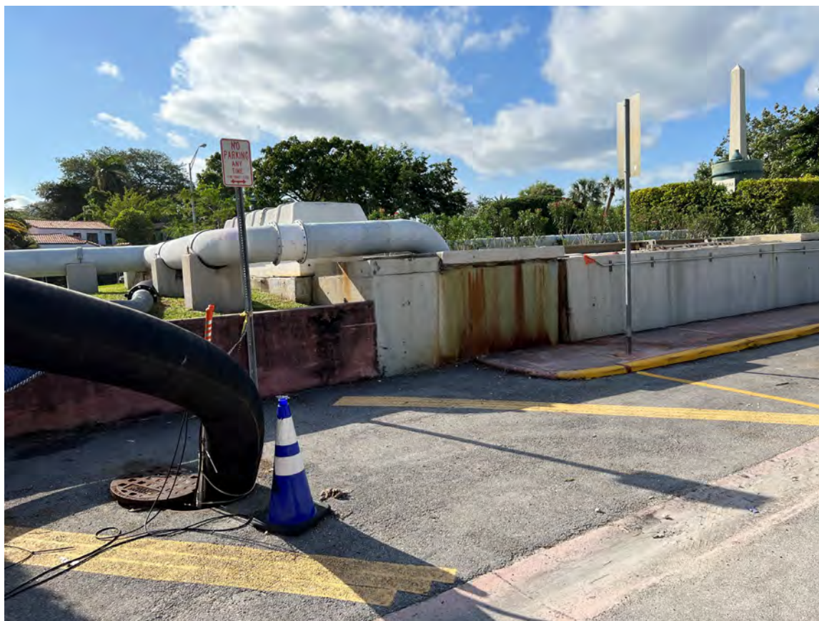
VIEW OF SITE – NORTH SIDE
