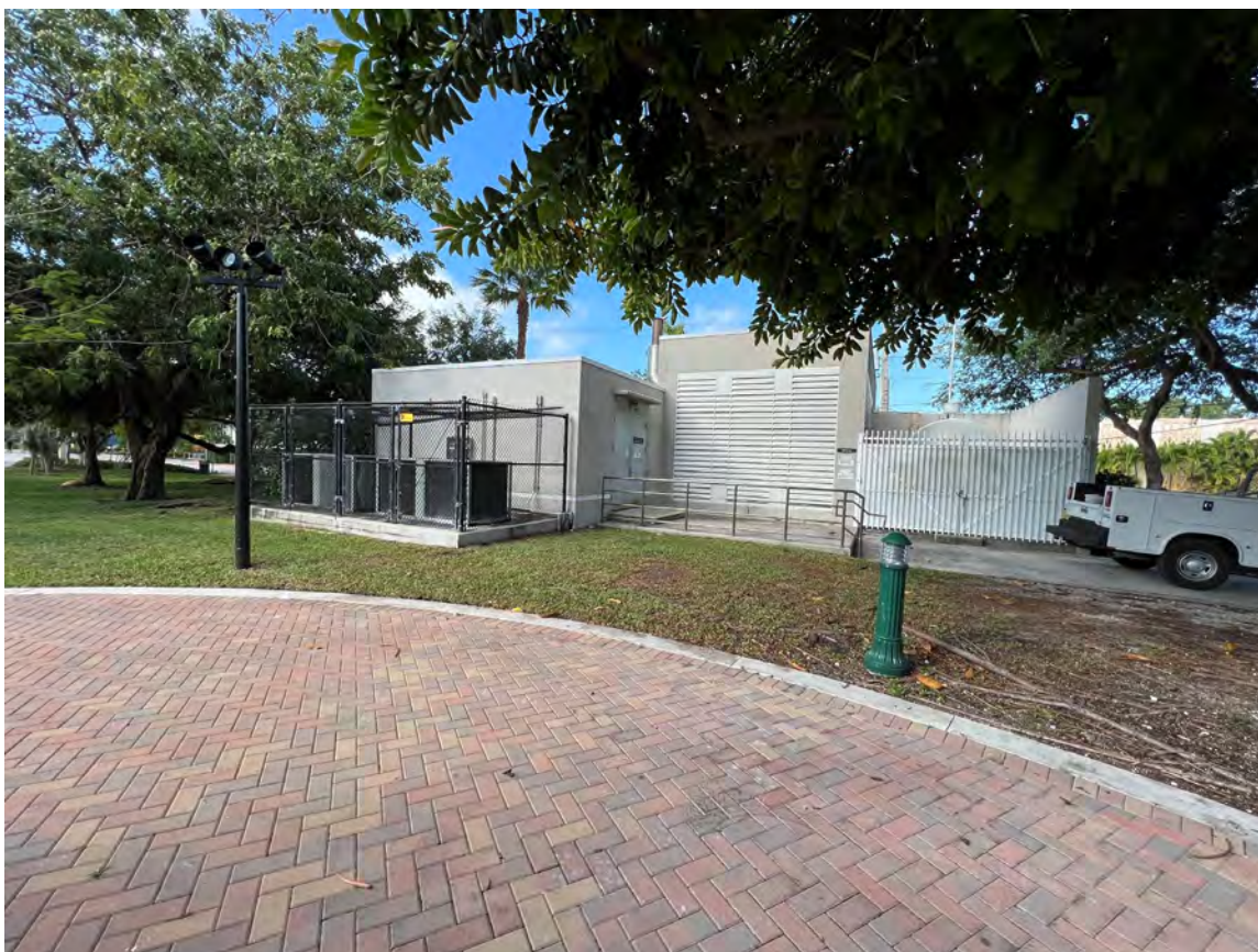
VIEW OF EXISTING BUILDING – EAST FACADE
