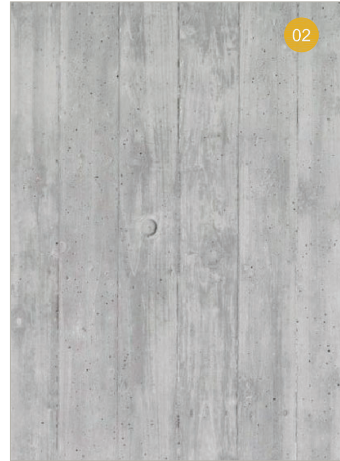
02 ARCHITECTURAL CONCRETE - BOARD FORMED @ FACADE TREATMENT
