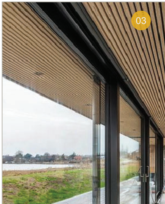
03 WOOD PLANK CEILING SYSTEM @ BALCONIES & OVERHANGS
