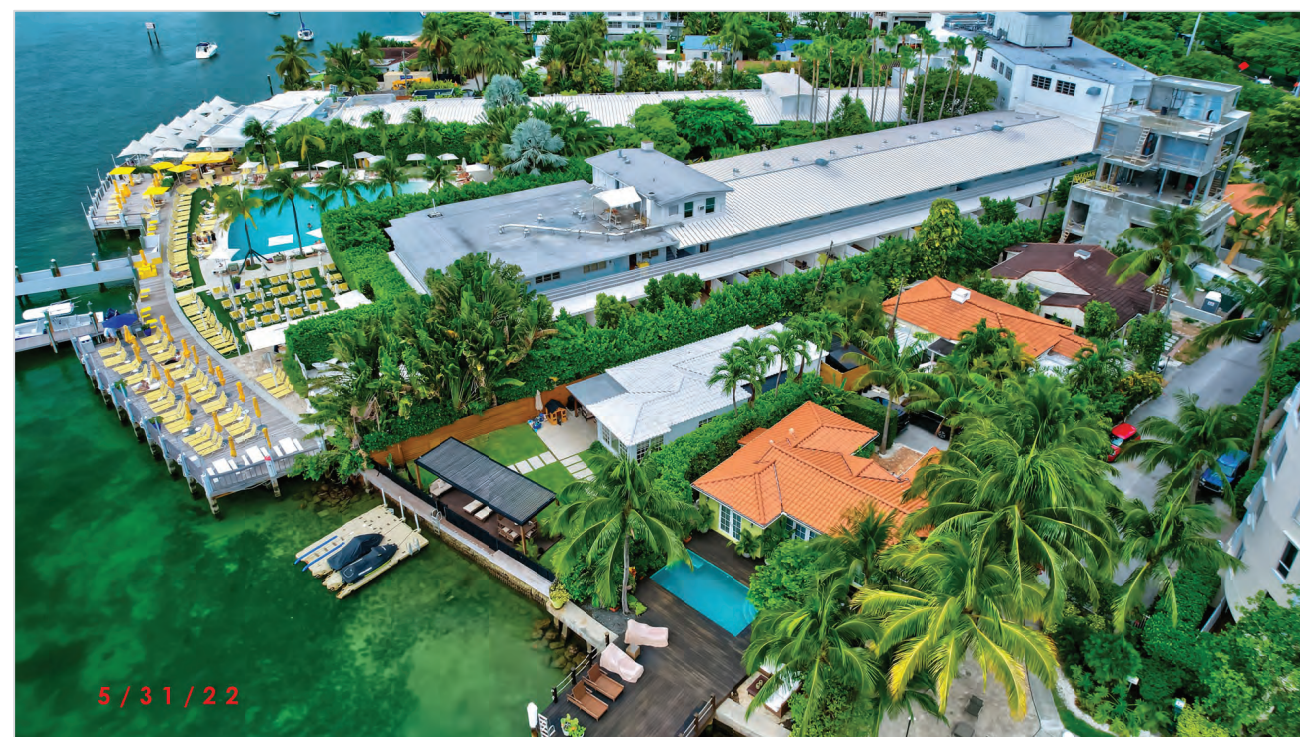
VIEW OF SITE FROM WATERWAY 01
