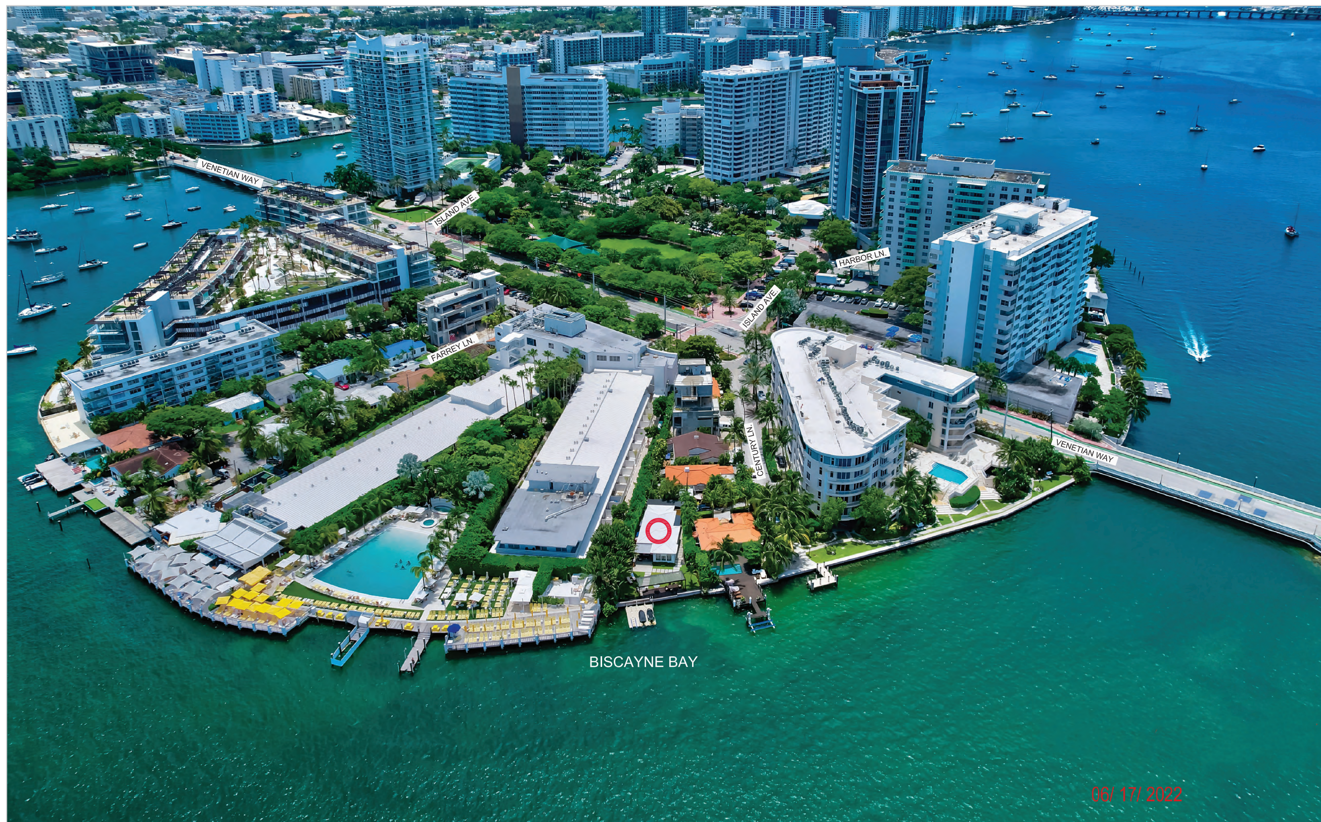
AERIAL VIEW OF BELLE ISLE & VENETIAN CROSSWAY
