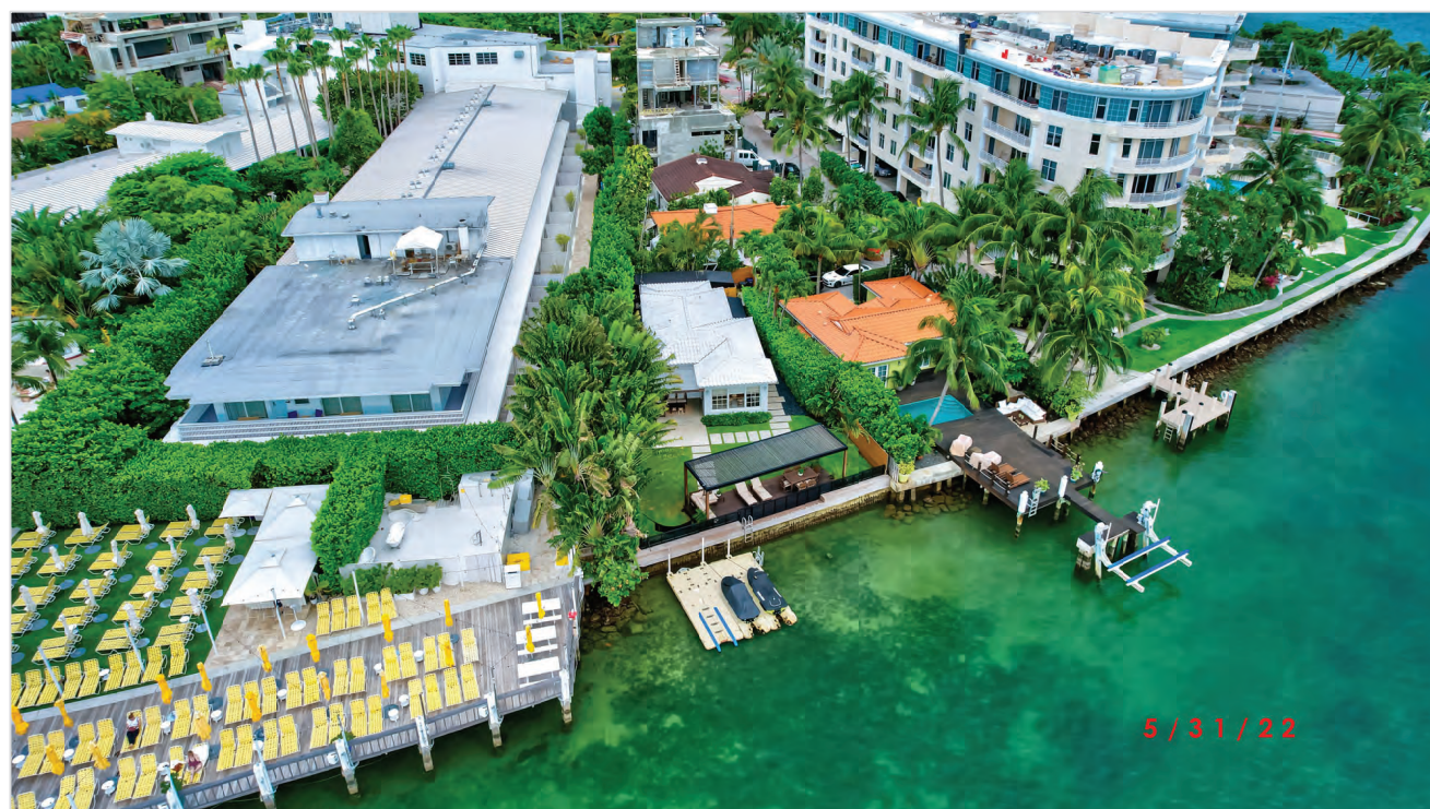
VIEW OF SITE FROM WATERWAY 02
