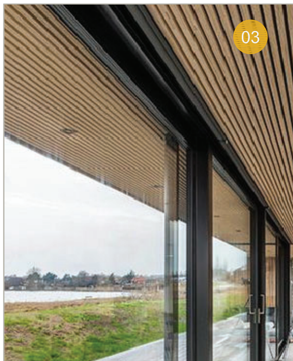
03 WOOD PLANK CEILING SYSTEM @ BALCONIES & OVERHANGS
