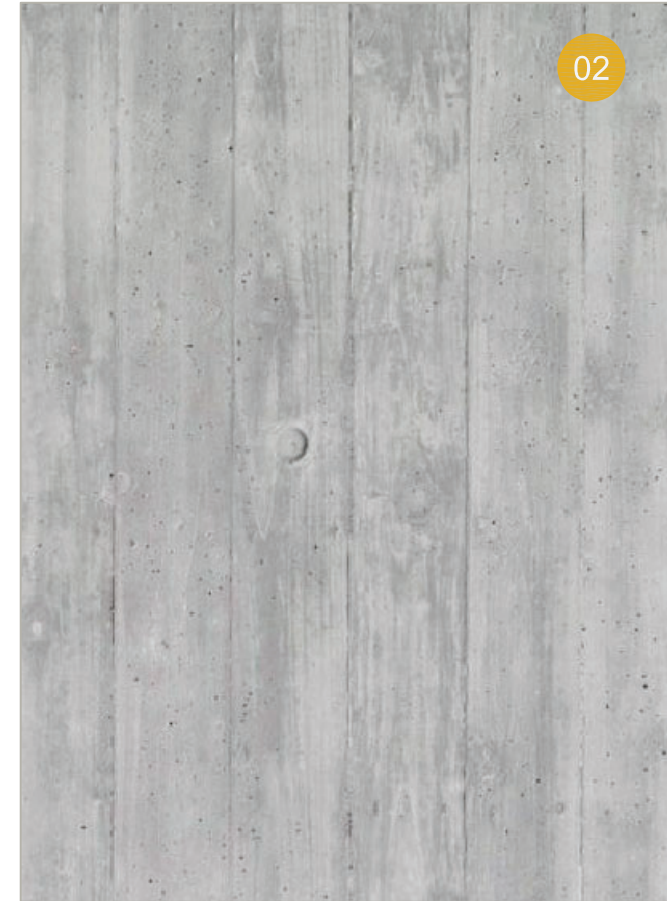
02 ARCHITECTURAL CONCRETE - BOARD FORMED @ FACADE TREATMENT
