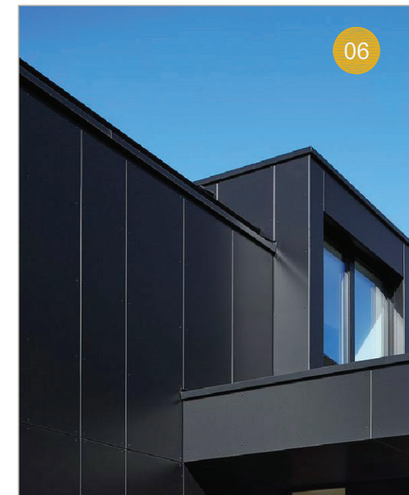
06 ALUMINUM CLAD SYSTEM @ BALCONIES EDGE
