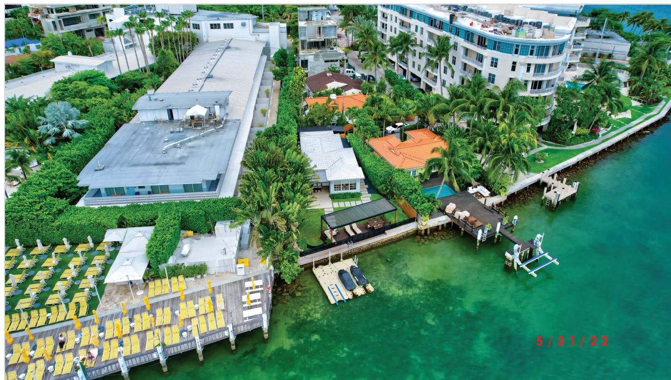
VIEW OF SITE FROM WATERWAY 02
