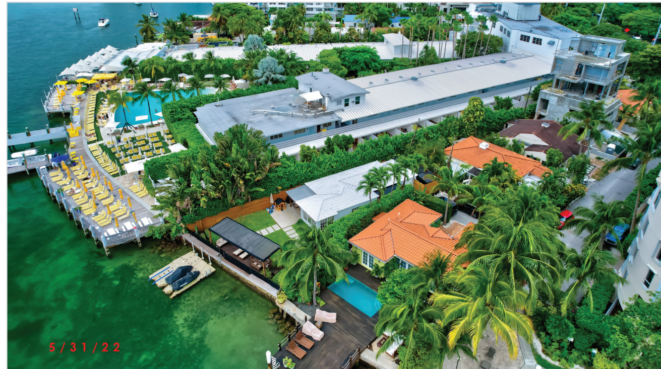
VIEW OF SITE FROM WATERWAY 01
