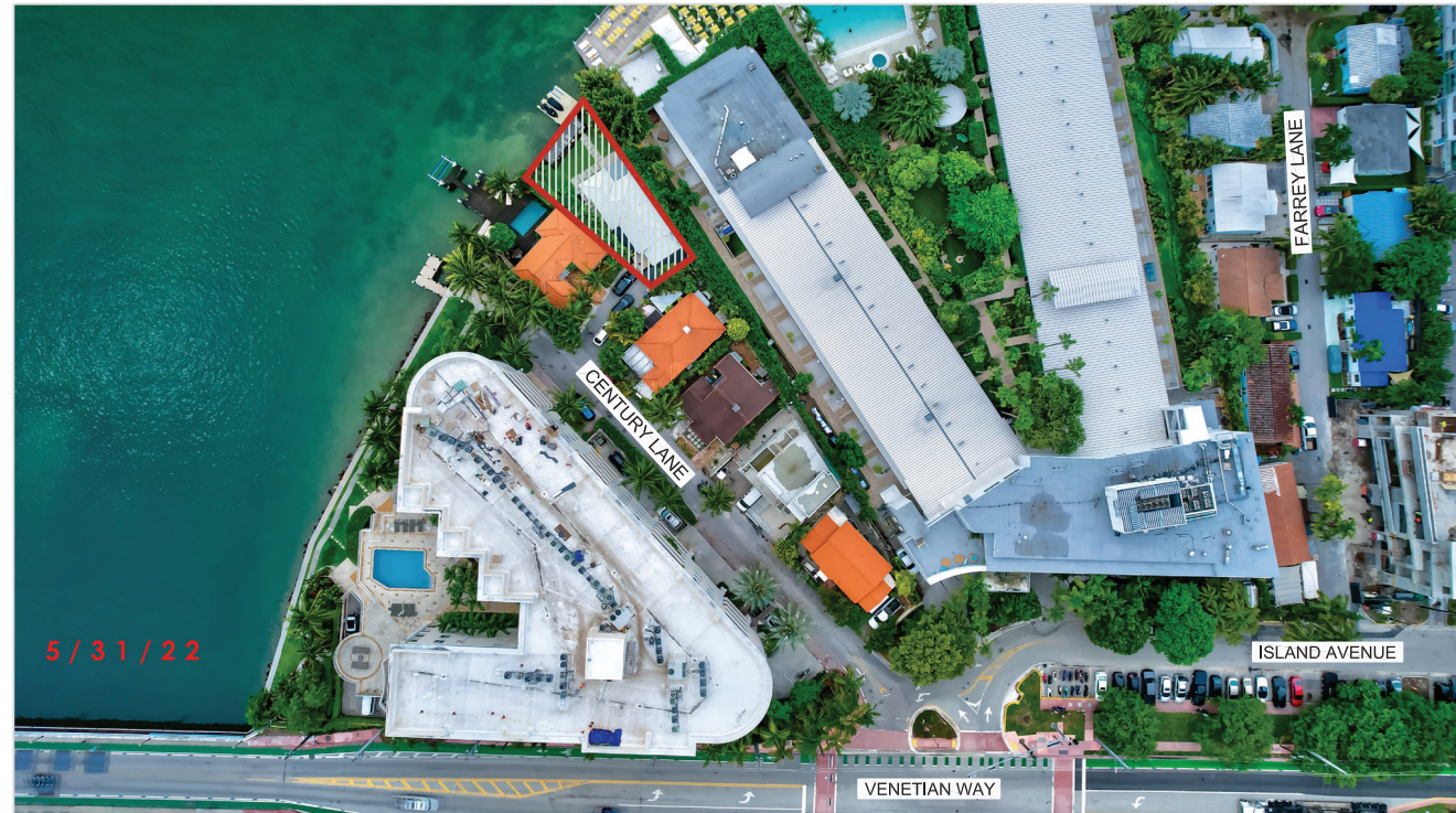
AERIAL VIEW OF SITE & SURROUNDINGS
