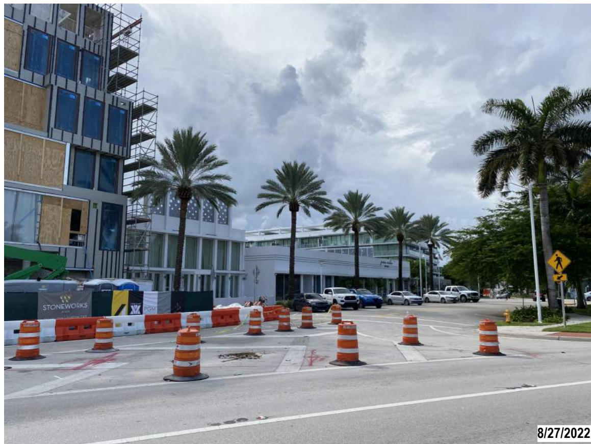
1. VIEW OF SITE FROM ALTON ROAD
