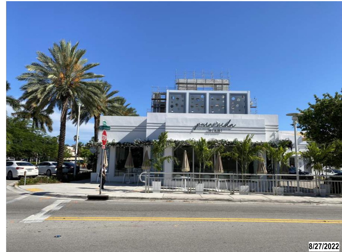
2. VIEW OF EXISTING STRUCTURES FROM 20TH STREET
