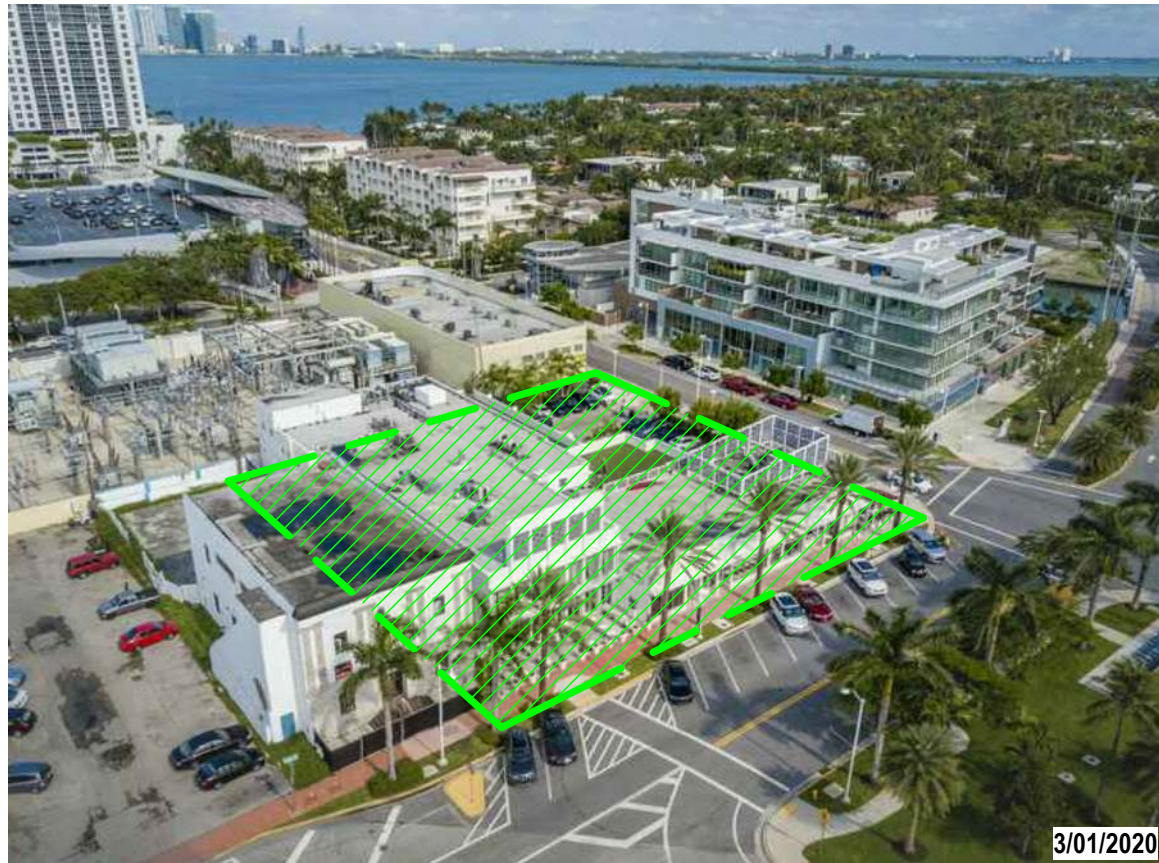
1. AERIAL OF SE CORNER OF SITE
