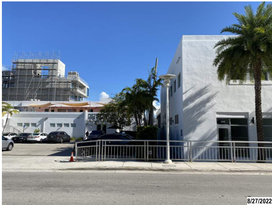
3. VIEW OF EXISTING STRUCTURES FROM WEST AVENUE
