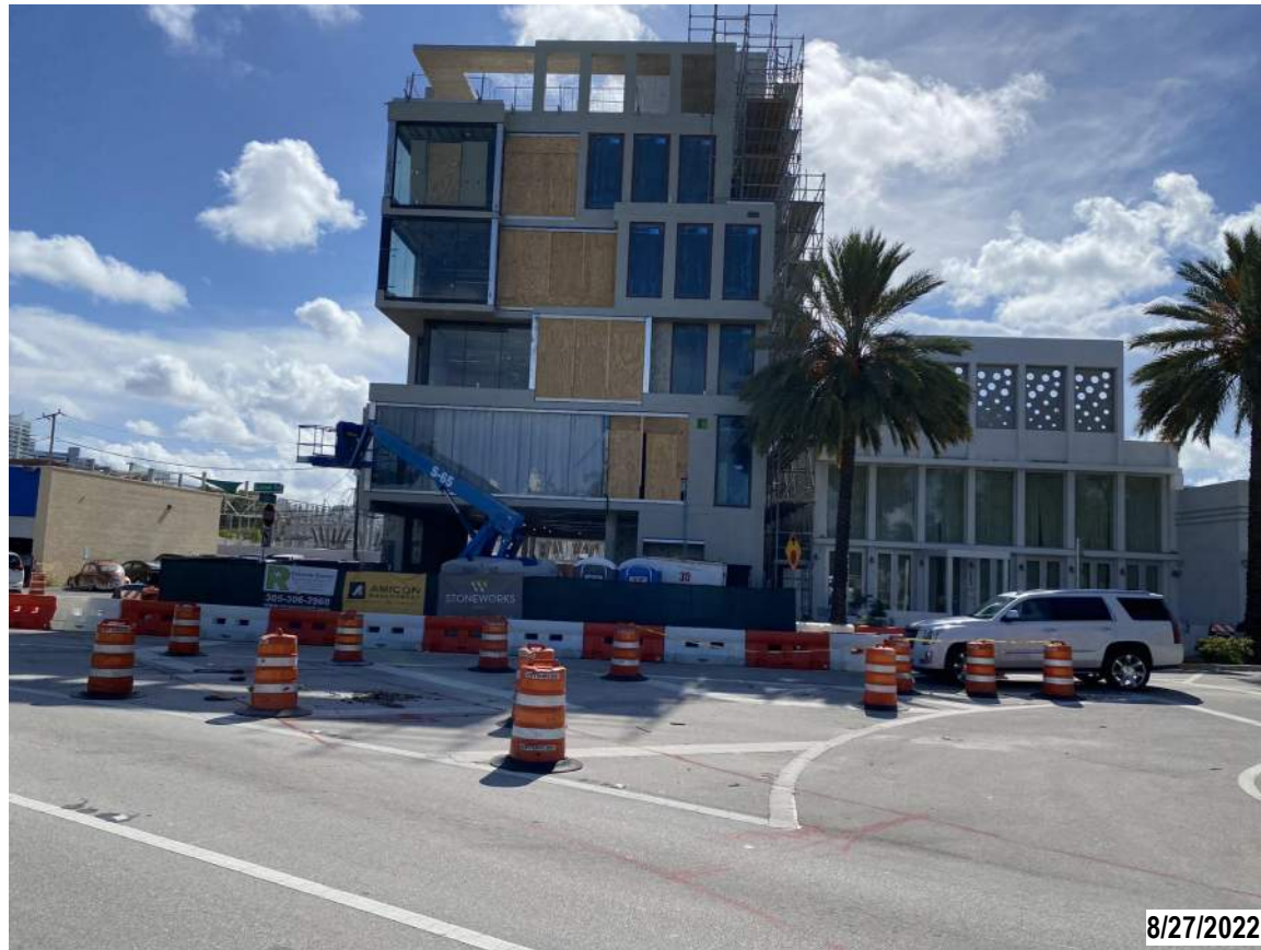
1. VIEW OF EXISTING STRUCTURES FROM ALTON ROAD
