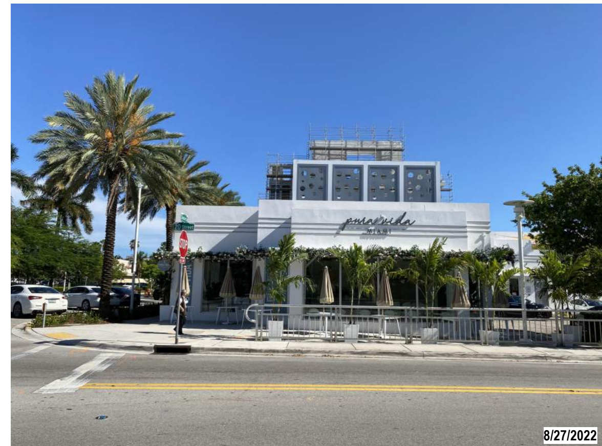
2. VIEW OF EXISTING STRUCTURES FROM 20TH STREET
