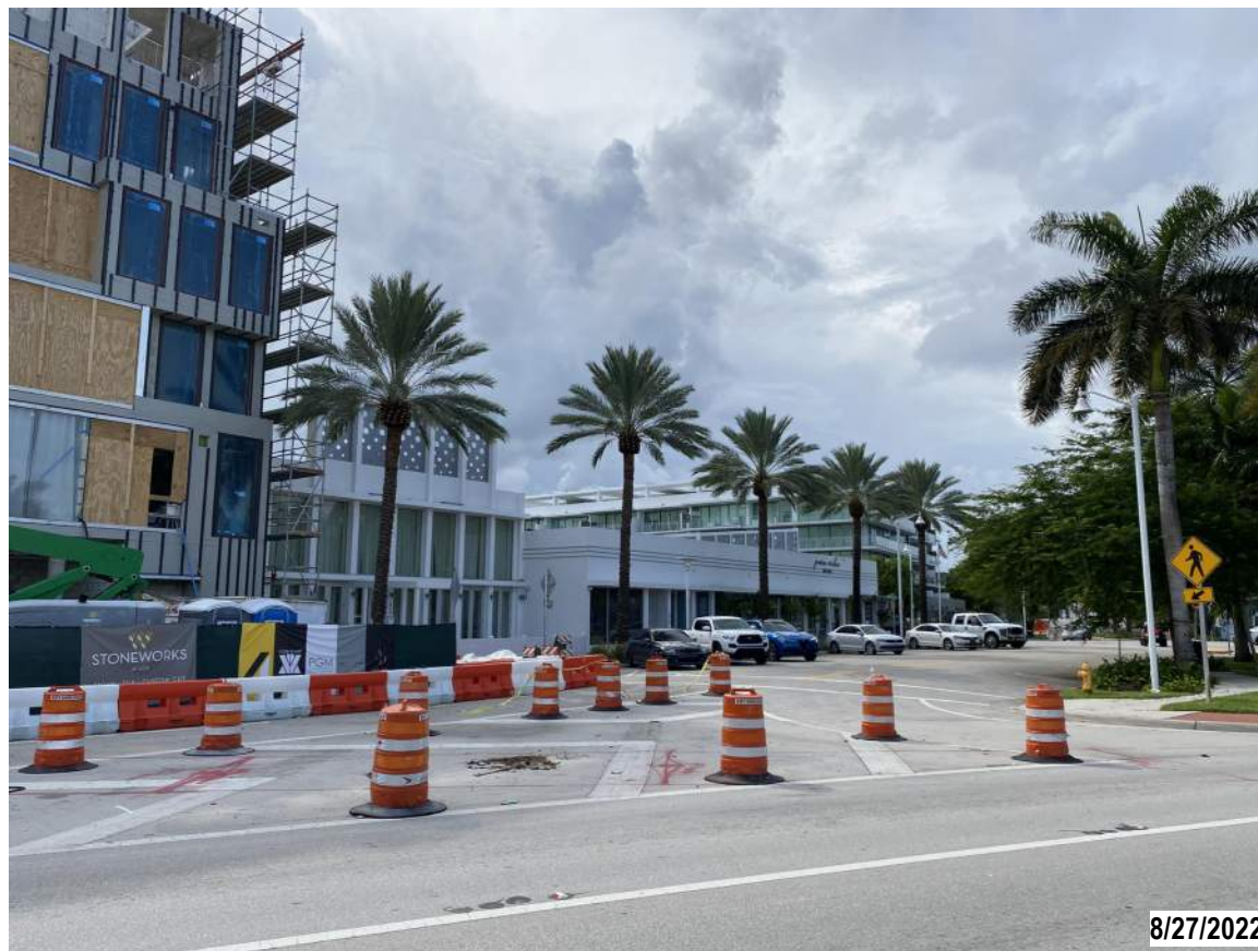
1. VIEW OF SITE FROM ALTON ROAD
