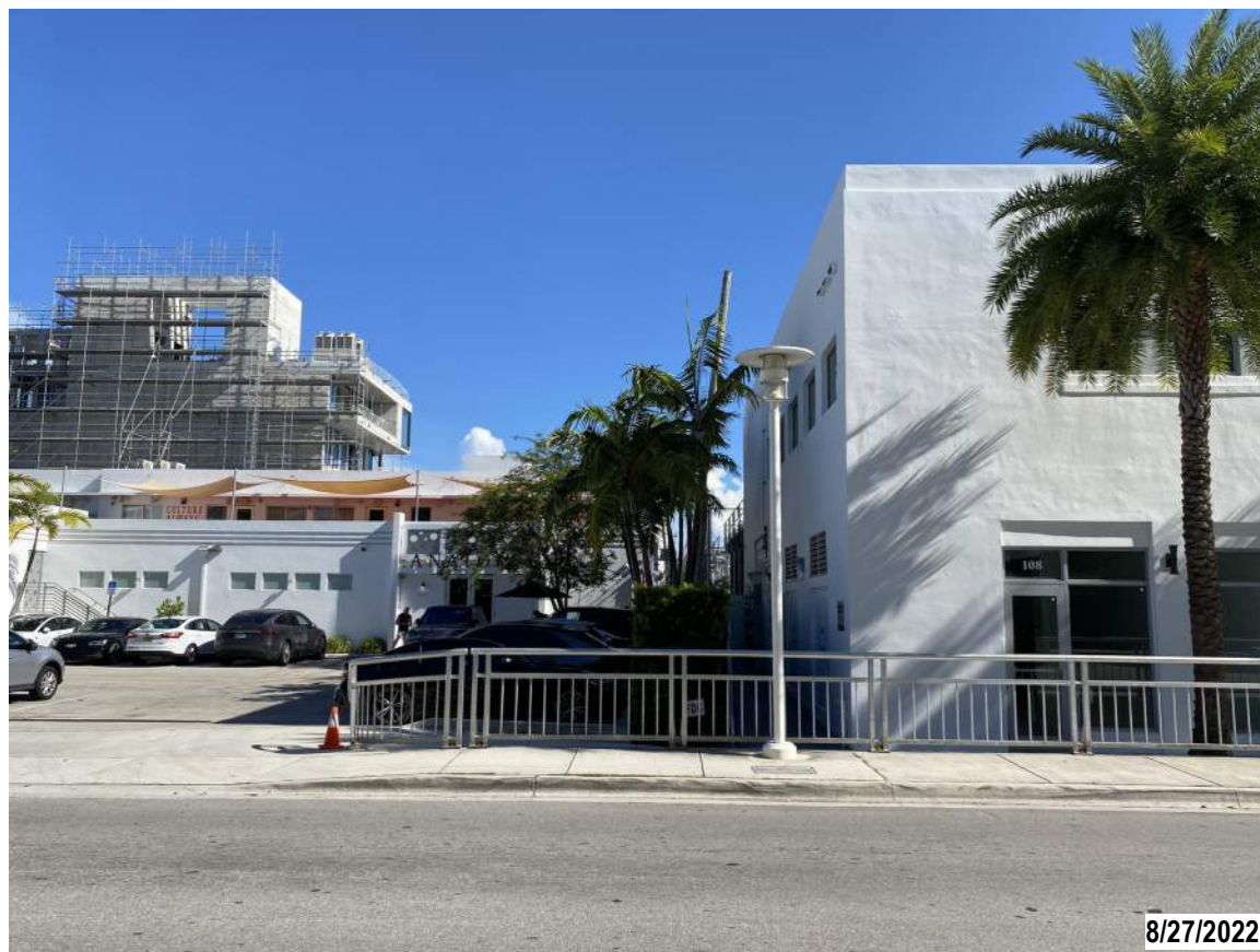
3. VIEW OF EXISTING STRUCTURES FROM WEST AVENUE
