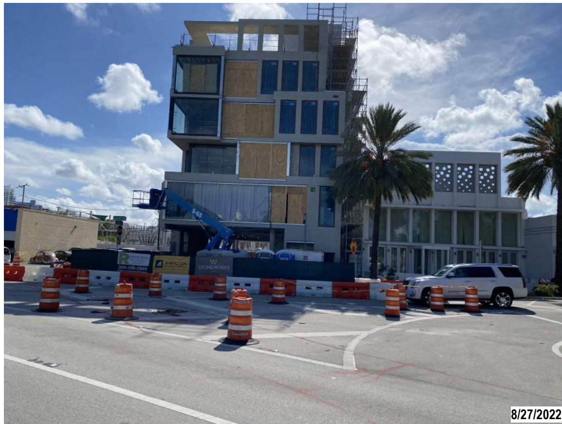
1. VIEW OF EXISTING STRUCTURES FROM ALTON ROAD
