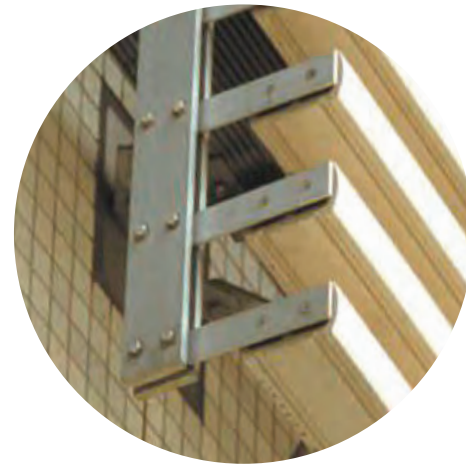
TERRACOTTA MECHANICAL SCREEN DESIGN BASIS: NBK TERRACOTTA - TERRART BAGUETTE 2" X 6" PROFILES, HORIZONTAL COLOR: 1.02-0 (GROUP 2)
