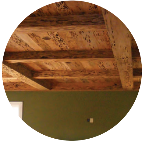
PECKY CYPRESS COFFERED CEILING DESIGN BASIS: CAPITOL CITY LUMBER PECKY CYPRESS T&G PANELING 1X6
