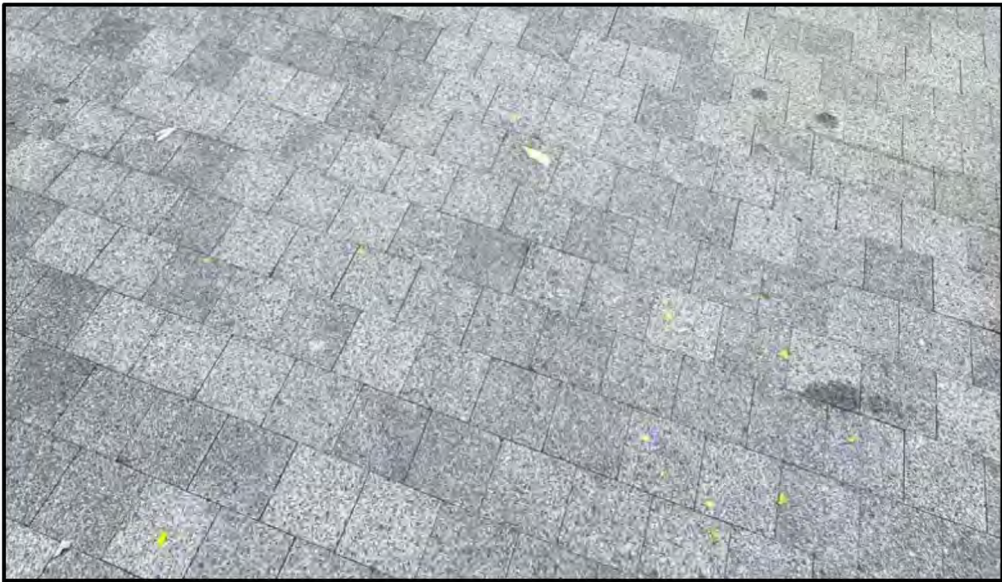
P-1 PAVERS AT DRIVEWAY BORDER: SQUARED PAVERS (GRAY STONE OR PRE-CAST CONCRETE)
