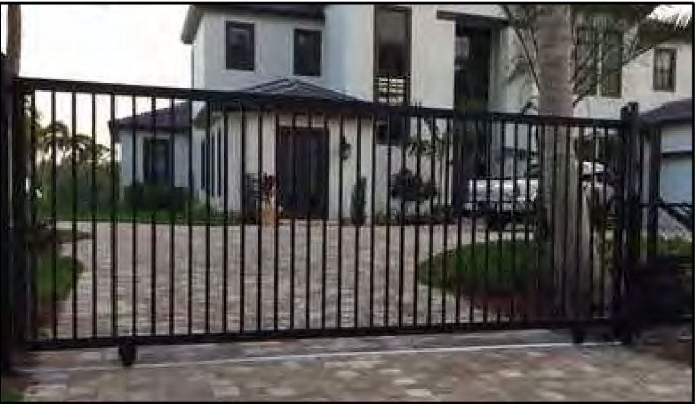
M-1 METAL AT PROPERTY FENCES & POOL GATES: BLACK ALUMINUM
