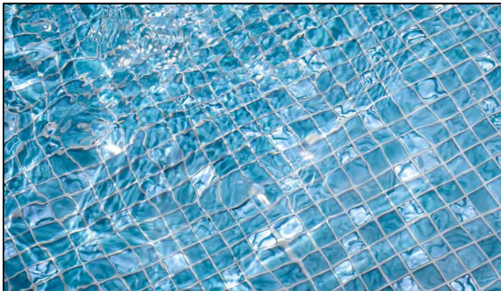
WT-1 OPT A WATERLINE TILE AT POOL & SPA: 1"x1" LIQUID ROCK BY ISLAND STONE (TILE GROUT COLOR TO MATCH TILE COLOR)
