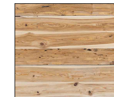
5 WOOD UNDERSIDE OF ROOF OVERHANGS
