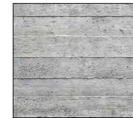
2 BOARD-FORMED CONCRETE
