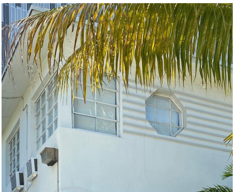
Spandrel with horizontal striping and Porthole Window Details. June 1st, 2020
