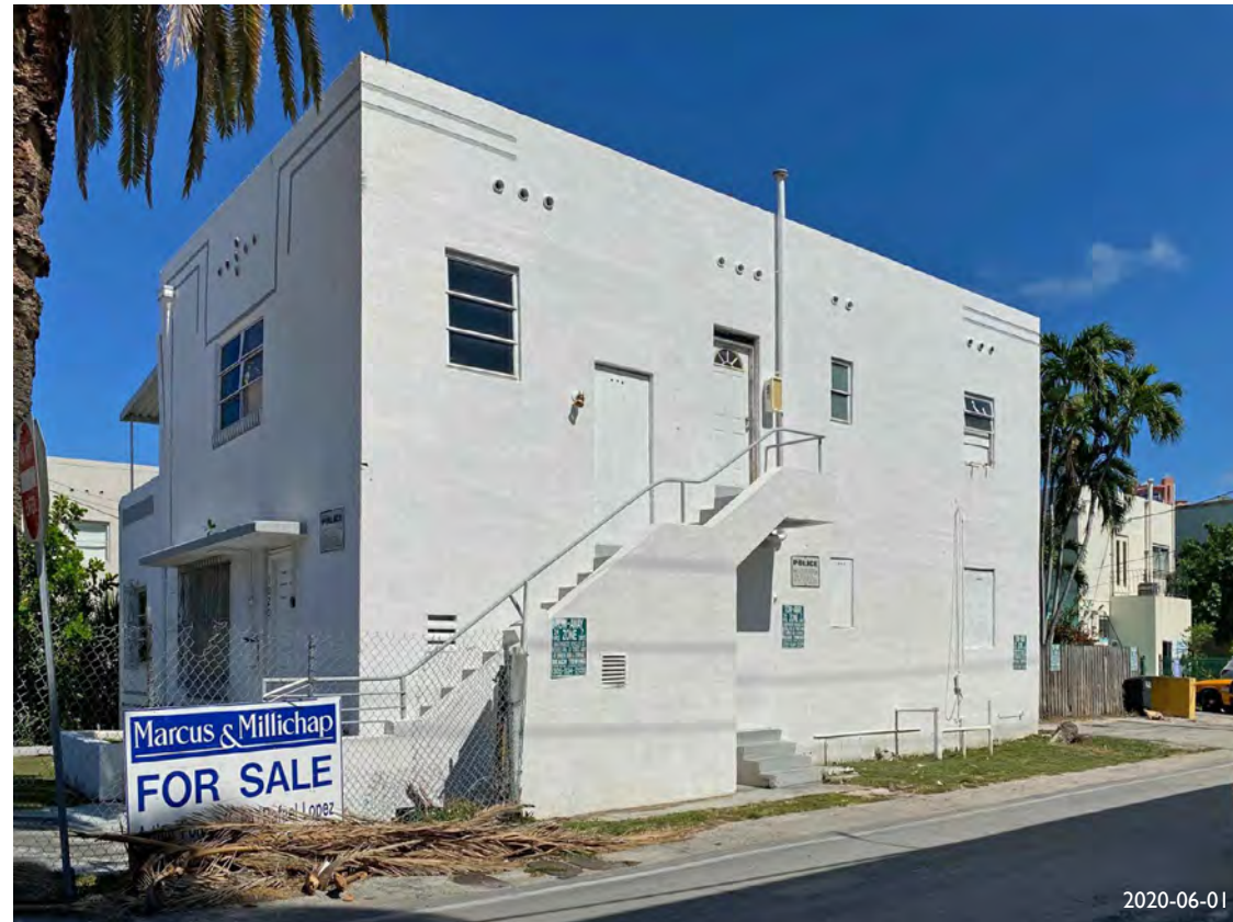
18. VIEW FROM THE SITE TOWARDS MICHIGAN COURT
