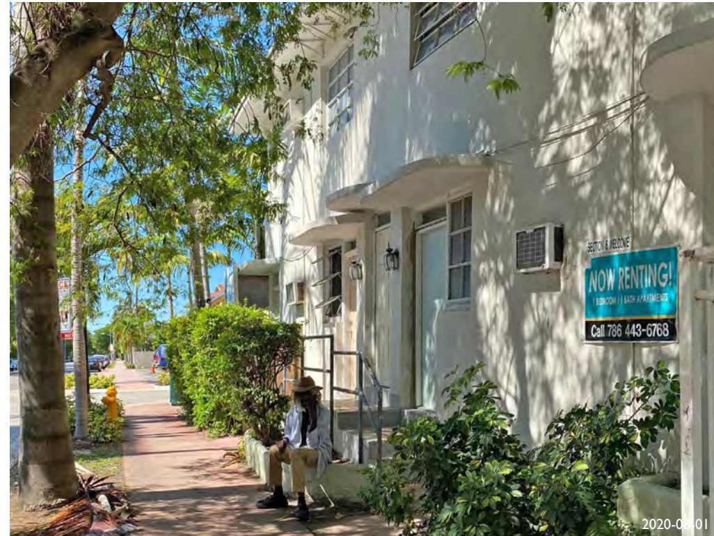
22. WEST BUILDING FACING LENOX AVENUE
