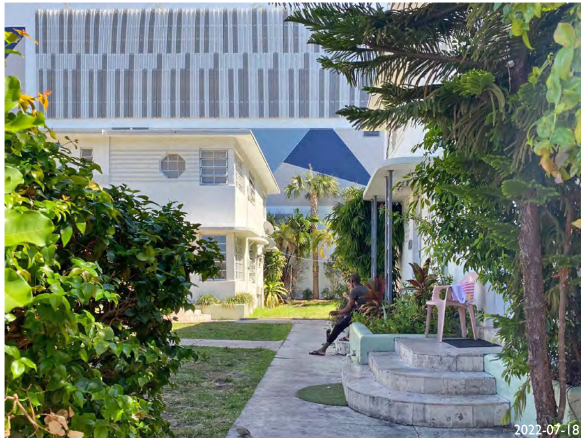
13. ENTRANCE OF EAST BUILDING
