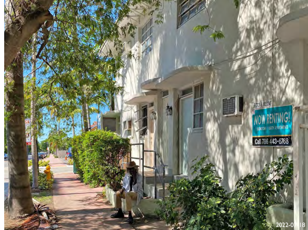
22. WEST BUILDING FACING LENOX AVENUE
