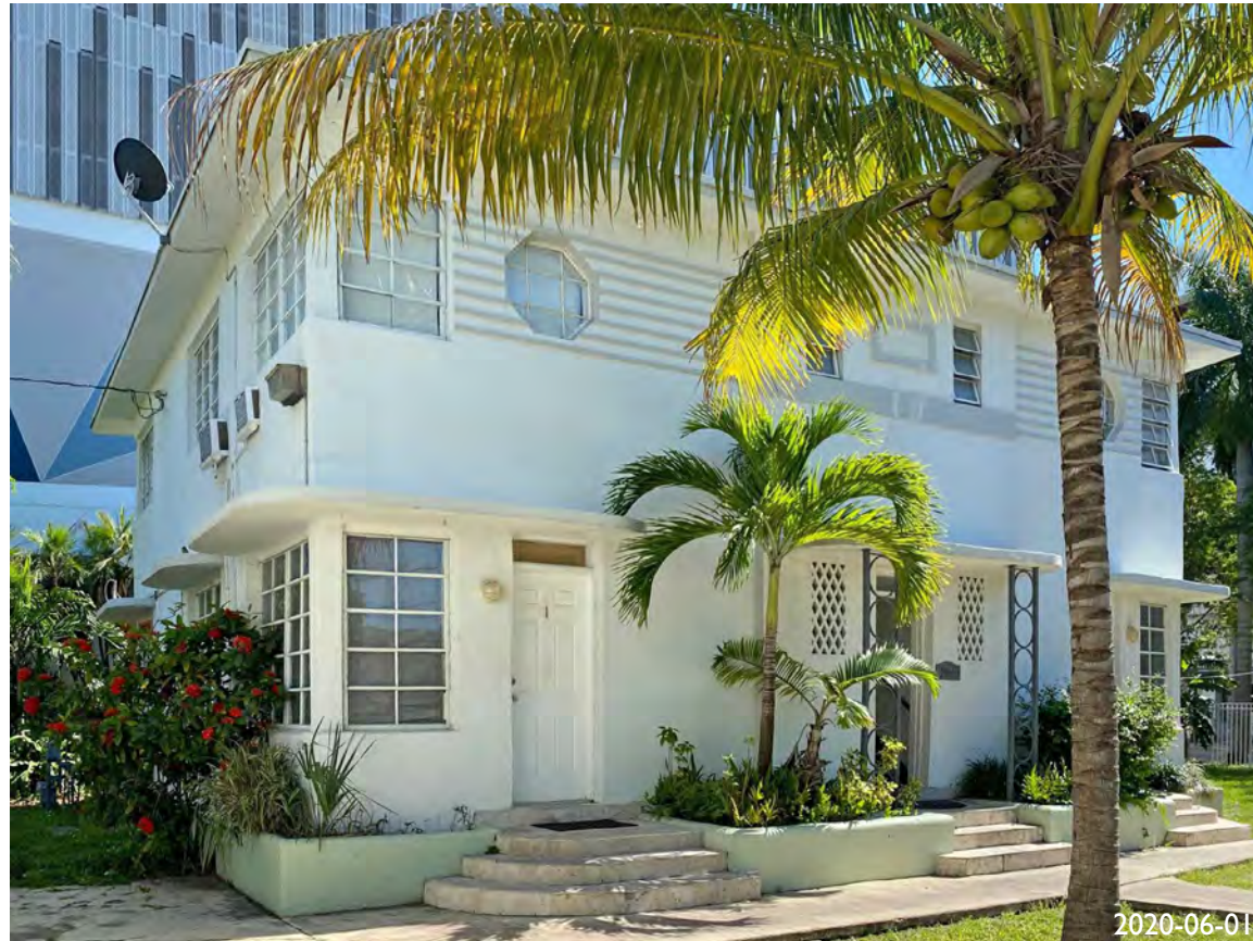
11. EXISTING SOUTH BUILDING
