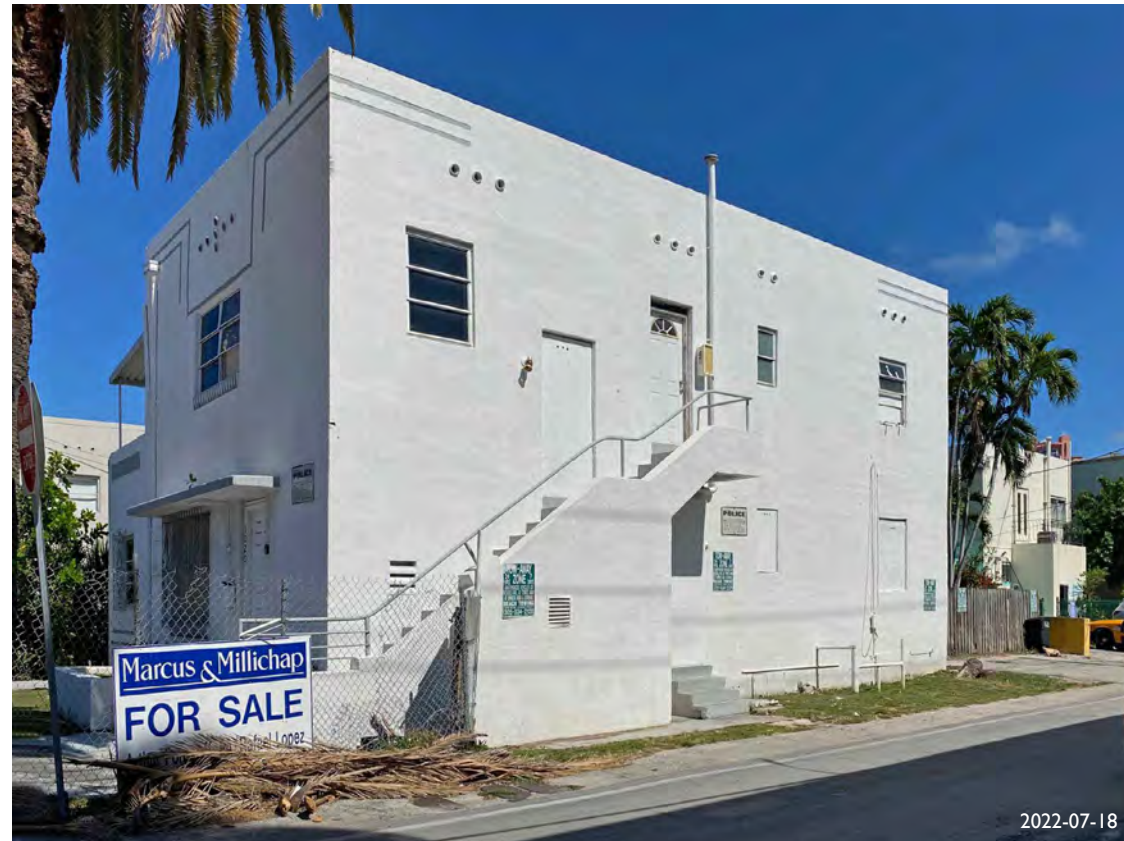
18. VIEW FROM THE SITE TOWARDS MICHIGAN COURT
