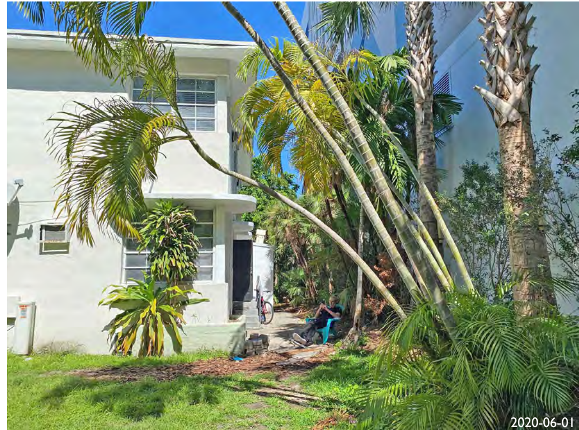
12. BACK OF SOUTH BUILDING AND ADJACENT RETAIL BUILDING
