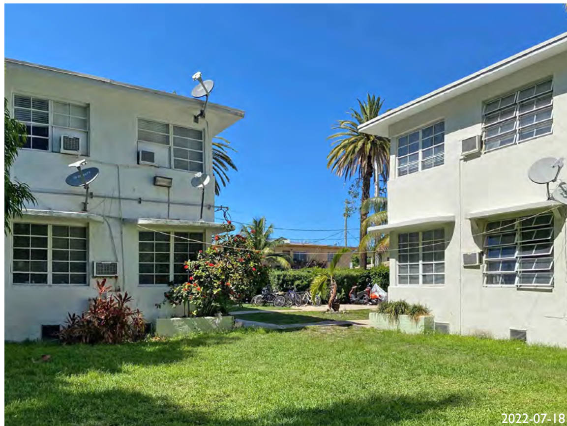
9. GREEN SPACE BETWEEN EAST AND SOUTH BUILDINGS
