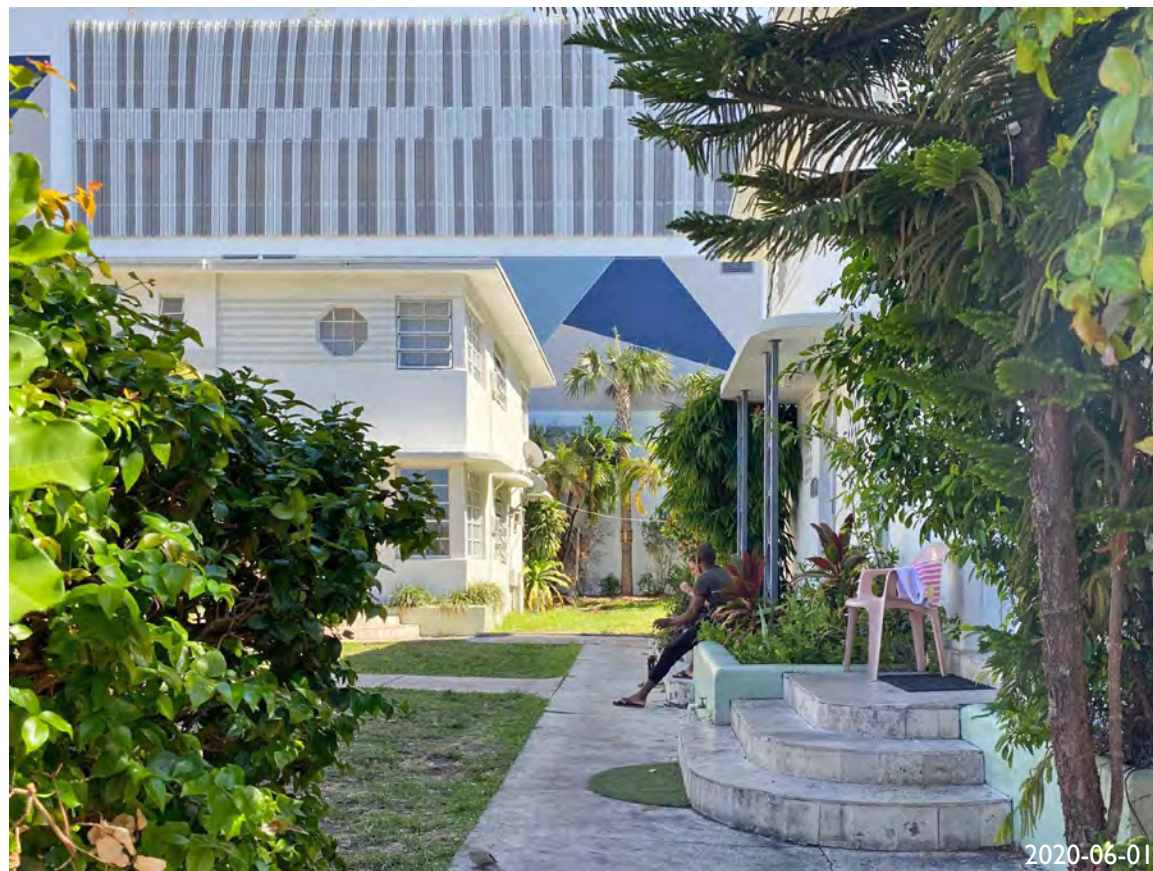
13. ENTRANCE OF EAST BUILDING
