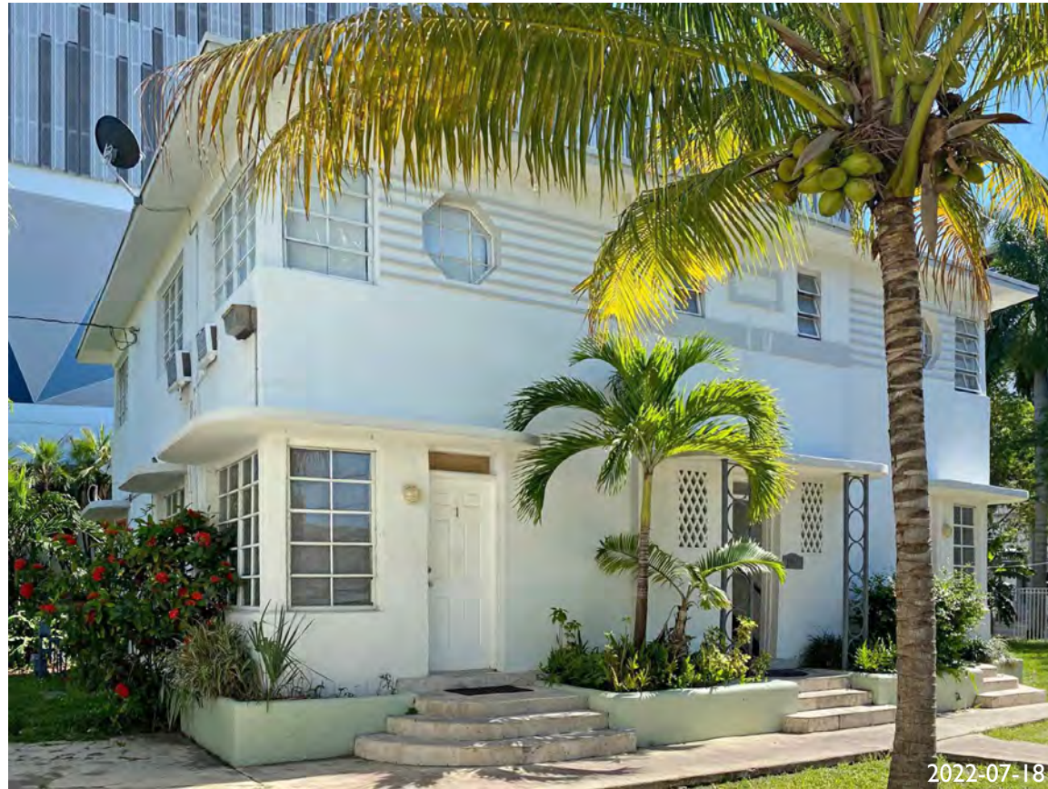
11. EXISTING SOUTH BUILDING
