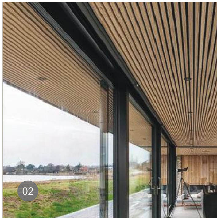
02 SOLID WOOD EXTERIOR CEILING SYSTEM @ BALCONIES & OVERHANGS
