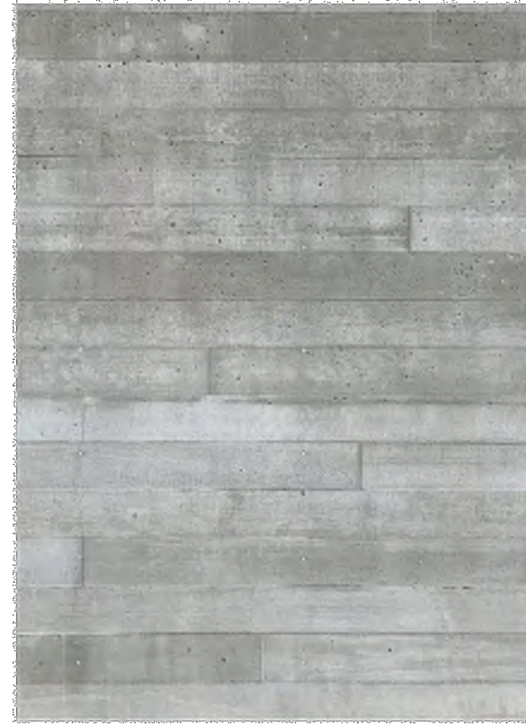
ARCHITECTURAL FEATURE WALL BOARD FORMED CONCRETE
