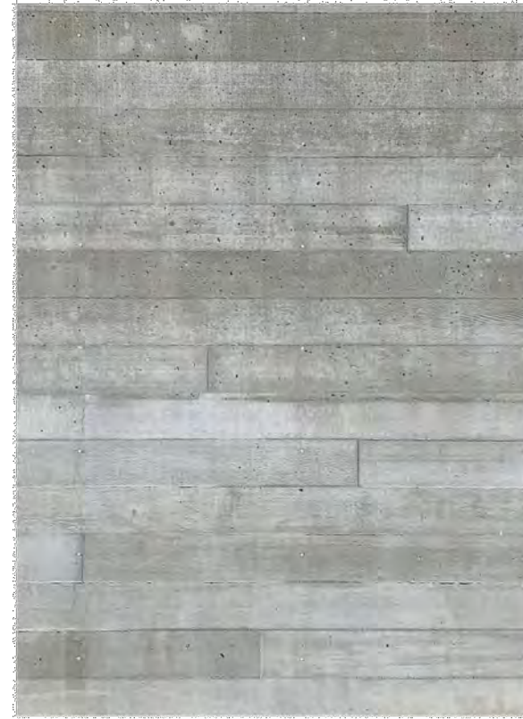
ARCHITECTURAL FEATURE WALL BOARD FORMED CONCRETE
