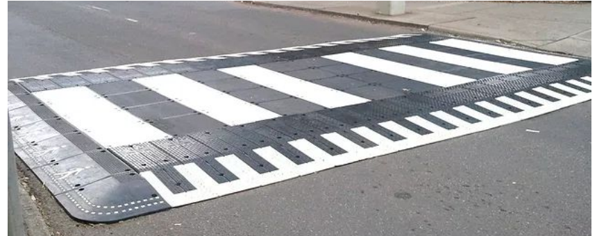
Temporary Raised Crosswalk/Intersection
