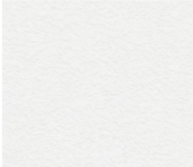
MICRO CEMENT WHITE FINISH ON MASONRY
