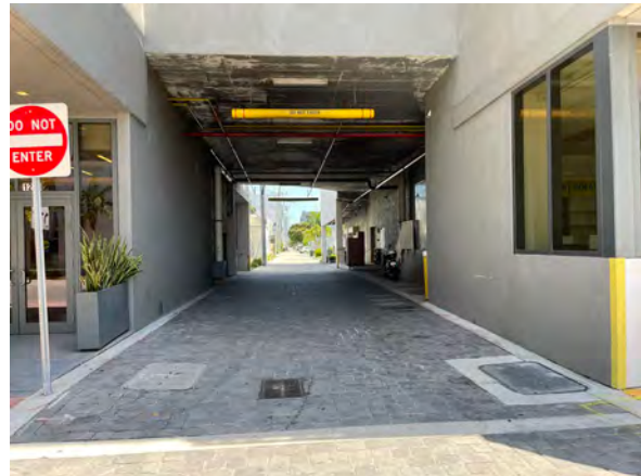
Photo 2 – Alton Court Looking South
