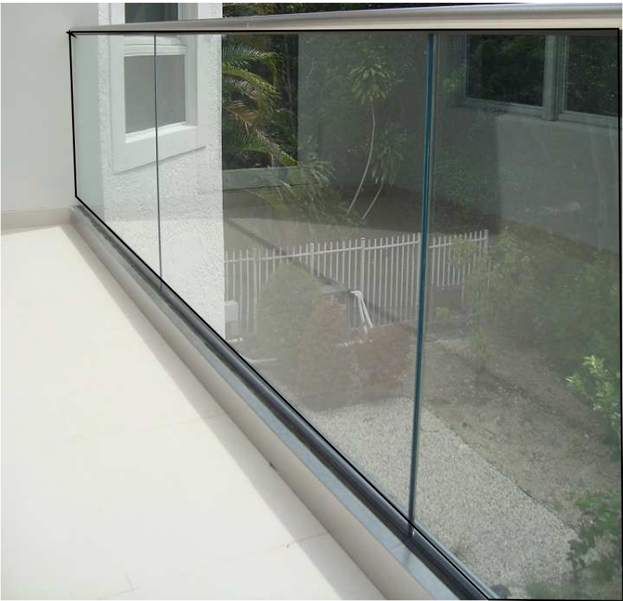
GREY TINTED GLASS WITH METAL RAILING
