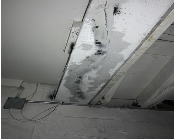
Excessive Beam Cracking and Spalling
