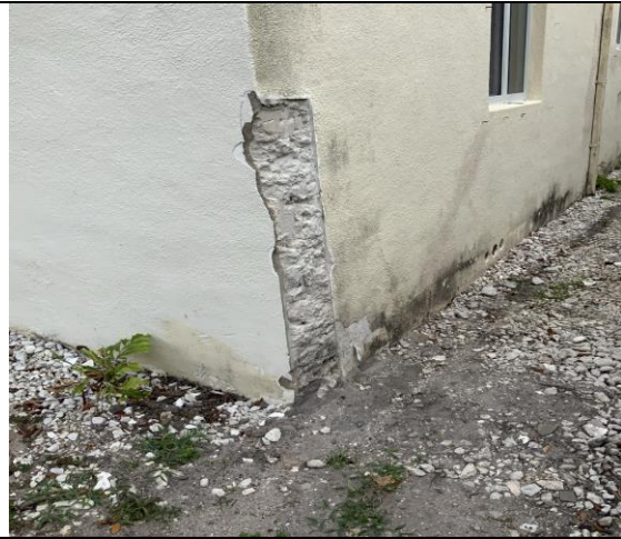
Delaminated Stucco and Spalling Concrete
