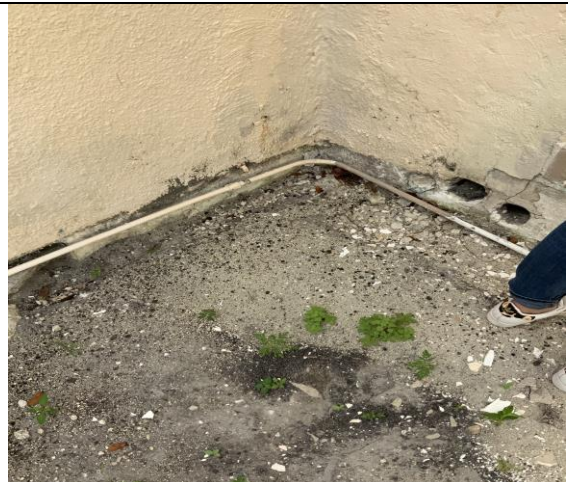
Deterioration at the Base of the Wall
