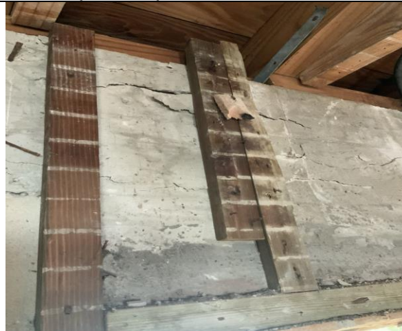
Spalling Concrete at top & bottom of Wall
