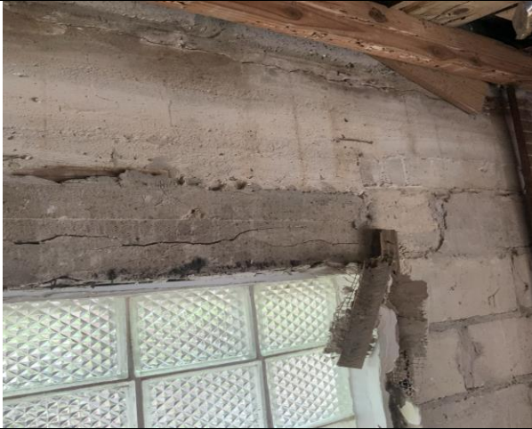
Cold Joints and excessive cracking and spalling
