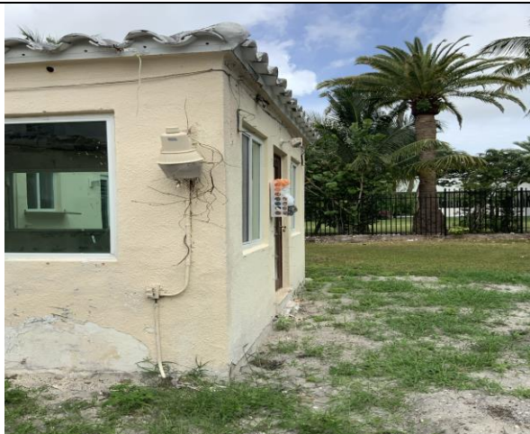
Delaminated Stucco and loose Electrical Connections
