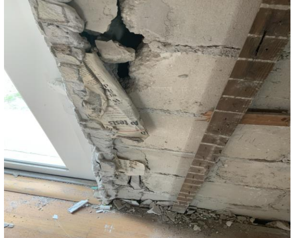
Interior Spalled Door Jam
