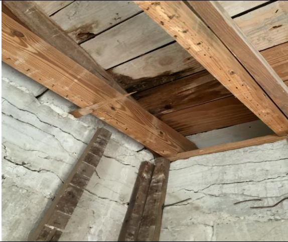
Internal Severe Wall Cracking
