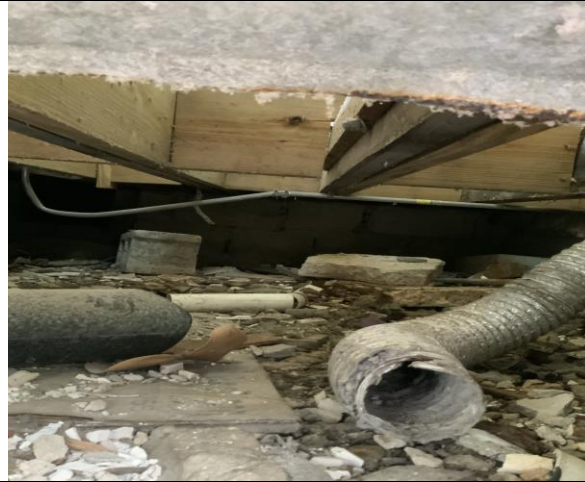
Crawl Space in poor condition due to Termites
