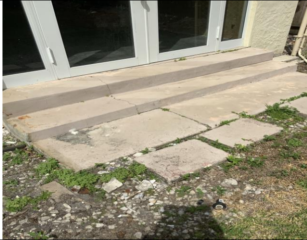
Cracks and loose Entrance Steps
