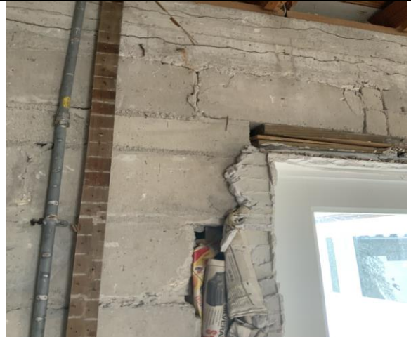
Severe Cracking, Concrete Spalling and wooden planks in the wrong place
