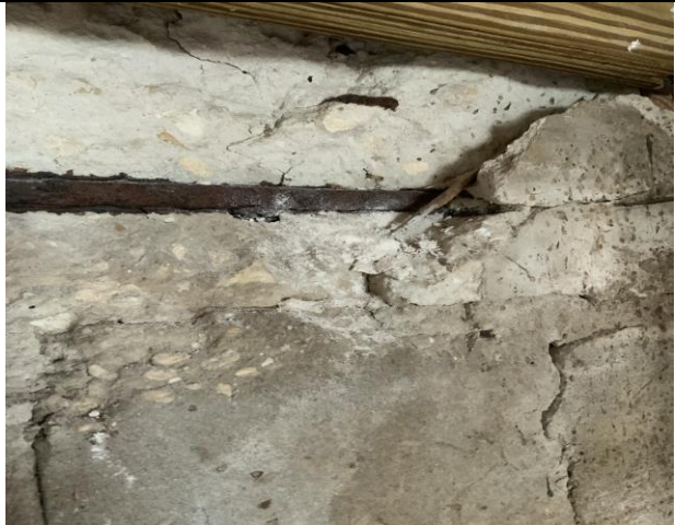
Excessive Concrete Spalling at the Beam
