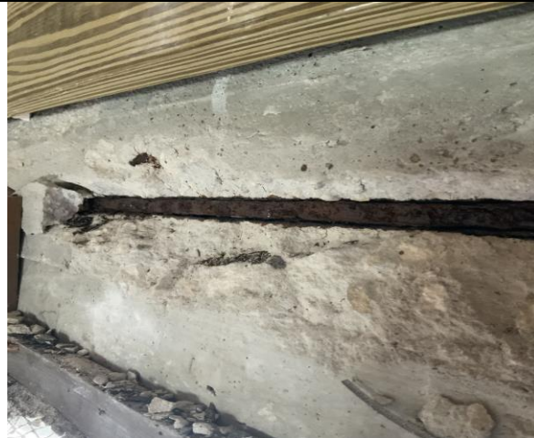
Excessive Concrete Spalling and Rebar Rusting
