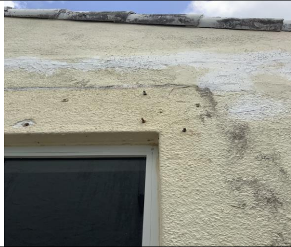
Delaminated Stucco on External Walls
