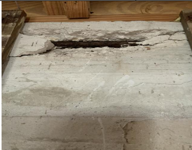
Spalling Concrete @ the Beam
