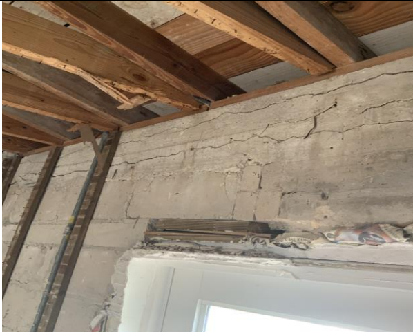
Excessive concrete spalling and wood Joist damage
