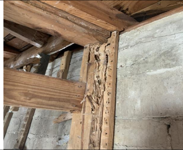
Severe Termite Attack at the wooden Joists
