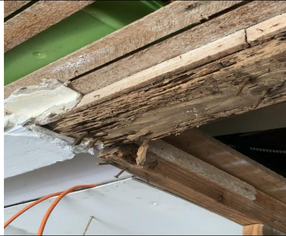
Wood Joists attacked by Termites
