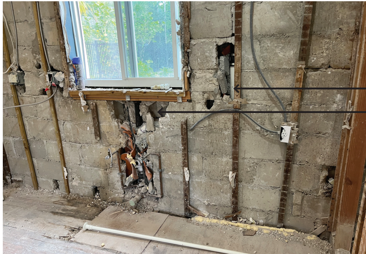
OPENINGS IMPROPERLY FILLED
