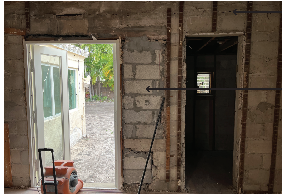
EXTENSIVE SPALLING AT UPPER AND LOWER REBAR OF TIE BEAM. REBAR FULLY EXPOSED AND DETERIORATED
