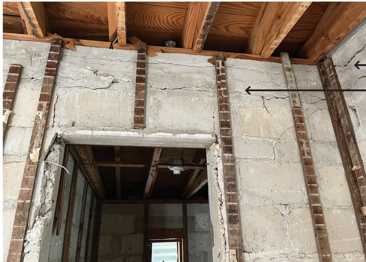
EXTENSIVE SPALLING AT UPPER AND LOWER REBAR OF TIE BEAM
