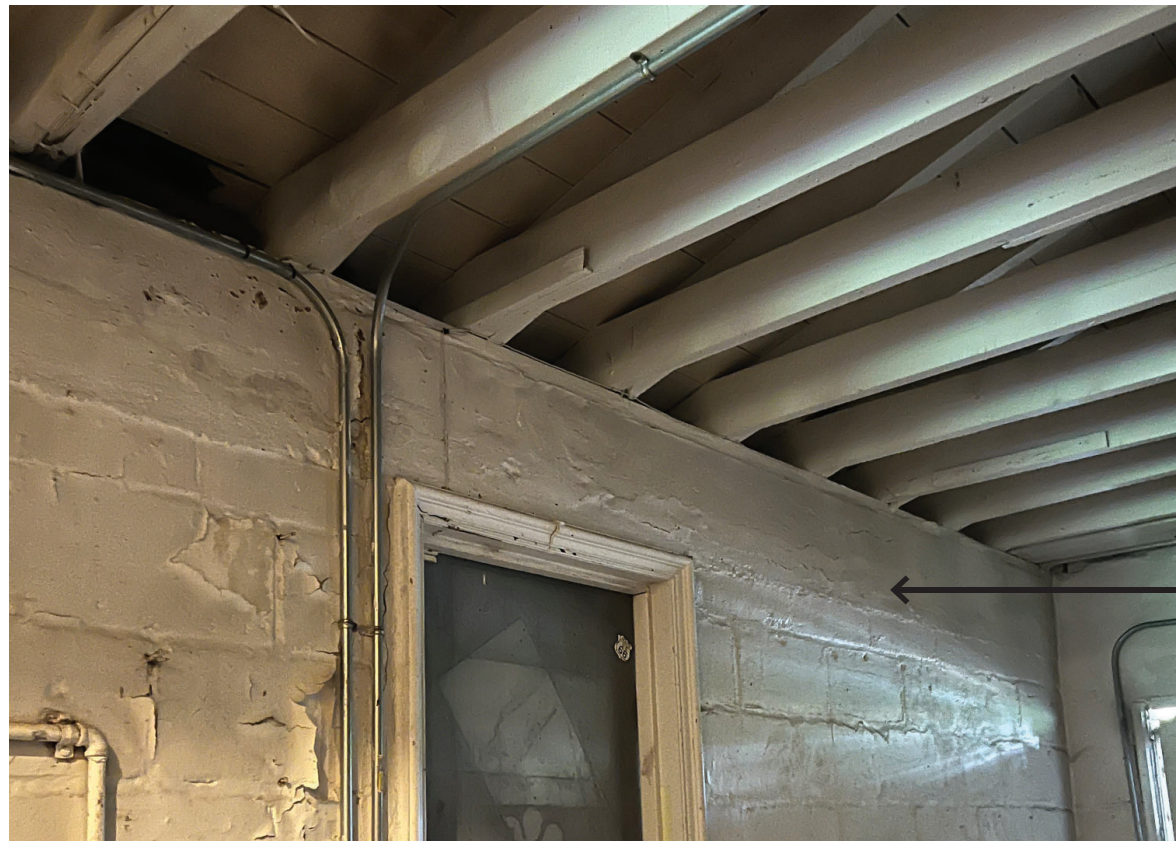
EVIDENCE OF SPALLING
