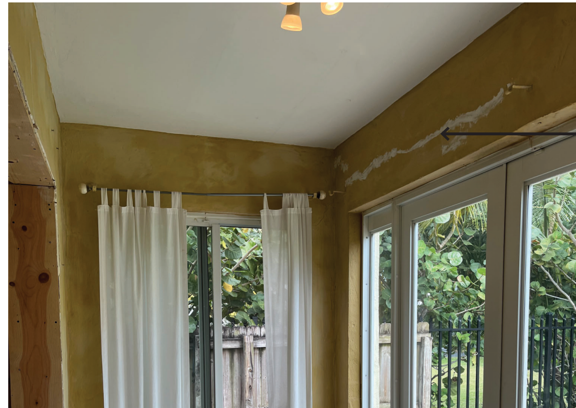
EXTENSIVE SPALLING AT UPPER AND LOWER REBAR OF TIE BEAM
