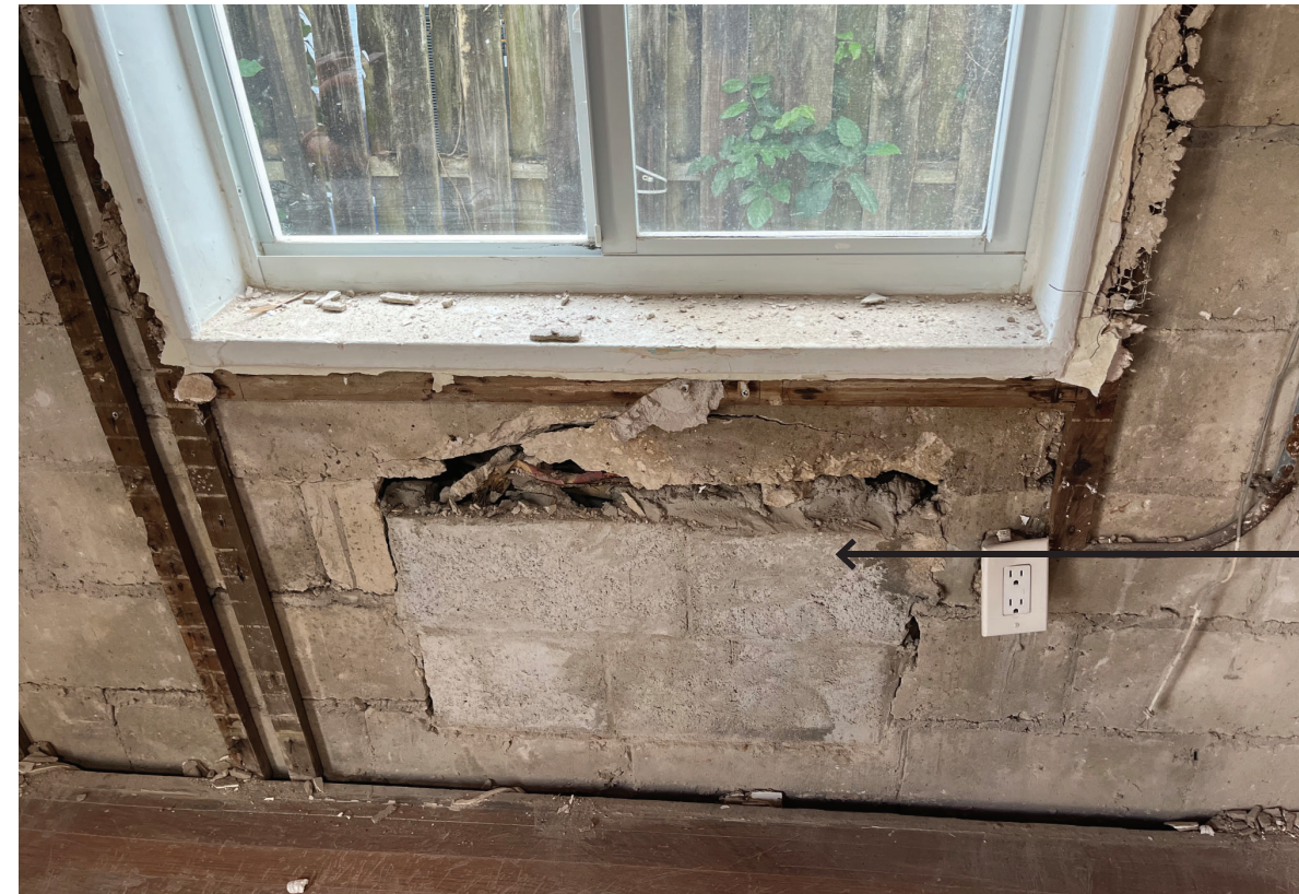
OPENINGS IMPROPERLY FILLED
