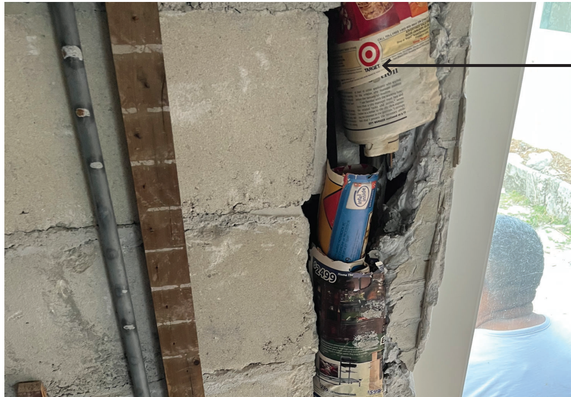
DOORS IMPROPERLY INSTALLED, NO TIE COLUMNS, NO BLOCK
