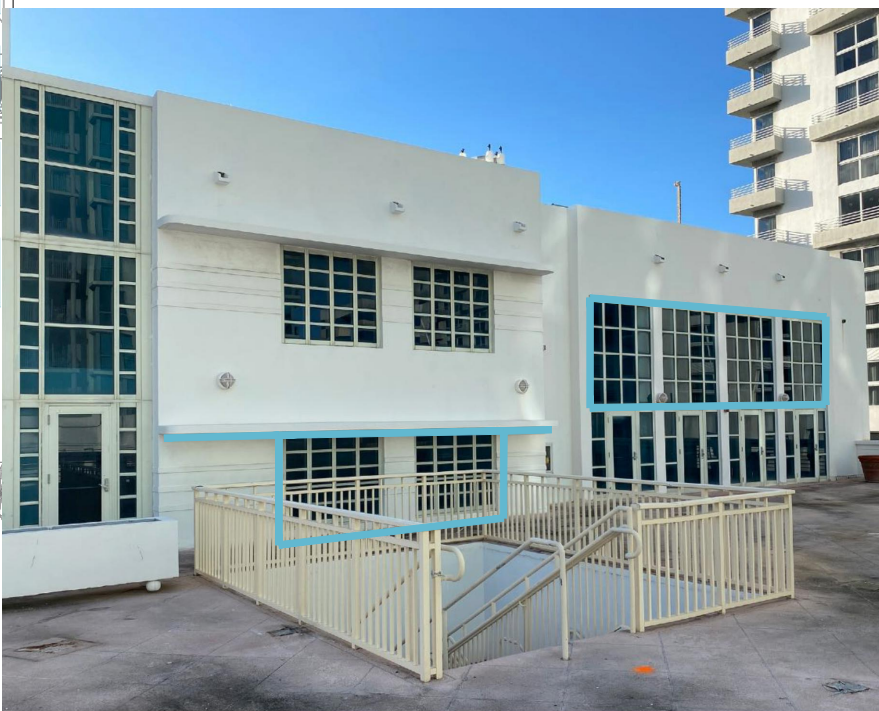
PHOTOS OF LEVEL 3 TERRACE EXISTING CONDITIONS
