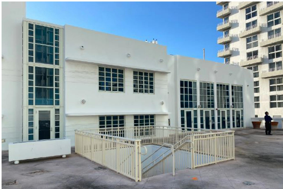
PHOTOS OF LEVEL 3 TERRACE EXISTING CONDITIONS
