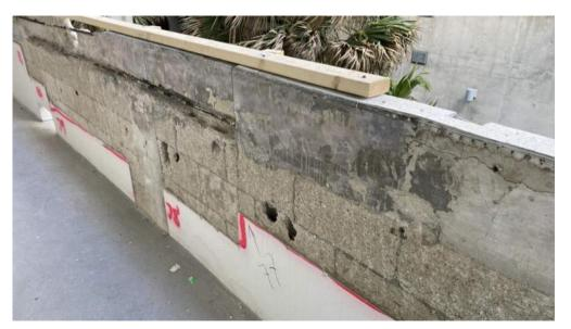
Distressed concrete and exposed / corroded reinforcement
