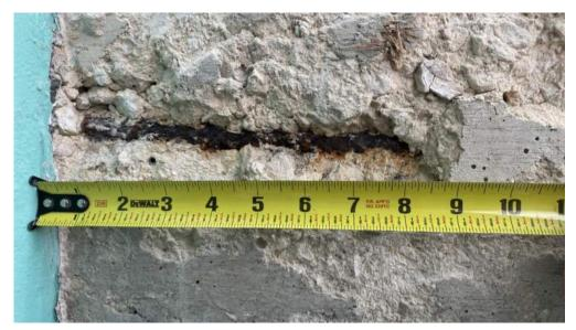
Distressed and exposed reinforcement
