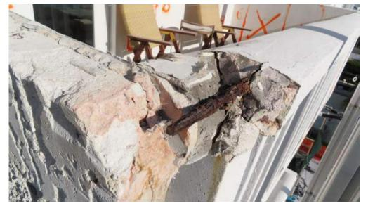
Discontinuous and exposed reinforcement
