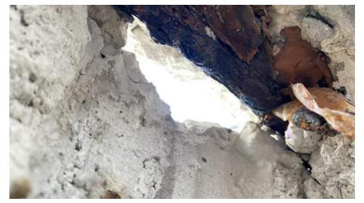
Unbonded concrete and corroded reinforcement
