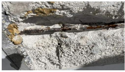
Unbonded concrete and corroded reinforcement
