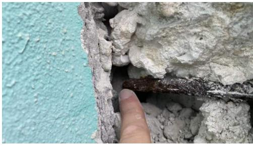
Discontinuous and exposed reinforcement
