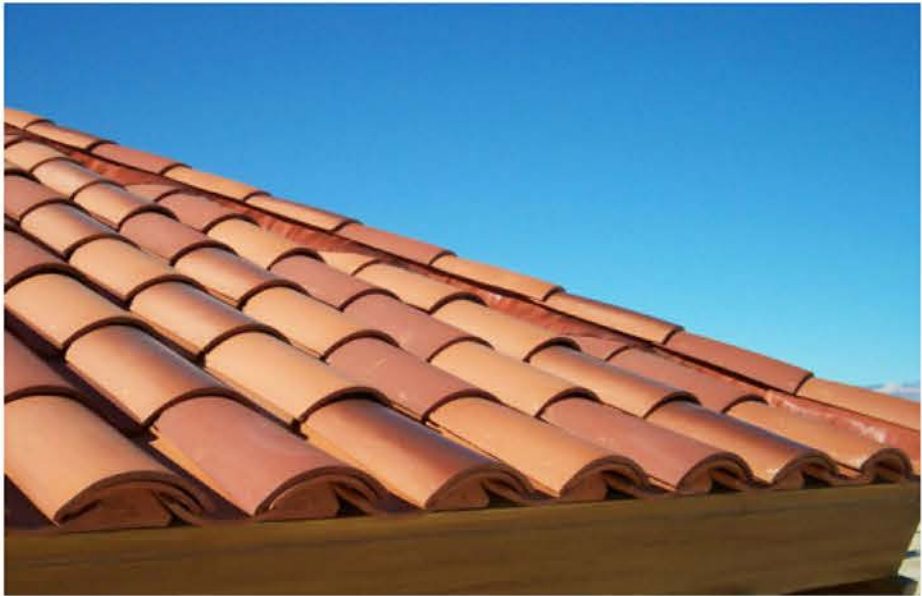
TERRACOTTA CLAY TILE ROOF ON THE TOWER
