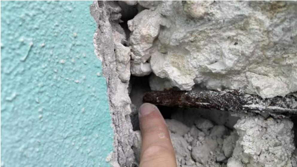
Discontinuous and exposed reinforcement
