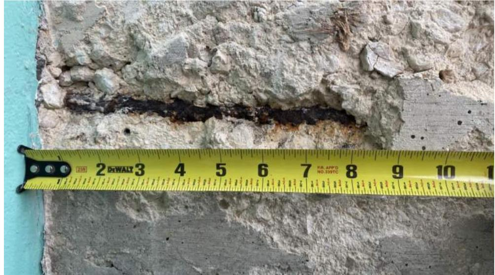
Distressed and exposed reinforcement
