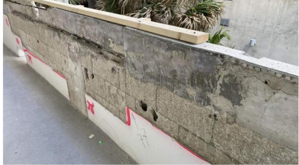
Distressed concrete and exposed / corroded reinforcement
