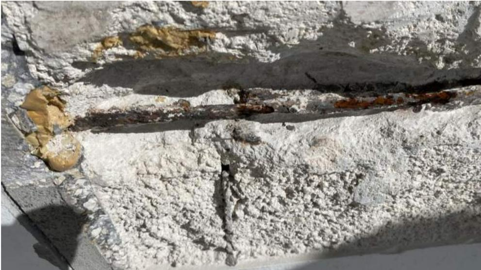
Unbonded concrete and corroded reinforcement
