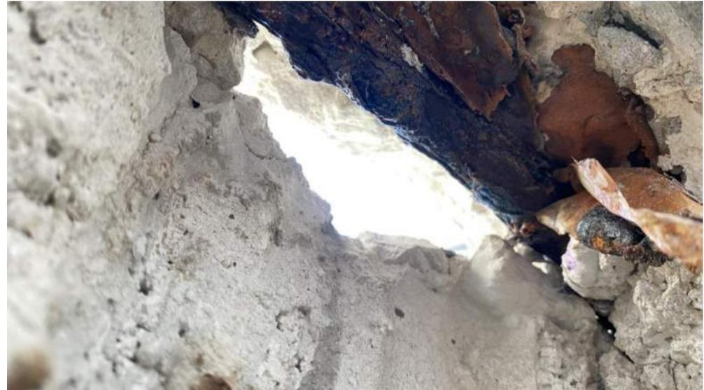
Unbonded concrete and corroded reinforcement
