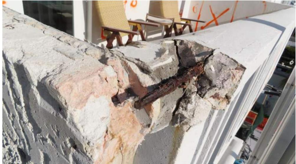
Discontinuous and exposed reinforcement
