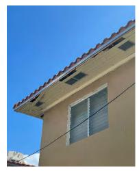
Fig. 35. Detail Flat tiles roof slighly overhangs.
