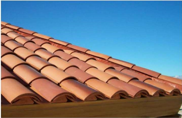
TERRACOTTA CLAY TILE ROOF ON THE TOWER
