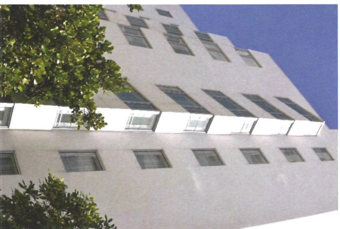
Fig. 181. Detail of angled windows at north elevation, July 2021.
