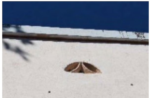
Figure 46. Detail of scupper at south elevation of Building A, January 2022.
