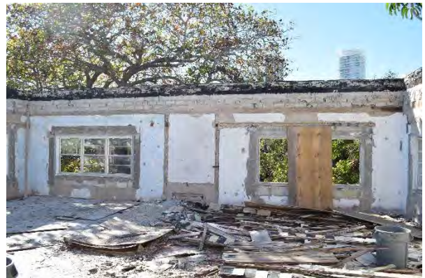
Figure 42. Missing roof and gutted condition at second level of Building A, January 2022.
