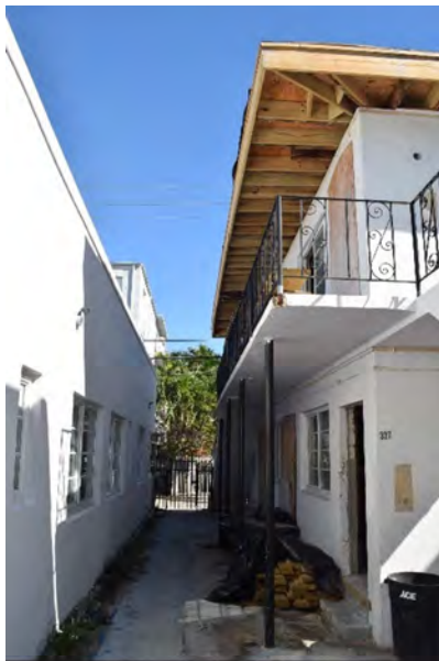
Figure 82. Metal posts supporting elevated walkway at north elevation of Building D, January 2022.
