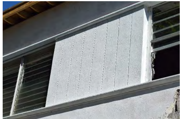
Figure 63. Incised stucco between upper level windows at west elevation of Building C, January 2022.
