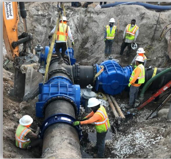
Pump Station No. 28 Valve Replacement
