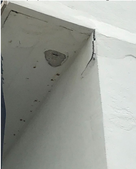
Lack of proper column reinforcing.
