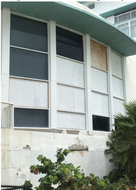
Reinforcing and extensive damage to eyebrows
