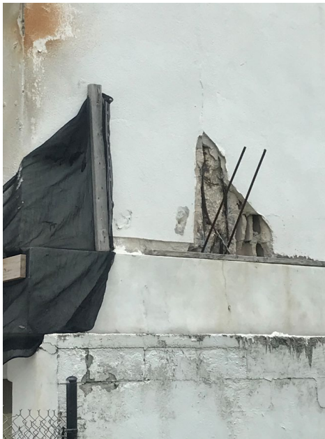
Lack of proper column reinforcing.
