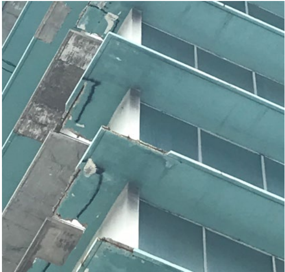
Reinforcing and extensive damage to eyebrows
