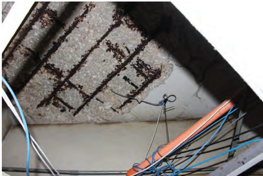
Image 55: Typical condition of corroded slab rebar apparent above Ground, Lobby, and Upper Levels.
