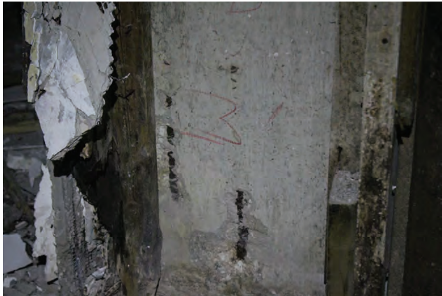
Image 67: Typical condition of column reinforcement with less than 1" of clear cover on Ground Level below South Ballroom, within the interior of the building.
