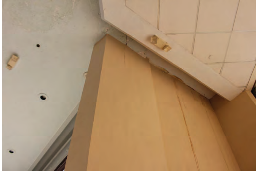
Image 64: Typical concealed corrosion damage with visible distress within Lobby along perimeter walls.
