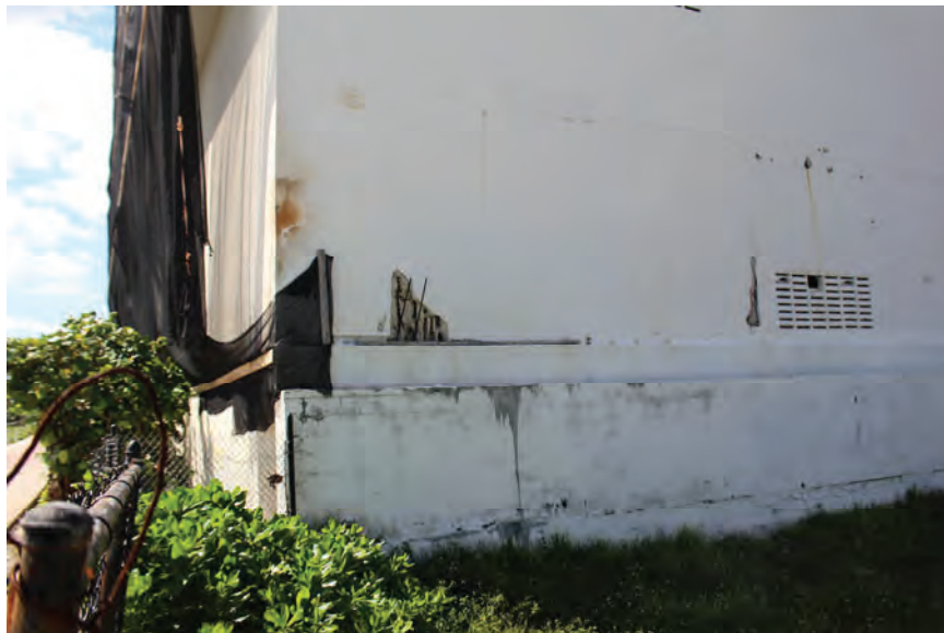
Image 25: Unfinished and open repair areas of structural columns along the Hotel's north face.
