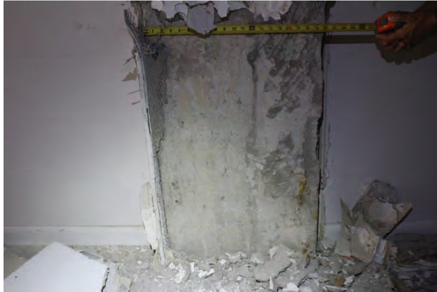
Image 88: Typical vertical joint in column.
