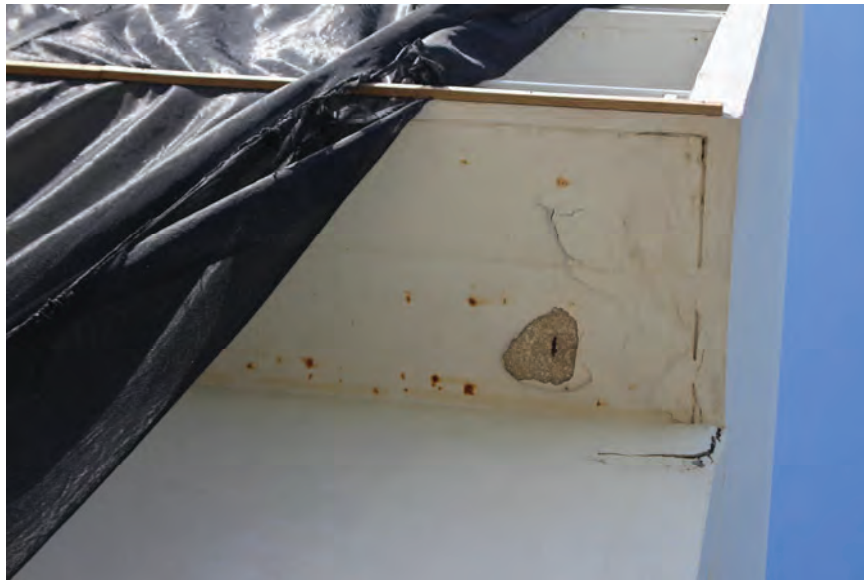
Image 29: Typical Hotel east face balcony and column corrosion.
