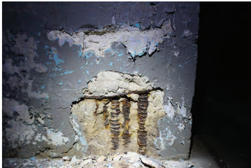
Image 77: Condition of Ground Level Hotel frame column which featured flaked paint and powder-like concrete. While sounding the column with a hammer, a concrete spall detached and revealed severe corrosion, closely spaced rebar, and offset rebar cage (inadequate clear cover). (Column Label 12)
