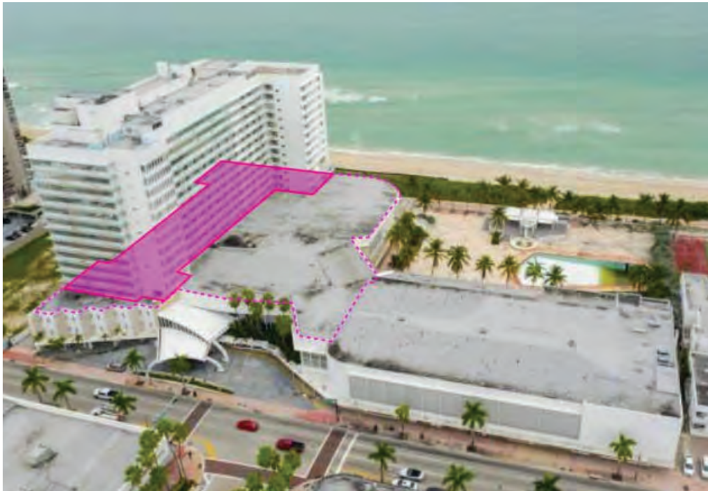
Image 17: Location of the Transfer Slab at 4 th Elevated Level below Hotel Portion of Structure, Continuous with Low Roof Structure.
