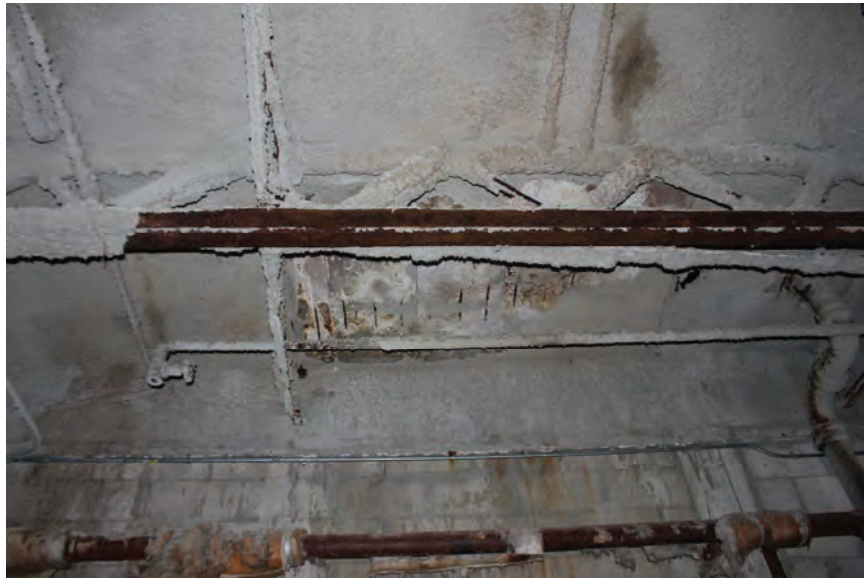
Image 57: Typical condition of corroded plank slab concealed by fireproofing/insulation.
