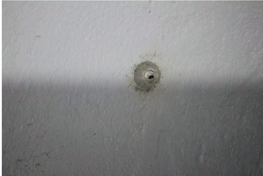
Image 101: Typical condition of a “blow out” location of a Windsor Probe which exposed interior voids within the concrete columns.
