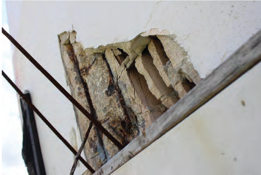
Image 26: Unfinished and open repair area for structural column at east end of the Hotel's north face.
