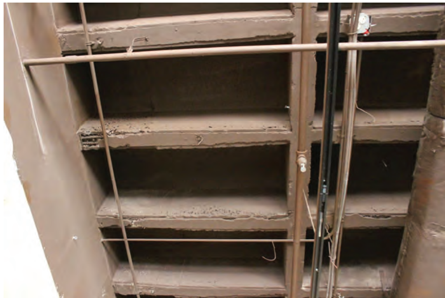
Image 85: Typical condition of sporadic and widespread nature of honeycombed concrete. Note exposed reinforcement.
