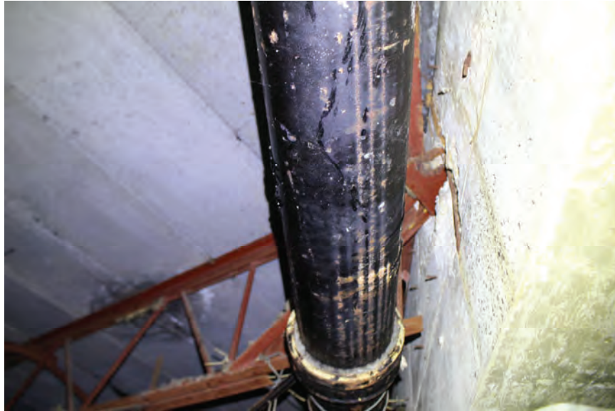
Image 86: Typical honeycomb at steel truss connection to reinforced concrete structural frame. Primarily located above Lobby and Ballrooms. Note corrosion of exposed reinforcement.
