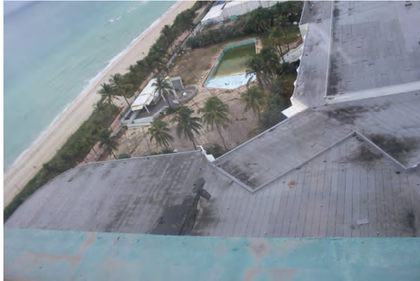
Image 94: Typical condition of low roof and parapets.
