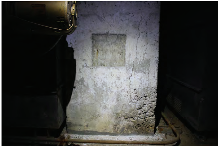
Image 75: Typical condition of Ground Level Hotel frame column with substantial honeycomb. Note corrosion cracks.
