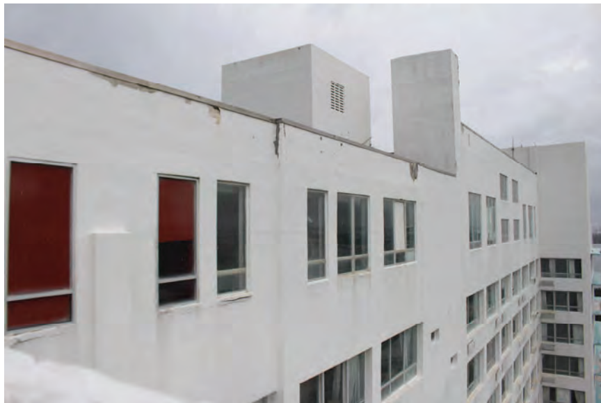
Image 23: View of the apparent beam corrosion and prior repairs on north face of hotel.
