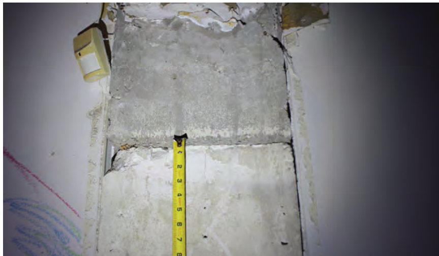
Image 87: Typical horizontal joint within frame column in conjunction with poor mix and concrete quality. Note that the lower portion of the column was a powder-like consistency, able to be removed in large pieces by hand, and the upper portion of the column was a grainy consistency which was able to be scraped away by hand. (Label 3)
