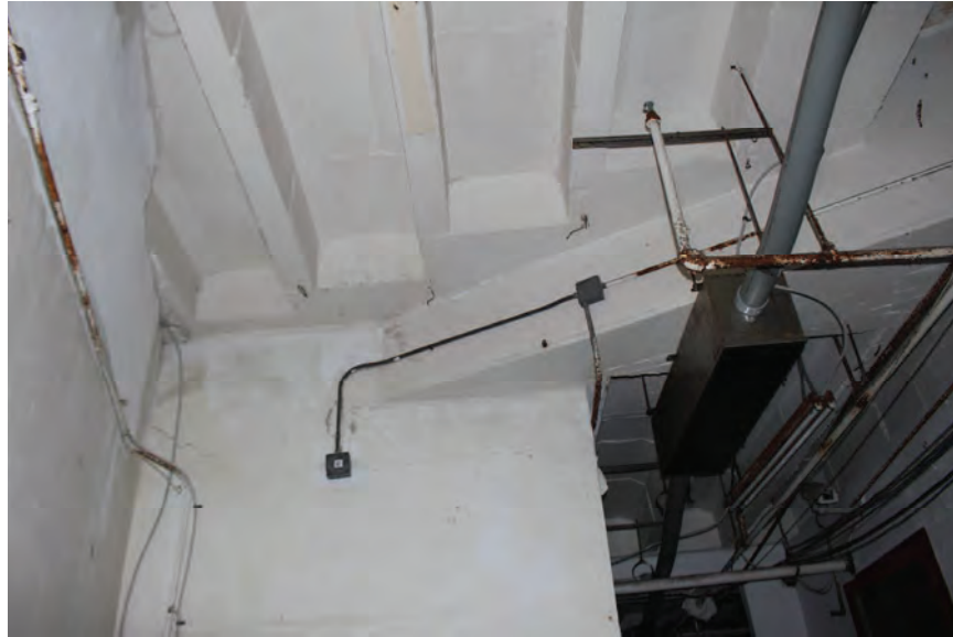
Image 90: Structural crack which transmits through walls, beams, and slabs along the interface between the hotel portion and lobby portion of the building, viewed within the Ground Level. Note that there was no isolation joint between the hotel and lobby portions of the building.
