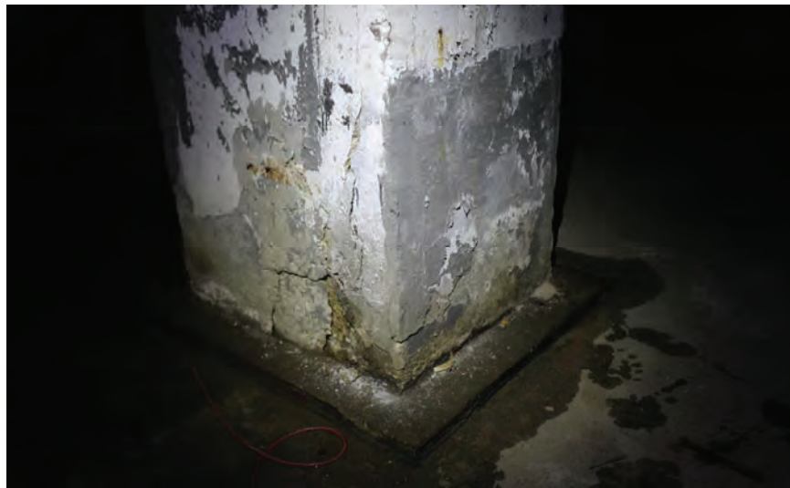
Image 73: Typical condition of Ground Level Hotel frame column with previous patch repairs.
