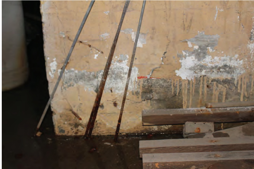
Image 78: Condition of the east end of the main lobby elevator shaft, including a Ground Level hotel frame column. Note the corrosion. (Column label 14)
