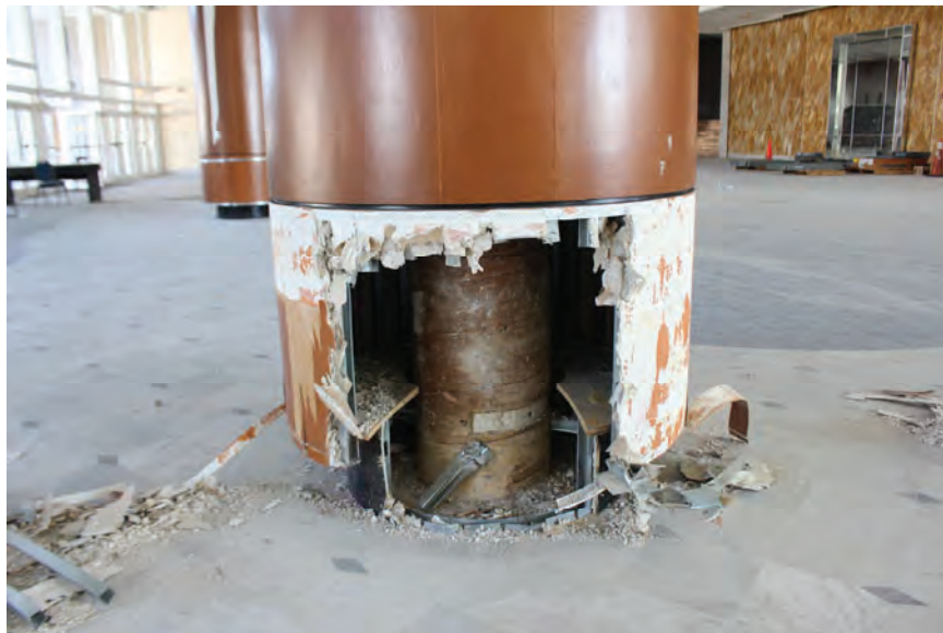
Image 51: Typical sonotube column within Lobby. Note that the column's sonotube paper was encasing the column.
