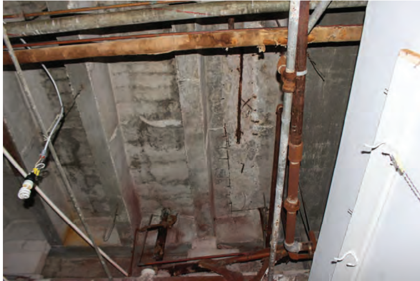
Image 54: Typical condition of slab system from Ground Level, below Hotel. Note corrosion as well as honeycombed concrete.
