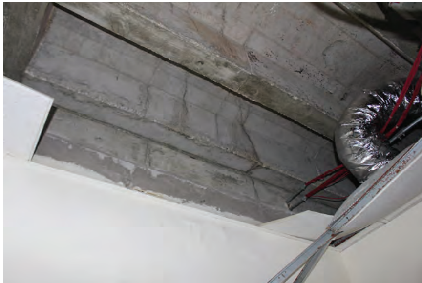
Image 89: Typical condition of slab system cracks which propagated through the joists near hotel perimeter walls in upper floors.
