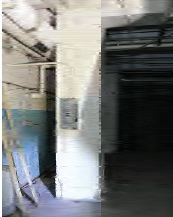
Image 52: Typical condition of Ground Level column, below Hotel, within the interior of the building. Note corrosion as well as honeycombed concrete.
