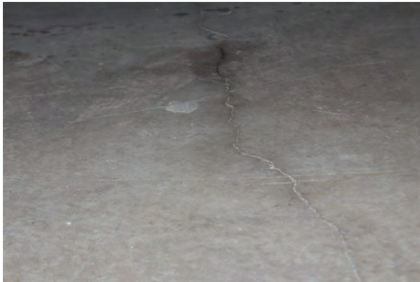
Image 65: Typical crack condition along top of South Ballroom floor slab, along the supporting Ground Level office walls, which was an indication of slab deflection between supports.
