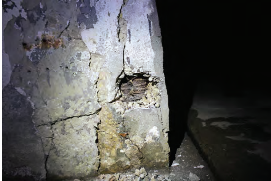
Image 74: Typical condition of Ground Level Hotel frame column closely spaced reinforcement as well as inadequate concrete mix. Note the loose aggregate and little to no cement paste. (Column Label 10)
