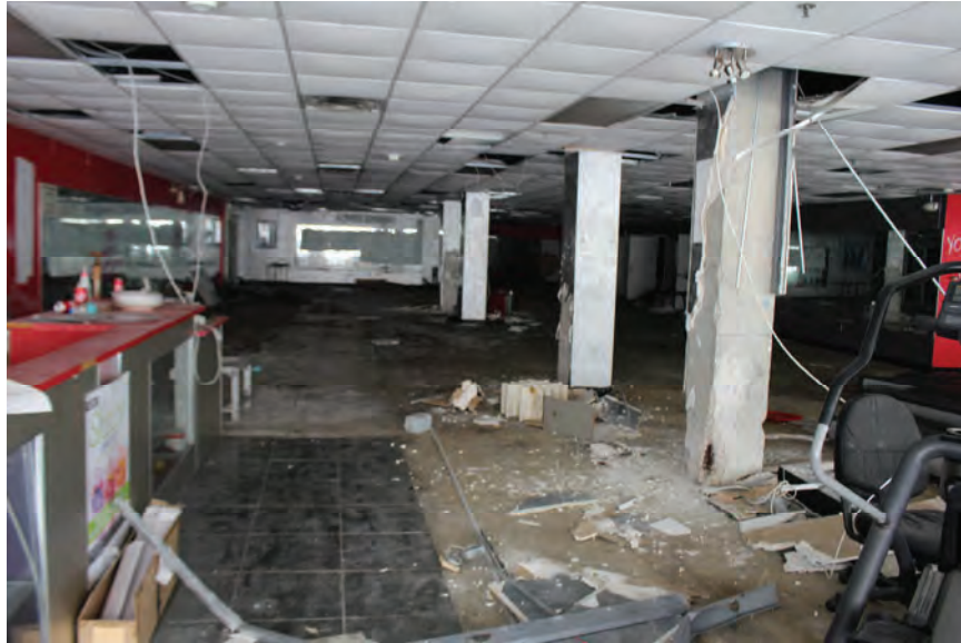
Image 68: Corrosion of interior Ground Level columns, located at south end of building.
