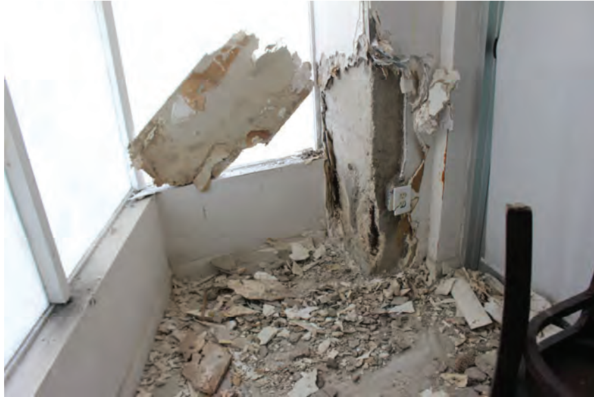
Image 70: Corrosion of perimeter Ground Level columns, located along west face of south end of building.
