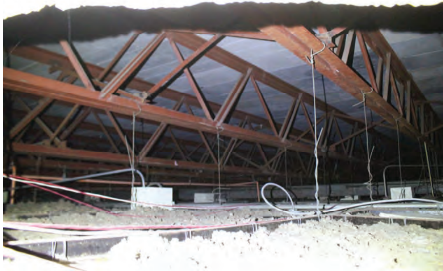
Image 50: Typical steel truss and concrete plank roof system above the Lobby and Ballrooms (excluding south ballroom).
