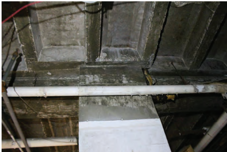
Image 81: Typical condition of congested beam-column Ground Level Hotel frame joint. Note honeycombed concrete. Note the size of the columns and beams (beam spans left to right above column in image)
