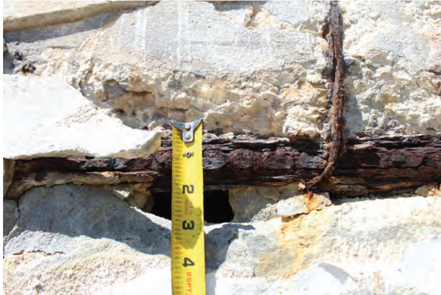
Image 34: View of the loss of steel cross-section within support wall below east ballroom.
