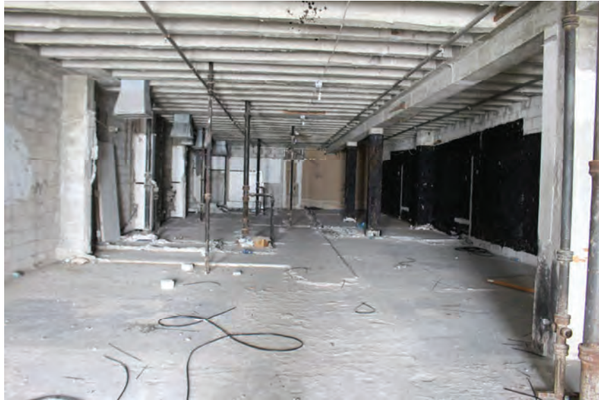
Image 46: Typical condition of concrete frame system at roof level of hotel. Note the size of the beams and columns.
