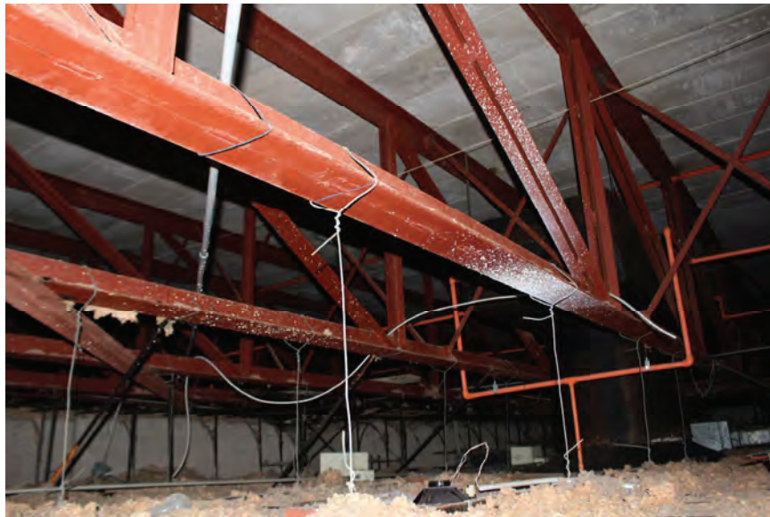
Image 49: Typical steel truss and concrete plank system above the South Ballroom.
