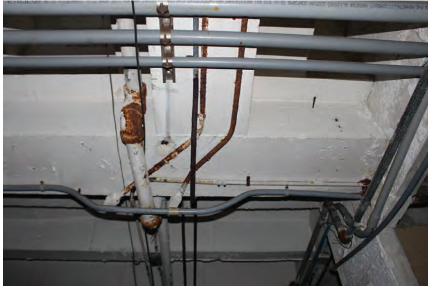
Image 32: View of the condition of a corroded and cracked beam (shear and flexural cracks), located below the exterior radius wall of the east ballroom. (Beam Label 6)
