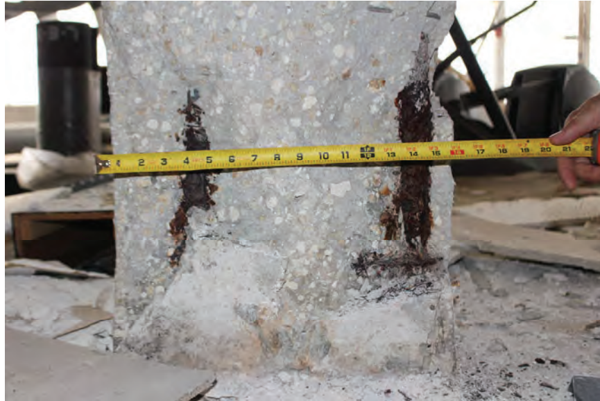
Image 84: Typical condition of offset rebar within column cross-section, affecting clear cover and depth of reinforcement. Note advanced corrosion particular to this column, Label 1.
