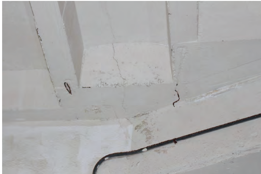
Image 91: Close up view of structural crack in previous image. Note the continuation of the crack through several elements. Note the honeycomb in the slab.
