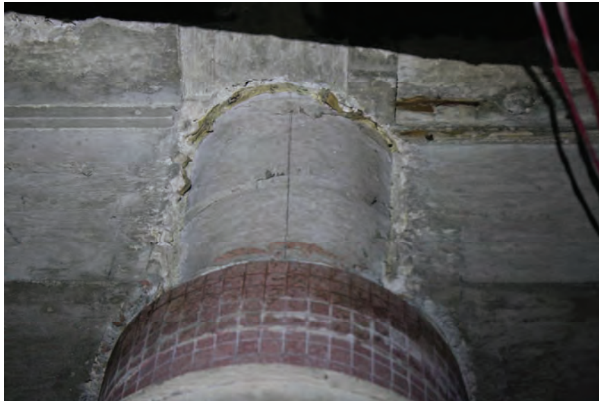
Image 83: Typical condition of sonotube paper within the beam-column joint. Note honeycombed concrete.
