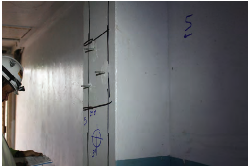
Image 99: Typical condition of the 3 probes installed for the Windsor Probe Test. (Column Label 5)
