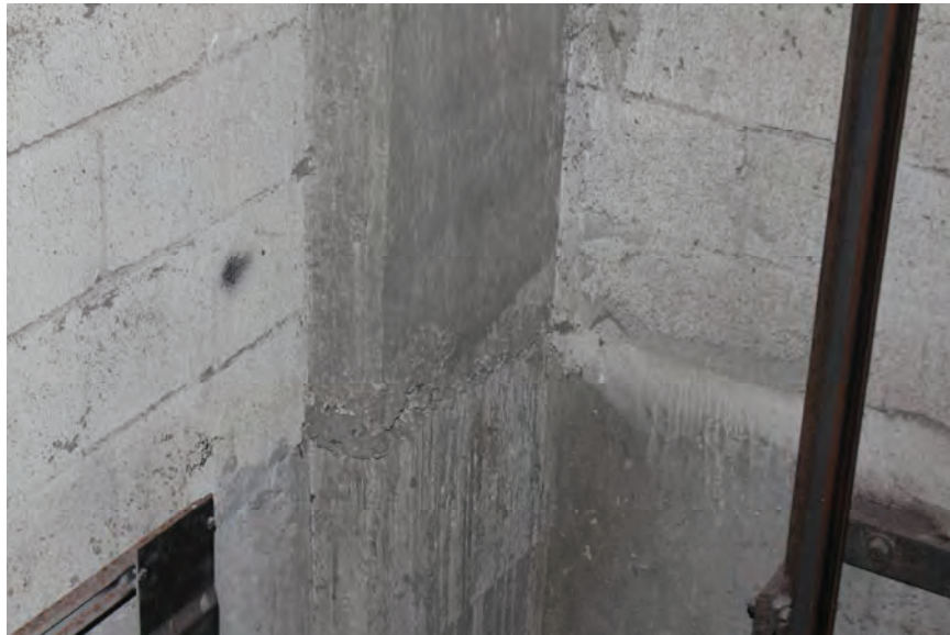
Image 79: Typical condition of the joints within the main lobby elevator shaft's rigid frame system. Note the honeycomb.
