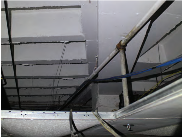
Image 80: Typical condition of congested beam-column frame joint. Note honeycombed concrete and poor horizontal joint within column.
