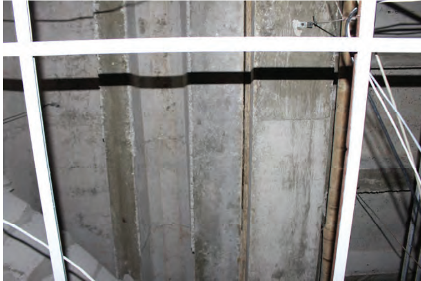
Image 44: View of the isolation joint between the north and south portions of the structure, shown in Image 15.
