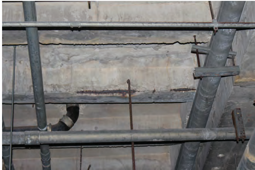
Image 60: Typical condition of joist corrosion.
