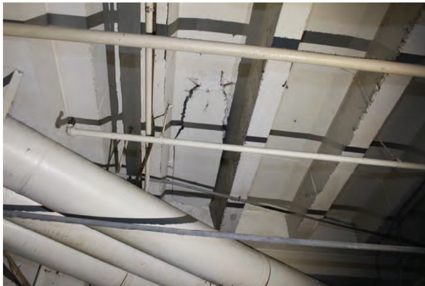
Image 53: Typical condition of slab system from Ground Level, below Hotel. Note corrosion as well as honeycombed concrete.
