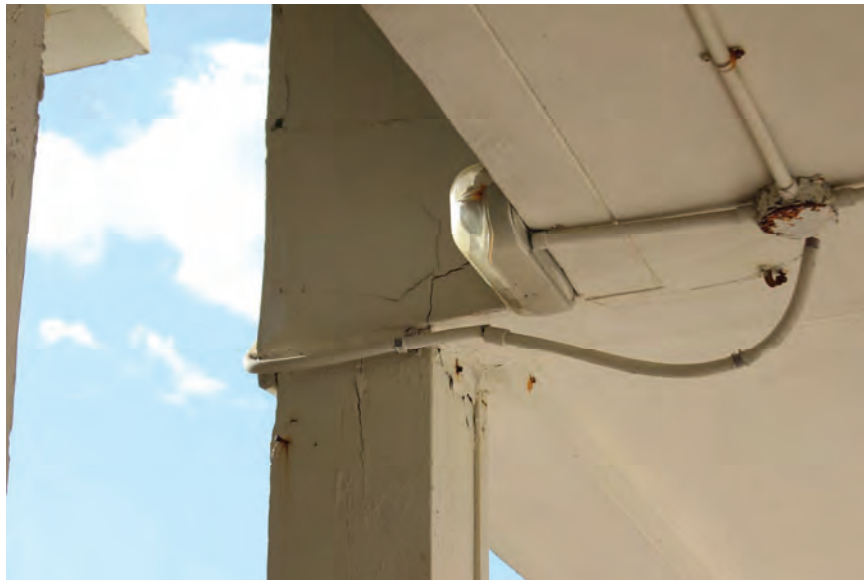
Image 71: Typical exterior corrosion damage along south portion of building.
