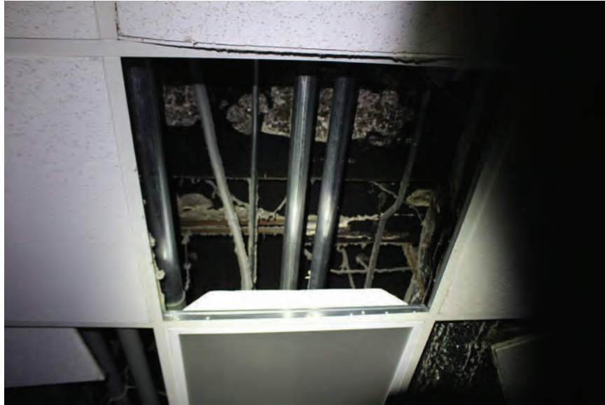
Image 58: Typical condition of 3 rd Floor Level (transfer slab). Note spalled, cracked, and deteriorated concrete.
