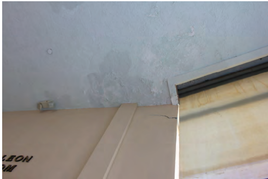
Image 63: Typical concealed corrosion damage with visible distress within Lobby along perimeter walls.
