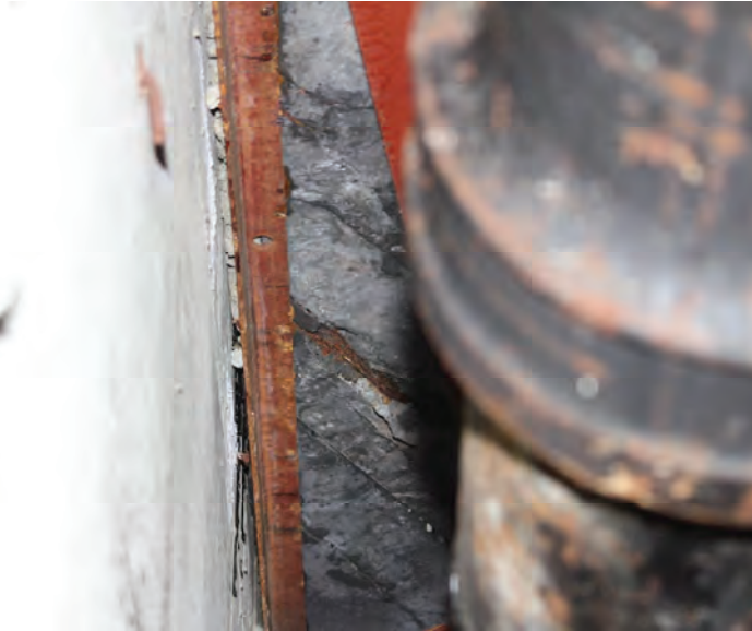
Image 56: Typical condition of corroded plank slab system above the steel truss framed roofs above the Lobby and Ballrooms
