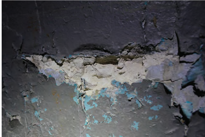
Image 76: Condition of Ground Level Hotel frame column which featured flaked paint. While sounding the column with a hammer, we encountered powder-like concrete at an apparent horizontal joint. (Column Label 12)
