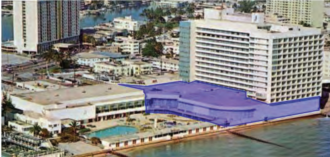
Image 16: Graphic Depiction of Continuous Structure with Hotel Portion (blue shaded area) based on Isolation Joint Location.
