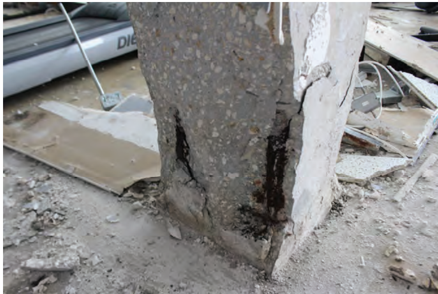
Image 69: Corrosion of interior Ground Level columns, located at south end of building.
