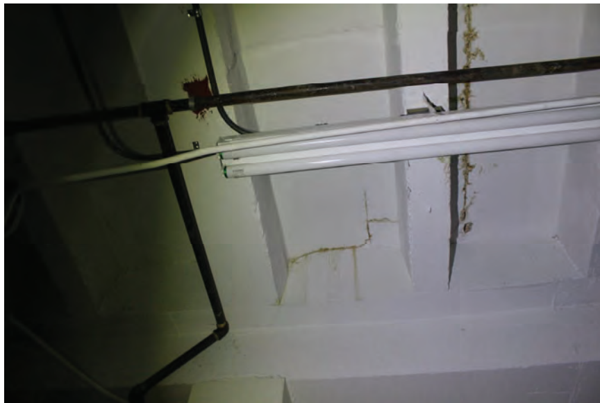
Image 47: Typical propagation of cracks off concrete frame system into adjacent slab (diaphragm) system. Photo shown below main roof level.
