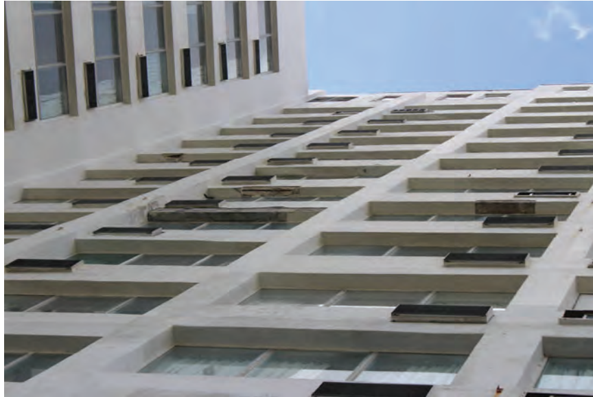
Image 22: View of the apparent beam corrosion and prior repairs along the Hotel windows on the north end of the building.
