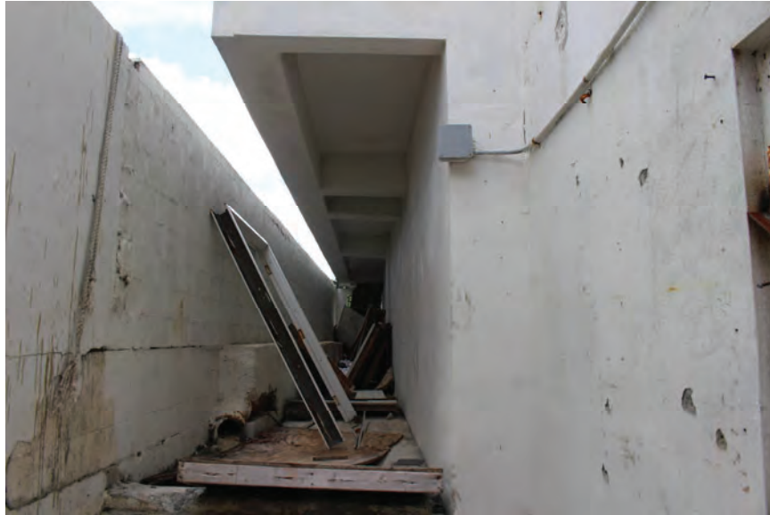
Image 24: Condition of the north end of the east wing of the Hotel. Note that the north wall of the Hotel's east wing was cantilevered off of the main structural frame at the Lobby Level.
